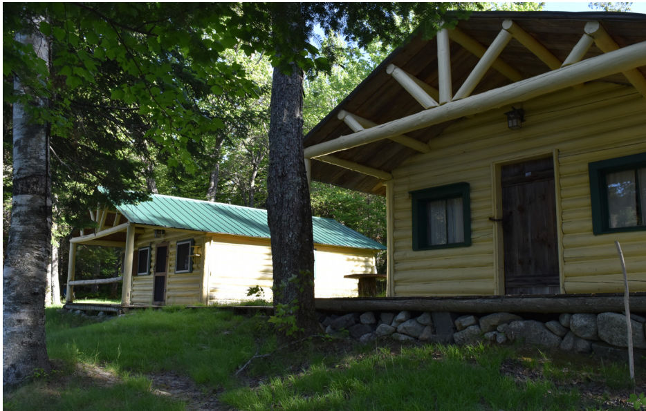
P2-13: Cabins at Spencer Rips on the Moose River.
