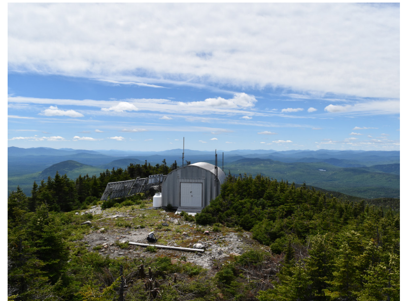
P2-33B: Building on Coburn Mountain.
