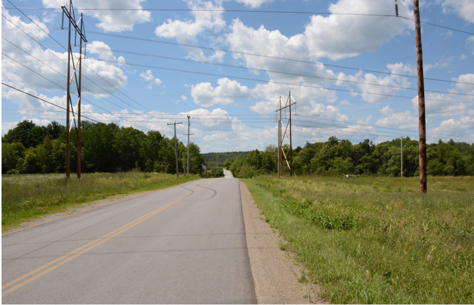
P12-4: View looking west on Maxcy's Mill Road in Windsor. The proposed 345 kV transmission line will be constructed in between the two existing transmission lines. No additional tree removal is required.
