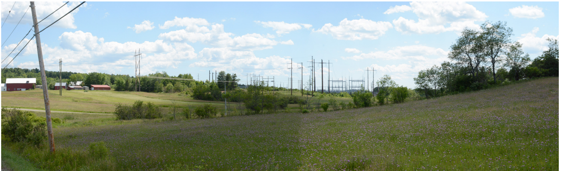
P12-3: Panoramic view looking from Coopers Mill Road in Windsor towards the Cooper's Mill Substation and existing transmission lines. Upgrades to the Substation for the Project will be located on the north side of the existing facility. The additional components will be minimally visible from Cooper's Mill Road.
