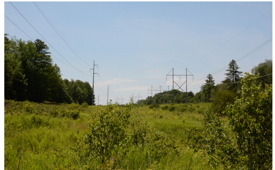
P12-15: View looking southwest from Cooper's Road. The proposed 345 kV transmission line will be constructed in between the two existing transmission lines. No additional tree removal is required.
