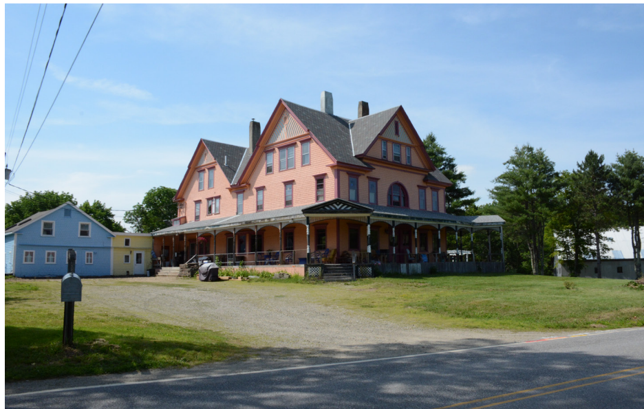
P12-28: National Register of Historic Places: Moody Mansion, Pittson. The Project will not be visible from this structure.
