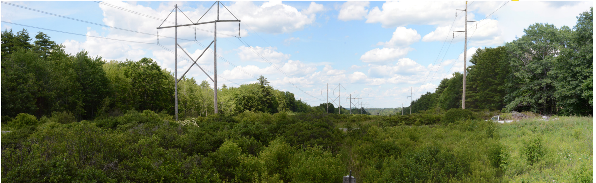
P12-7: Panoramic view from Route 32 in Windsor from north to northeast. The proposed 345 kV transmission line will be constructed in between the two existing transmission lines. No additional tree removal is required.
