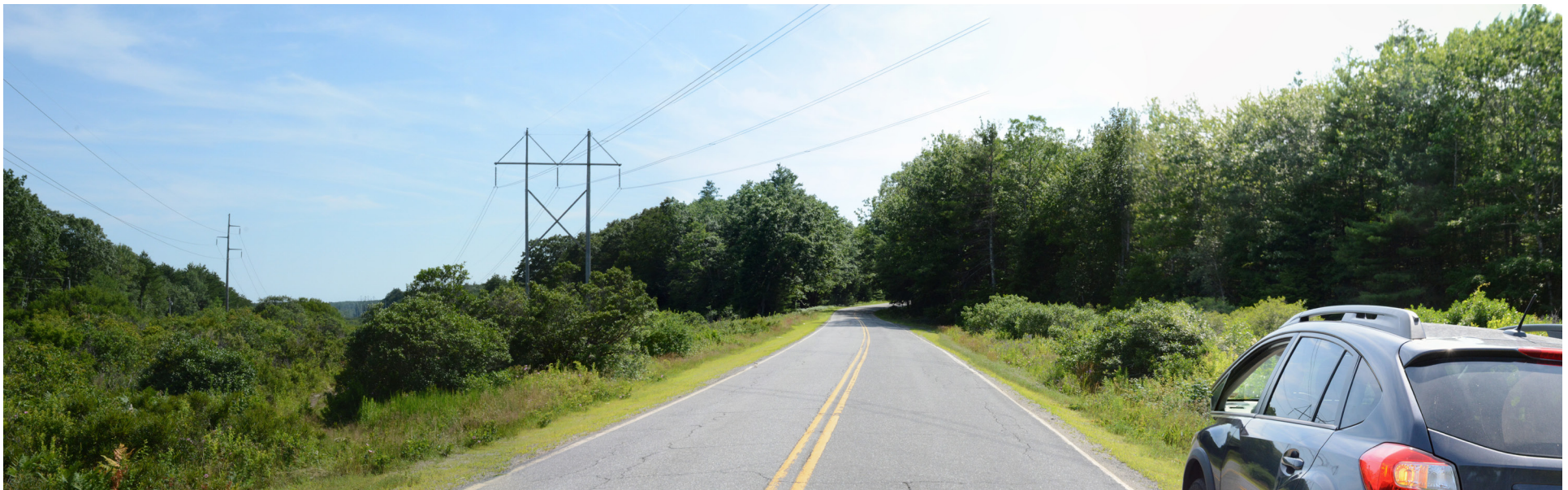
P12-32: Panoramic view from Wiscasset Road/ Route 218 existing transmission corridor looking southwest, Whitefield. The proposed 345 kV transmission line will be constructed in between the two existing transmission lines. No additional tree clearing will be required.
