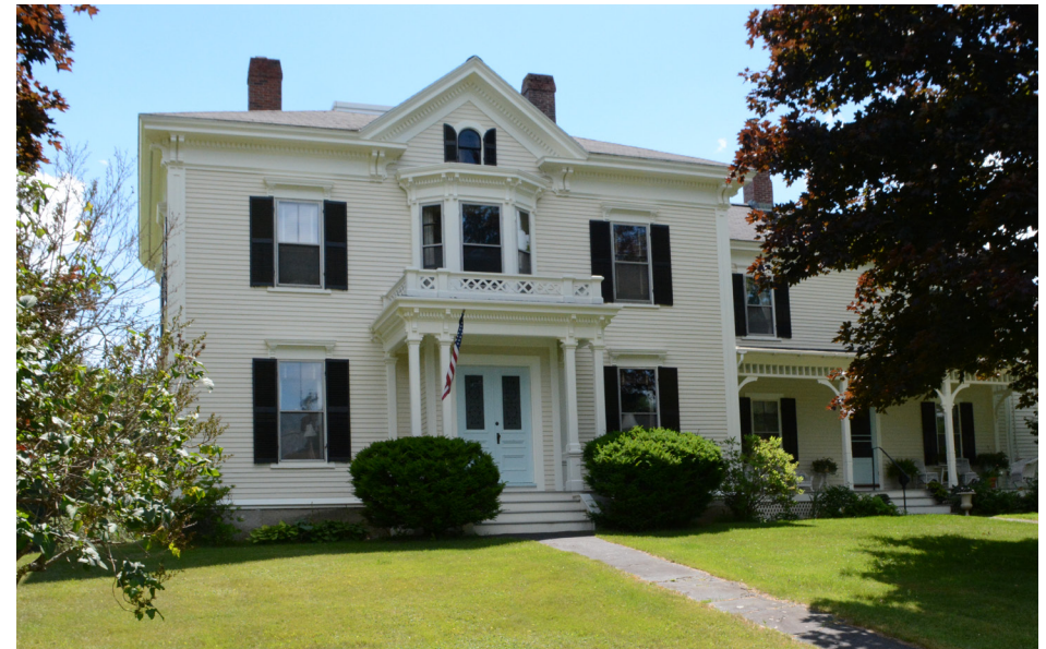
P11-32: Cross Point Road historic structure, Edgecomb. The Project will not be visible from this structure.
