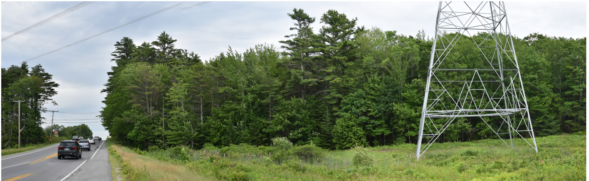
P11-35: Panoramic view from Route One in Wiscasset looking southwest toward the existing transmission line corridor crossing. The only visual change will be the addition of conductors to an existing lattice structure. See Photosimulation in Appendix D.
