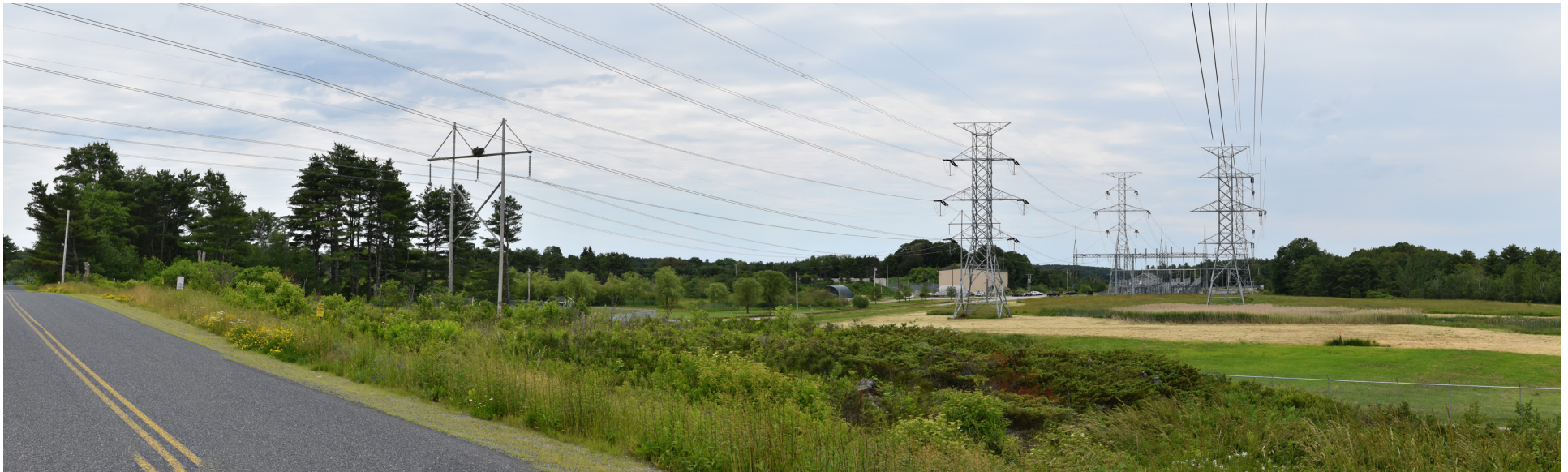
P11-41: Panoramic view looking south from Old Ferry Road at the Maine Yankee Substation in Wiscasset. The substation will be expanded on the western side within the existing fenced facility. The additional components will be similar in scale and color to the existing components. No additional lattice structures will be installed. The visual change will be minimally noticeable.
