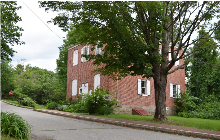
P11-22: National Register of Historic Places: Red Brick School House on Warren Street in Wiscasset. The Project will not be visible from this structure.
