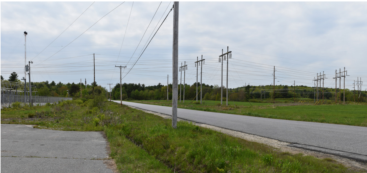
P10-9: Panoramic view looking southwest on Allen Road near the Surowiec Substation toward the existing transmission lines and location of Sections 62 & 64 Rebuild.
