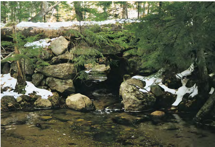
An old stone culvert still functioning.
