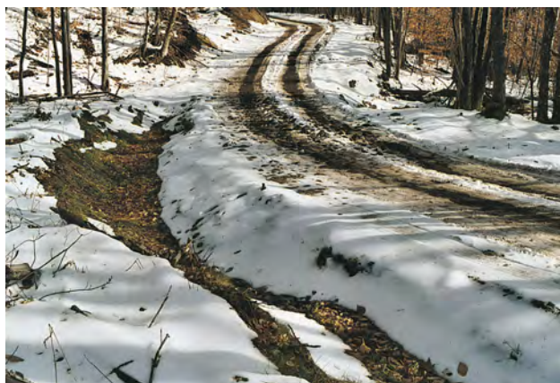
Properly sized ditches capture and slow down runoff.
