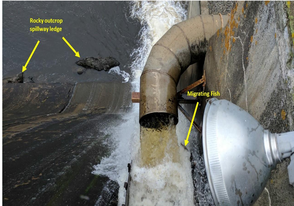
Figure 19. Spillway flume and downstream migrant pipe at Ellsworth Dam. (Source: FERC).
