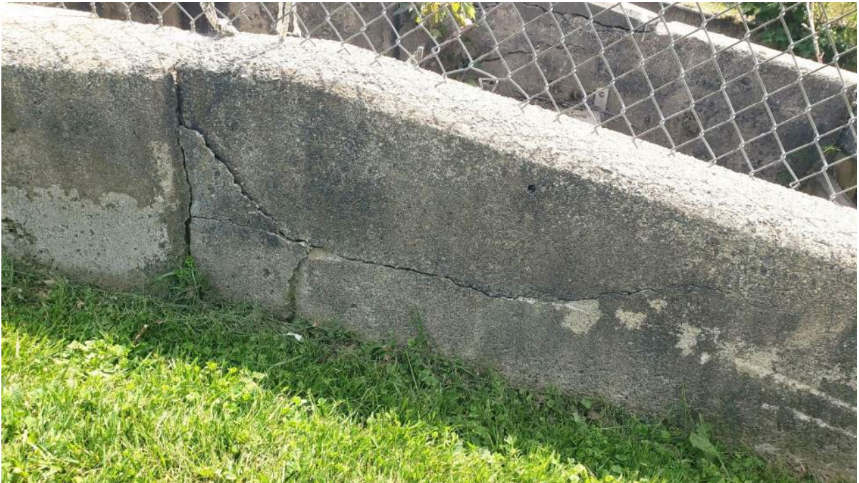
Photo No. 22 – View of right wall of fishway from right embankment, looking left. Note cracking.
