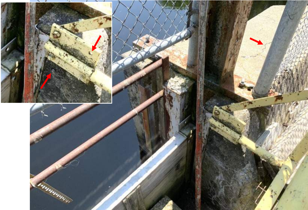
Photo No. 19 – View of left side of fishway intake. Note connection with walkway railing. Two screws appear to have a minimal distance to the edge of the concrete. Note cracking to the left of the fishway intake.
