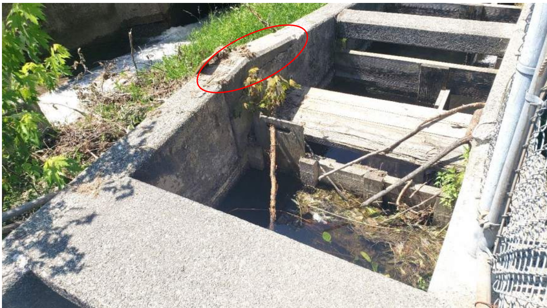
Photo No. 16 – View of top of fishway, looking downstream. Note debris and evidence of concrete repair.
