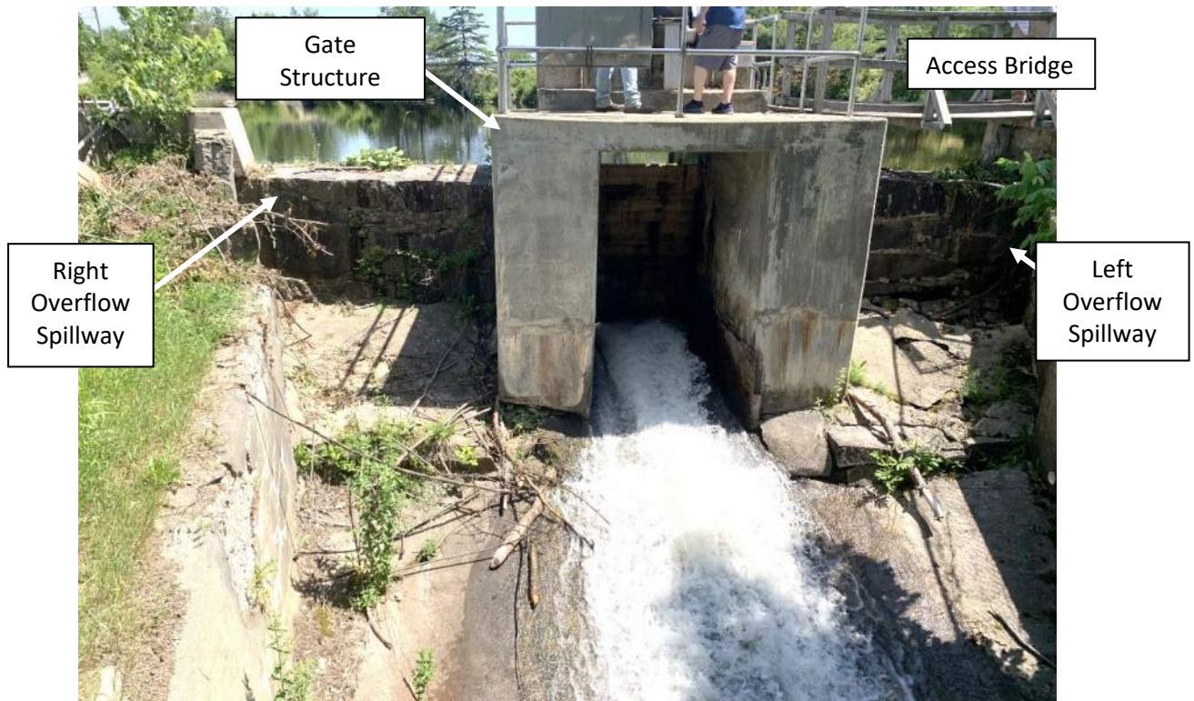
Photo No. 7 – View of dam from Hatchery Road bridge, looking upstream while the gate was opened. Note the debris and vegetation on the spillway aprons.
