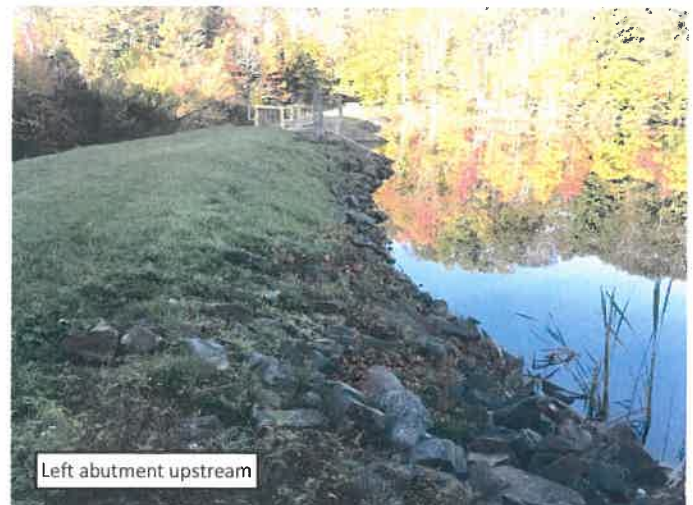
2. Uneven TOD & stone wave protection. Waters edge not straight indicating settlement and/or riprap slippage. No new shorefront development upstream of dam.
