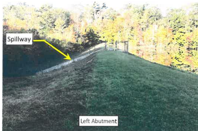
1. Left abutment from top of dam (TOD). Brush recently cut, bank well grassed. Some settlement along TOD. Downstream slope has significant settlement in place.
