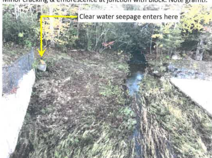
11. Spillway downstream channel between left & right wingwalls silted. Note flattened grass from recent storm.
