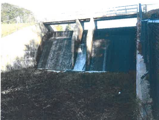
12. Spillway & stoplog weirs. Note the right bulkhead overtopping considerably more than the left & leaking stoplogs leaking. Note difficult access to stoplogs.
