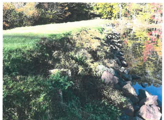
22. Right embankment stone wave protection (rip-rap). Remove brush & rearrange riprap to correct slope. Place new riprap where embankment is exposed.
