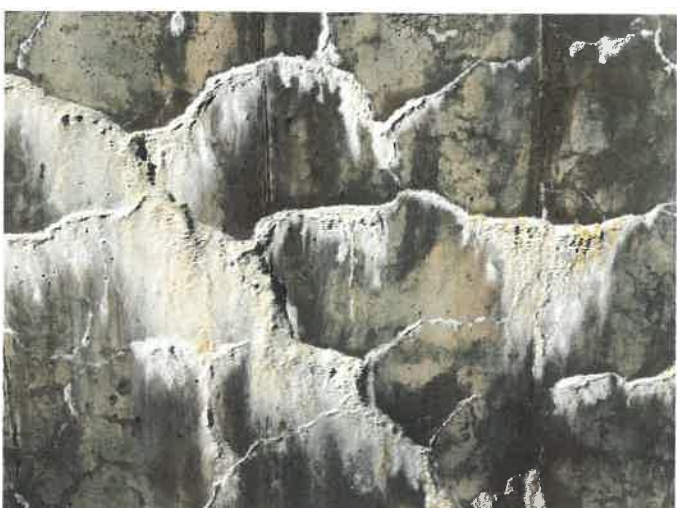
30. Efflorescence (calcium carbonate) caused by evaporation of water seeping through cracks in the channel wall.
