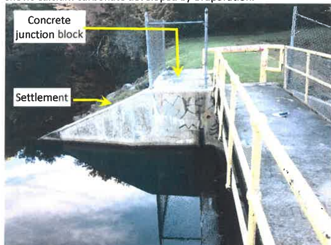
9. Upstream, left mass-gravity retaining wing wall & footbridge. Minor cracking & efflorescence at junction with block. Note graffiti.
