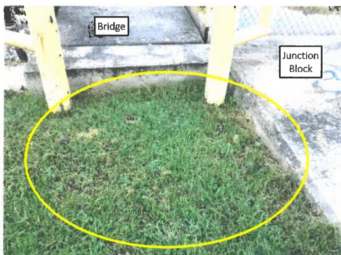
15. Settlement of left embankment at walkway. No defects seen on the concrete junction.
