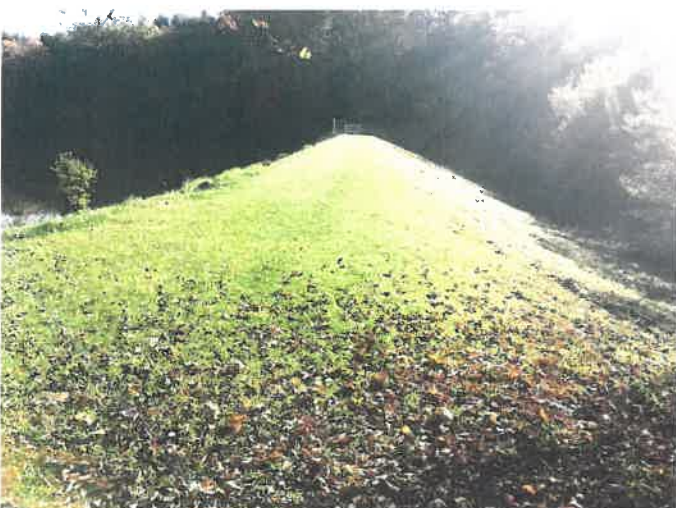
23. Top of Right embankment & downstream face — mostly covered by grass. Downstream face of dam uneven due to local settlement and/or small slips.
