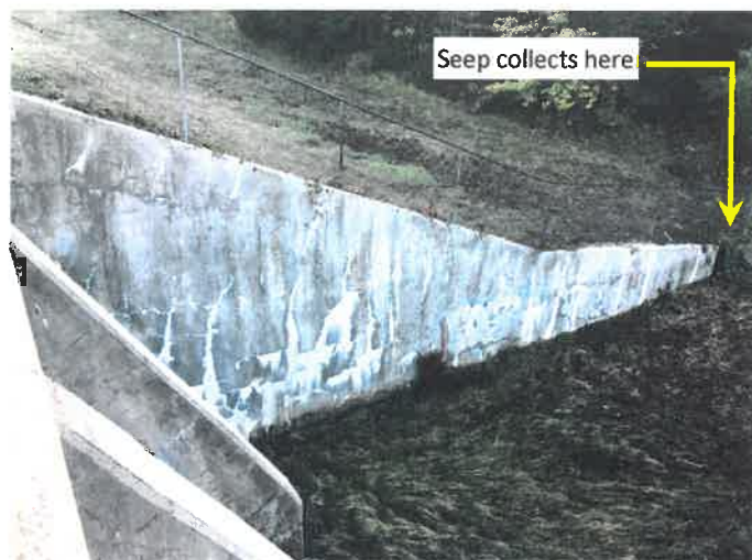
7. Left downstream mass gravity channel. Built 1930, re-faced 1984, with Gunitite. Photos show similar cracks & efflorescence reported by the Army Corps of Engineers (COE) in 1978, A3&A6. Efflorescence shows calcium carbonate developed by evaporation.
