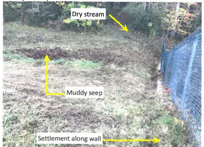
4. Left embankment looking downstream. The brown area is a muddy seep which must be inspected after spring runoff & around labor day & monitored for flow & reservoir stage.
