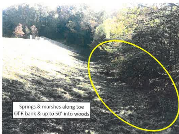
26. View down right embankment toe. Yellow ellipse is area where at least 6 separate marshes have formed. No seepage carried silt or was discoloured.
