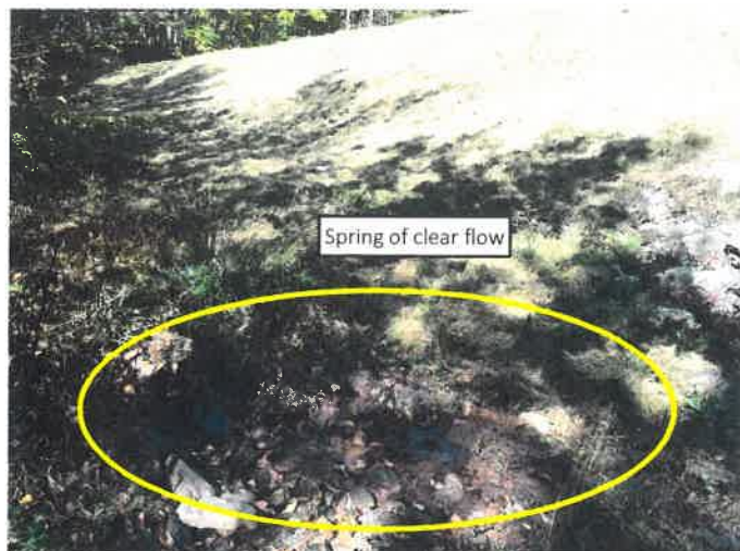
25. Right embankment seepage clear, possibly a toe drain outlet.
