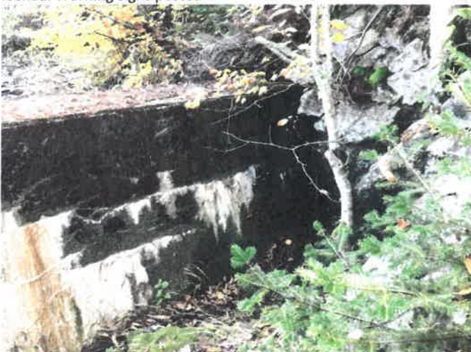
5. Left non-overflow section taken from left downstream. Crack matches horizontal crack in 4. Above. Clear trees & brush to allow for regular easy inspection of abutment. Note ledge.
