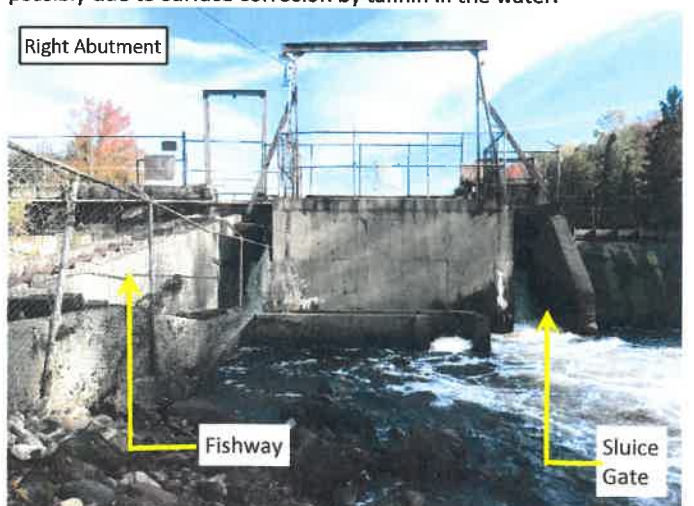
6. View of gate & fishway structure. No movement seen. Concrete spalling & flaking on ogee spillway. Green trace on spillway is either algae or moss. No instability seen.
