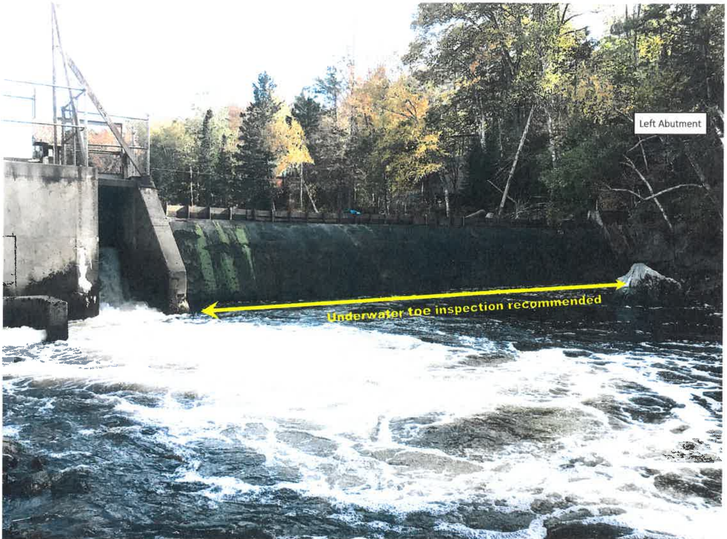
7. Sluice gate & Left concrete ogee weir spillway. Photograph modified to accentuate concrete surface deterioration. Owner requested to have the underwater toe area probed for undercutting by water currents in tail-pond.
