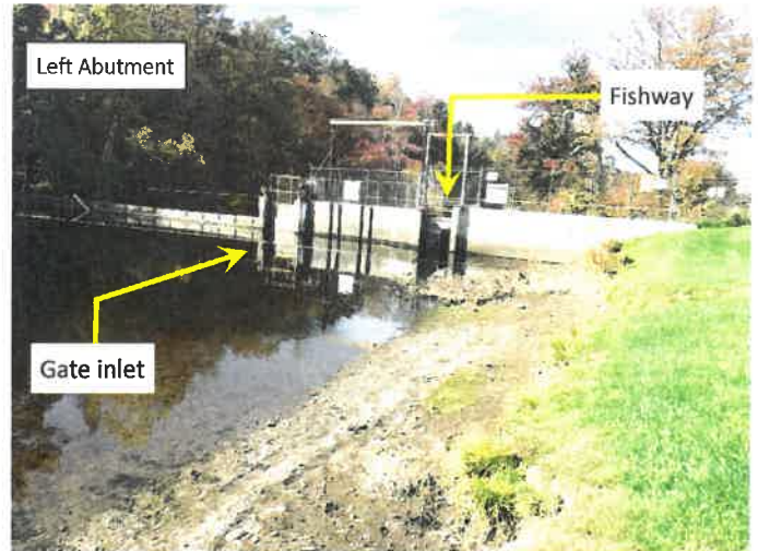
2. View from right upstream shoreline. No debris seen on screen. General concrete deterioration. Security fence, Gate & Fishway functional but rusted in places.
