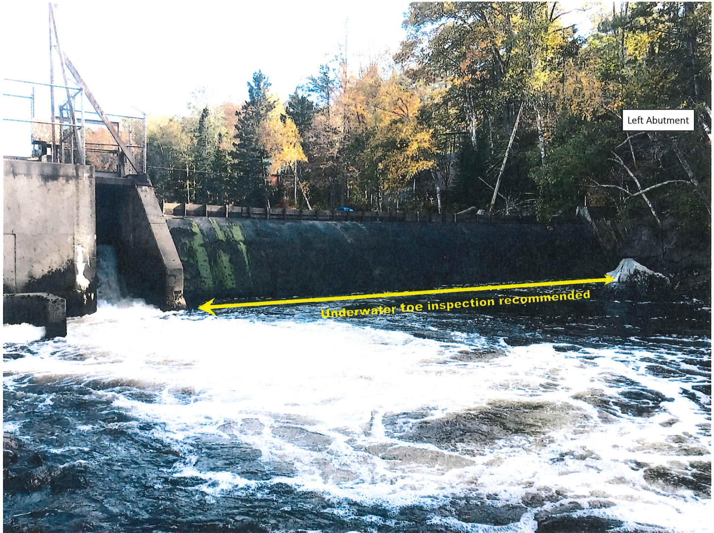
7. Sluce gate & Left concrete ogee weir spillway. Photograph modified to accentuate concrete surface deterioration. Owner requested to have the underwater toe area probed for undercutting by water currents in tail-pond.
