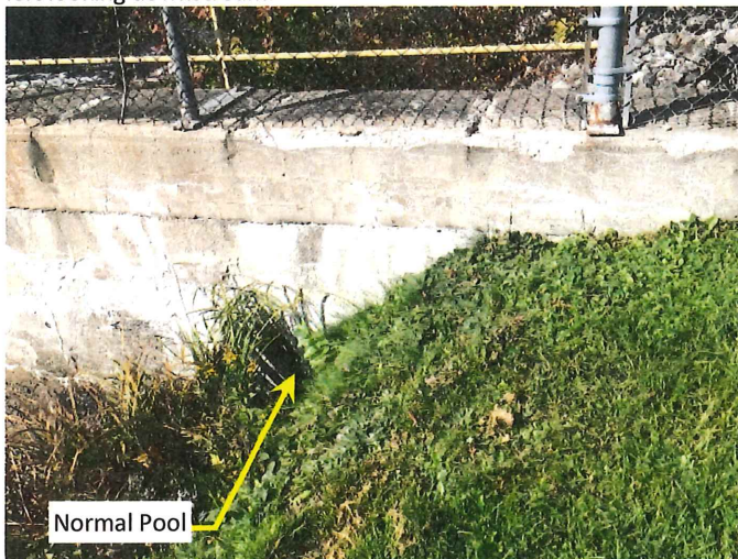
3. Right abutment. Typical surface concrete deterioration. Main body of concrete shows no movement. Fence & poles corroding. Gate locked. Warning signs posted
