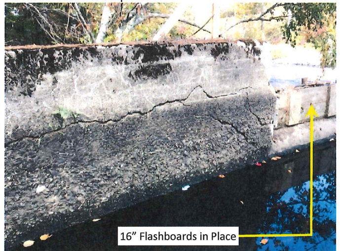
4. Left abutment. Horizontal & diagonal crack through the structure. See photo 5 taken from opposite face. Concrete aggregate exposed possibly due to surface corrosion by tannin in the water.
