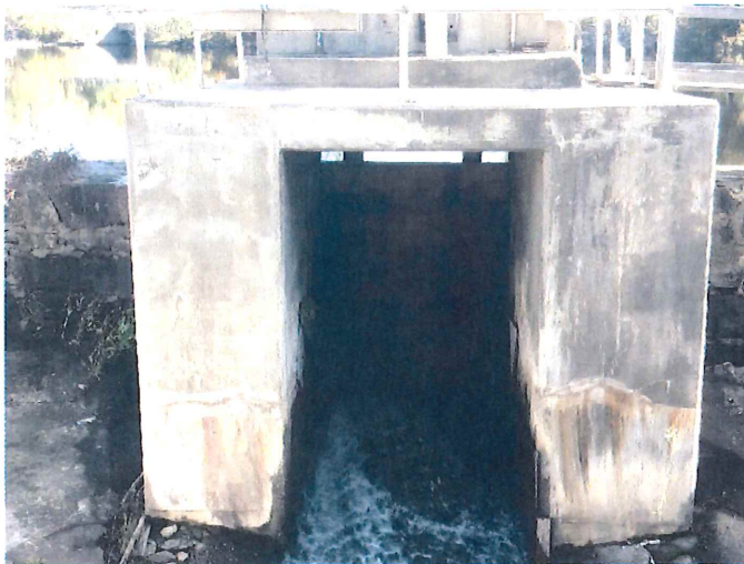
9. Concrete piers & slab housing sluice gate & electric hoist. Rust streaks are likely at construction joints.
