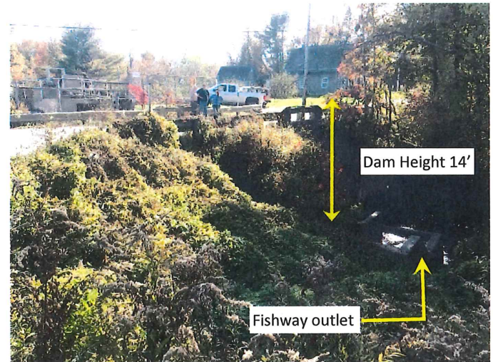
10. Downstream road embankment which merges with the road embankment. Fishway outlet lower right. Toe of dam assumed at channel outlet to bridge.
