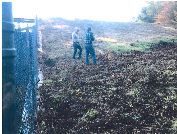
17. Left embankment/wing-wall abutment. Swamp from seepage in the area where the brush has been cut.
