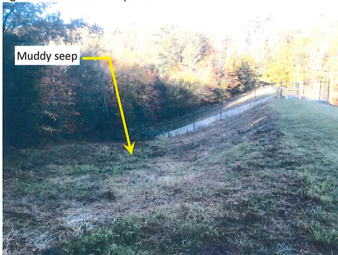
3. Left embankment downstream recently cleared of brush. Both the inclined & level surfaces show unevenness indicating embankment or local slippage.
