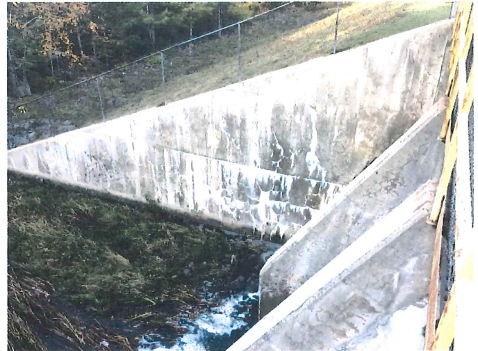
8. Same as A7. Craze cracks & a lift joint can be seen. Efflorescence caused by dissolved free lime in the leak dissolved within the mass gravity concrete wall. No inward deflection or iron oxide from rebar seen along the wall - A18.
