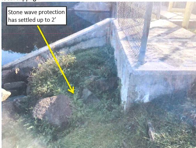
5. Settlement, random boulders & uneven earthwork surface. Concrete cracked but surfaces are plain. This concrete block is connected to the reinforced concrete cutoff wall.
