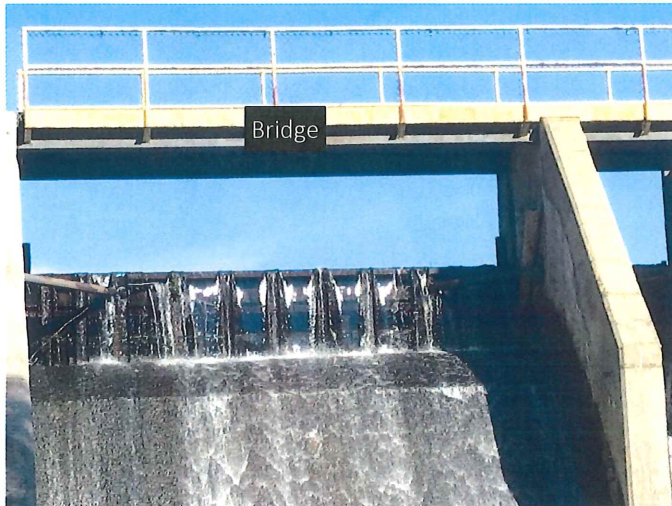
19. Right Spillway. The reason for overflow is that the top of the bulkhead is lower than the left bulkhead.
