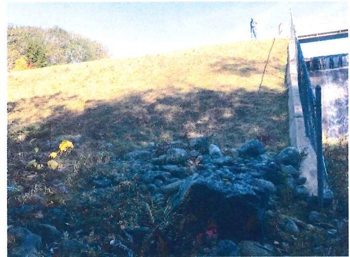
18. Right embankment/wing-wall abutment. Note either settlement or erosion along wall
