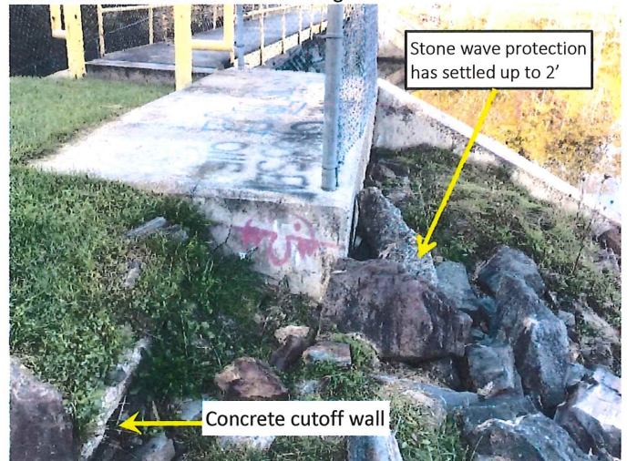
6. Stone wave protection (rip-rap) settled by up to 2 feet at the concrete connecting block - arrow. No visible distress in concrete.
