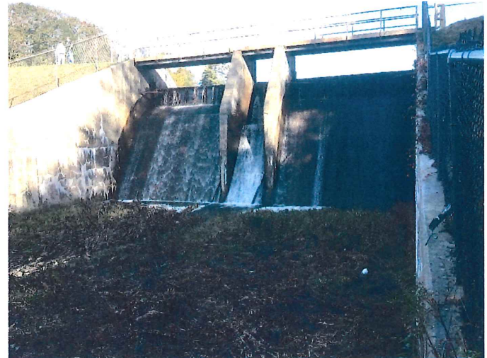
12. Spillway & stoplog weirs. Note the right bulkhead overtopping considerably more than the left & right stoplogs. Note difficult access to stoplogs.
