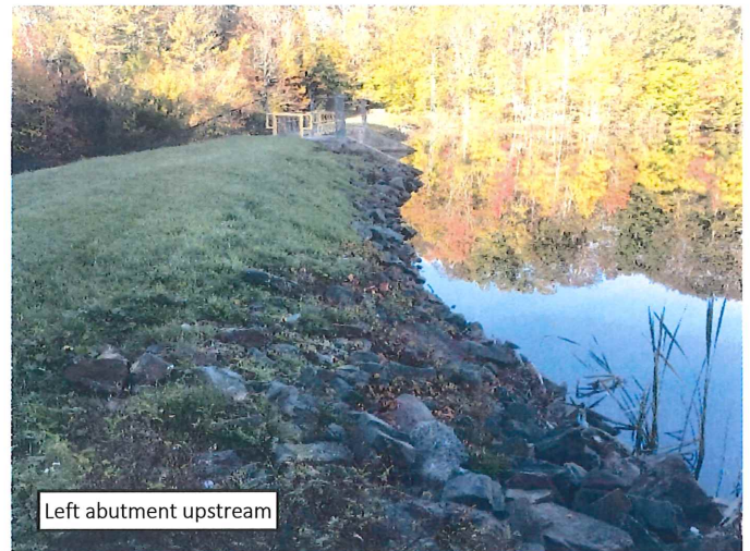
2. Uneven TOD & stone wave protection. Waters edge not straight indicating settlement and/or riprap slippage. No new shoreline development upstream of dam.
