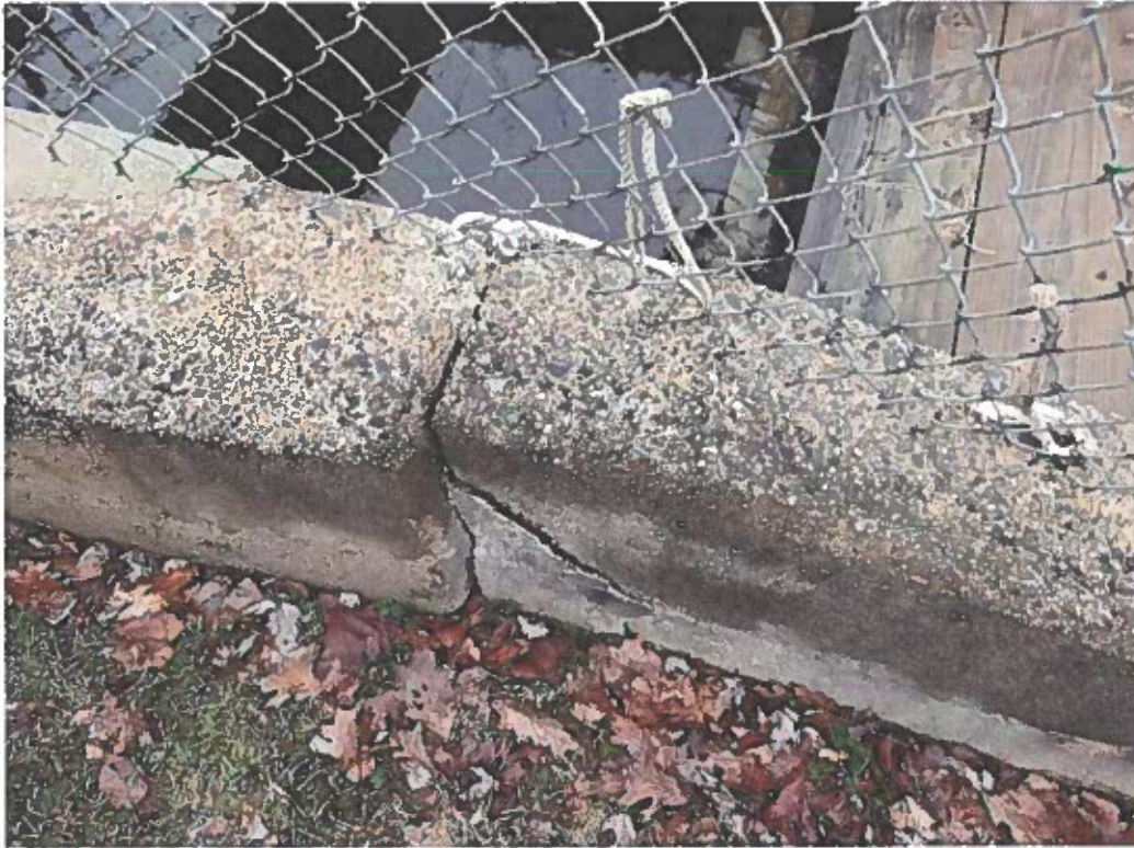
1. The right fishway retaining wall is displaced at concrete joint.
