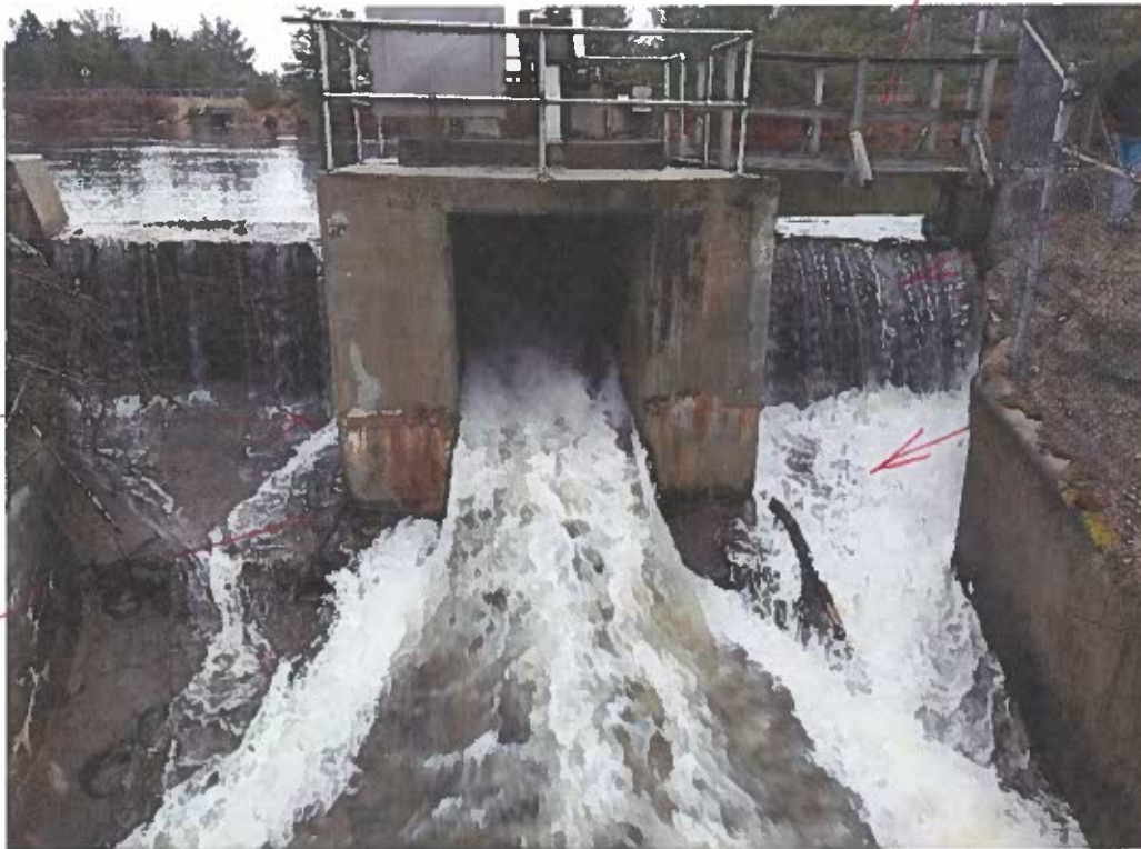
2. The left spillway flows more than right spillway despite originally being level.
