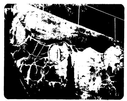
No. 6 VIEW OF DISCHARGE CHANNEL WALL (LEFT SIDE) - NOTE CRACKING EFFLORESCENCE AND SEEPAGE ON WALL
