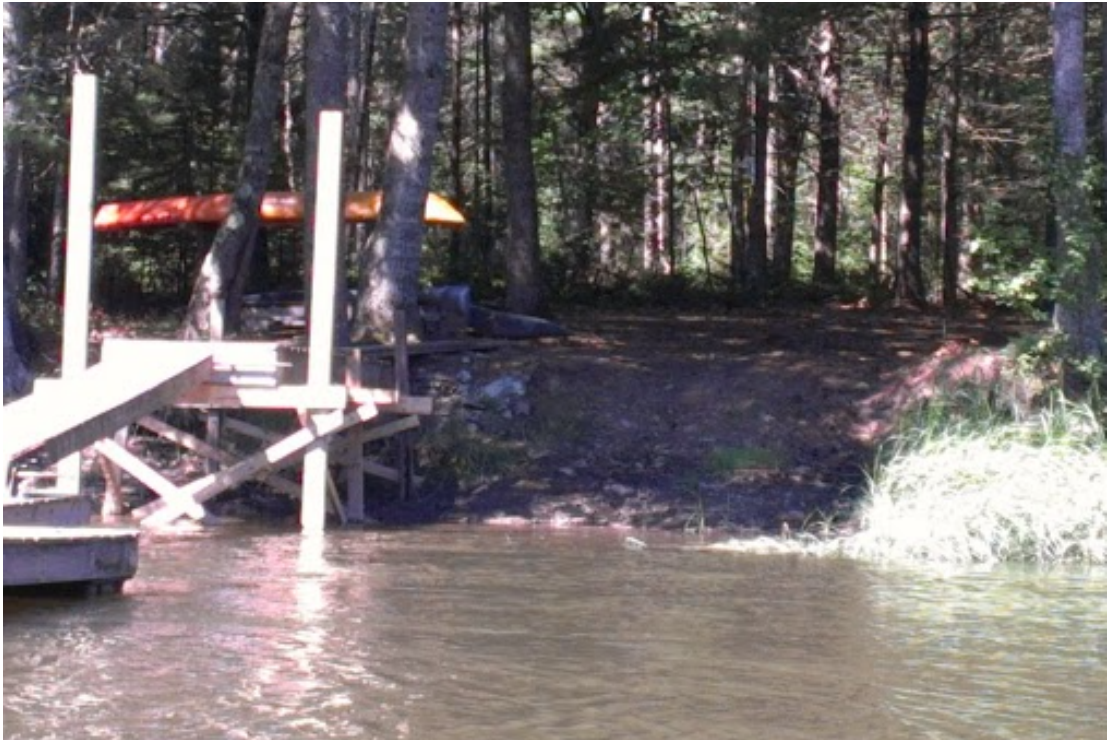
Figure 2. July 31, 2012 photo after completion of Spinney’s permanent pier structure, showing tide level above the second row of permanent pilings.
