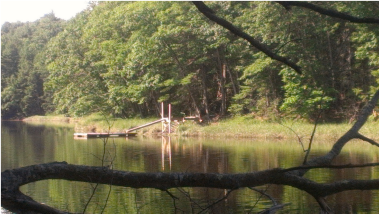
July 13, 2012: The installation is complete. Note longer dock down to the float.
