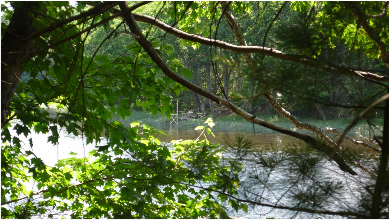
June 24, 2012: The new dock is going in, Jeff Spinney working on it. Note that there now are six pilings into the river bank, making it "more" permanent.
