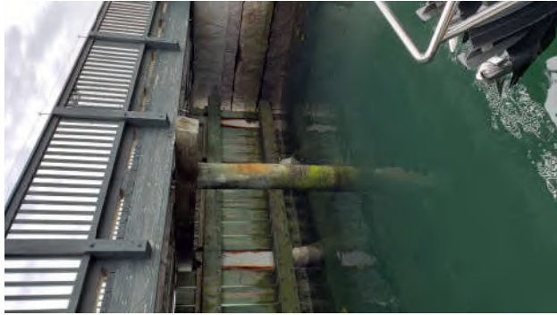
Photo 11: End of Jetty
