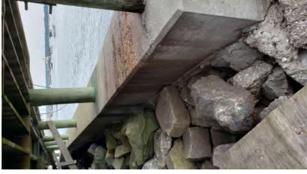
Photo 13: Beginning of Pier
