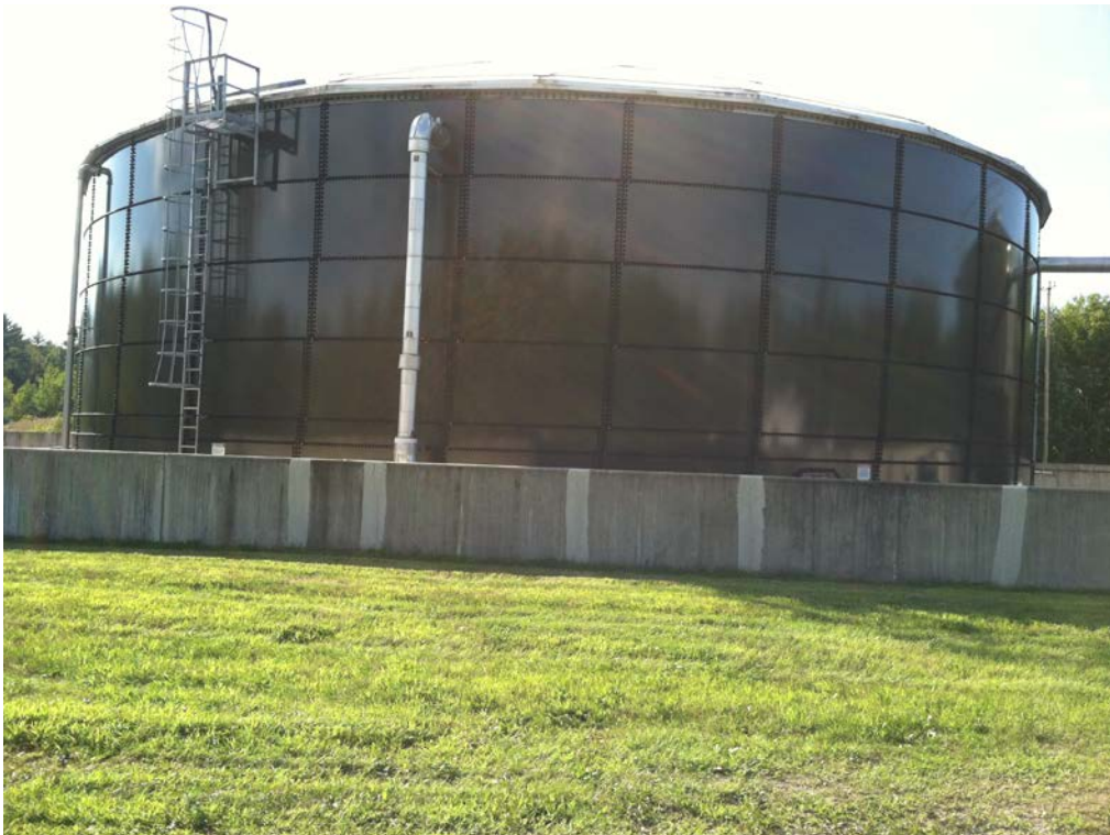
Figure 3. Large Leachate Storage Tank
