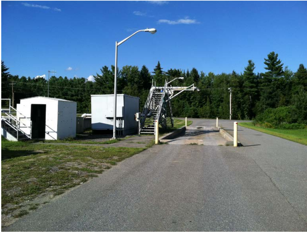
Figure 4. Leachate Load-out Station – Drive-in View
