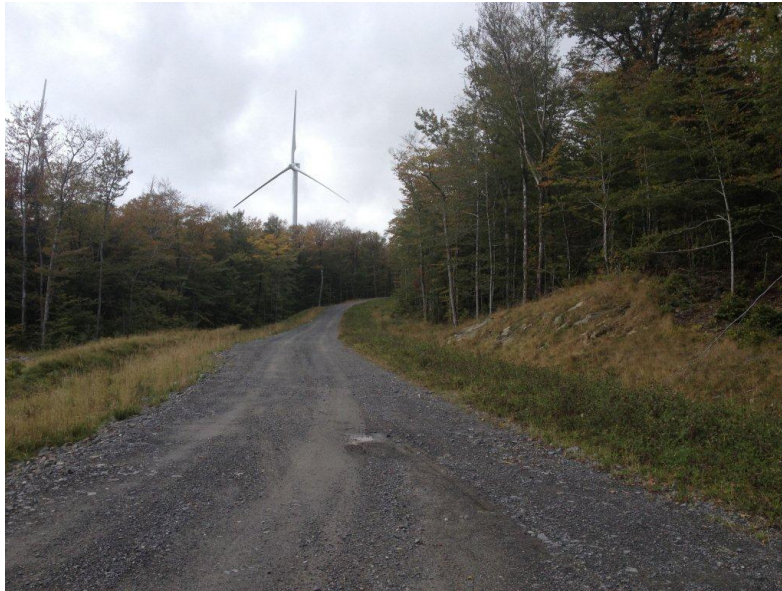
Photo of a post-construction crane road with re-vegetated shoulders at the Sheffield Wind Project after two growing seasons.
