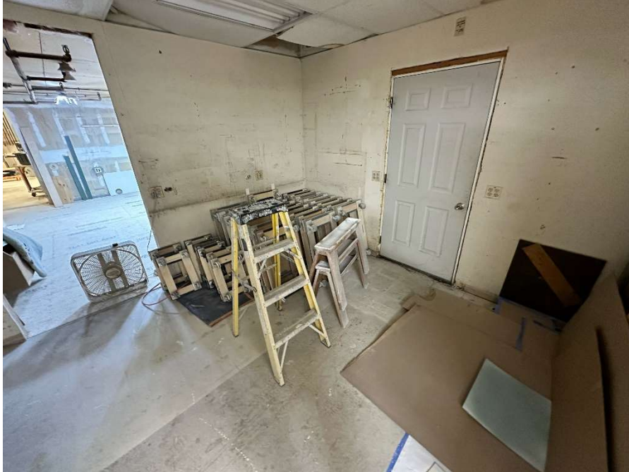
Photo 7: View of the former Micrometrics “chemical storage area” (location shown in Figure 1), in which a stained chemical storage cabinet and flooring were observed and removed as part of the Corrective Action process. The area is currently a storage space for woodworking equipment. MEDEP did not observe staining or other indicators of hazardous waste release.
