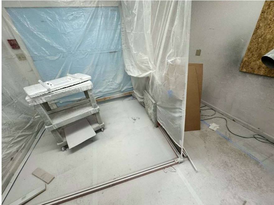
Photo 6: Latex paint finishing area in the southern portion of the building.
