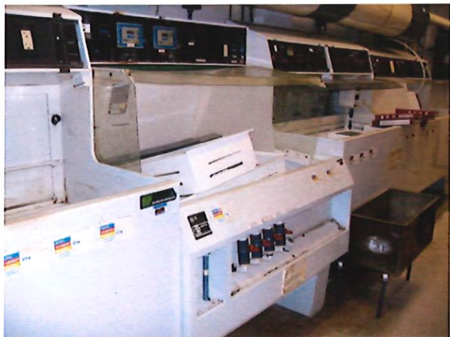
A view of four sinks located in the Etch Room that were tested, neutralized, flushed, and dried by Clean Harbors. The sinks are to remain in the building.
