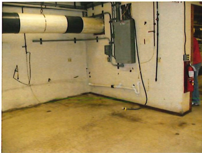
A view of the former location of three sinks in the Finish Room that were removed by Clean Harbors.
