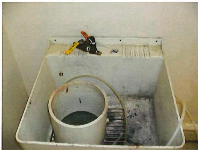
A view of the sink in the Paint/Brand Room.
