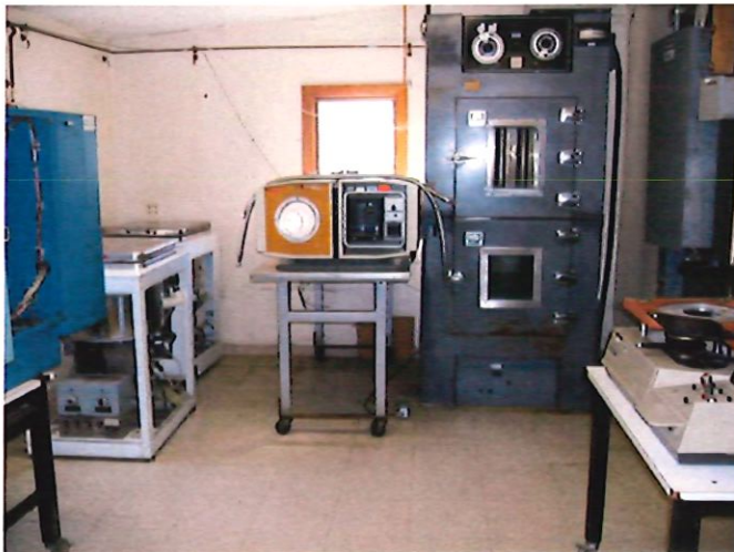
A view of the remaining equipment in the southwest portion of the Environmental Area.
