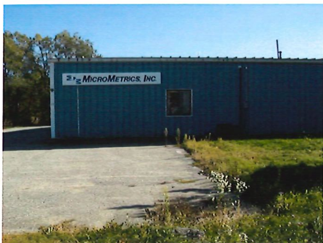
A view of the MicroMetrics facility looking south.
