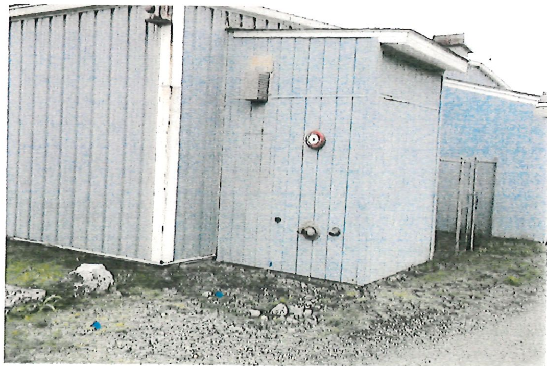
2. View of water connection, northwest corner.
