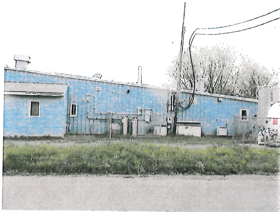
3. West side of Knox building.
