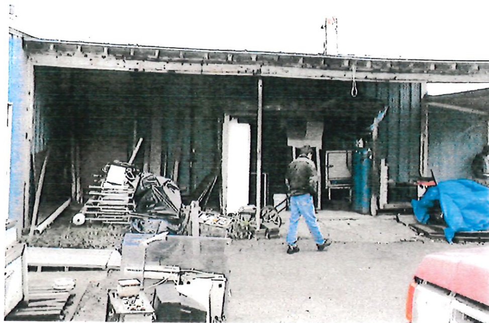
5. View of canopy from southeast.
