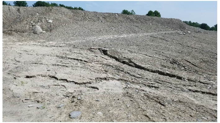
July 3, 2018: After placement of soil. View is to the north of a soil stockpile in the northern portion of the Site. Stormwater rills typical across entirety of Site.
