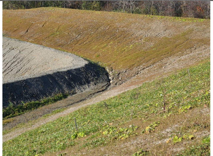
November 9, 2021: Post-Construction. View is to the east from the top of the northern soil berm. Note stormwater rills on the interior northeast corner of the northern soil berm. The City indicated they will install riprap in this area.
