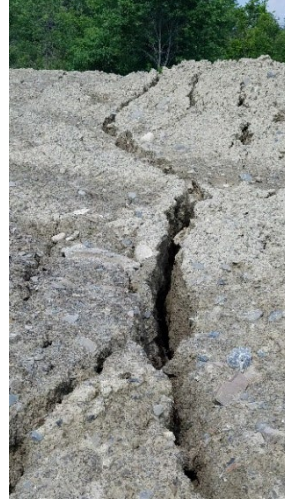
July 3, 2018: After placement of soil. Large stormwater rill, typical.
