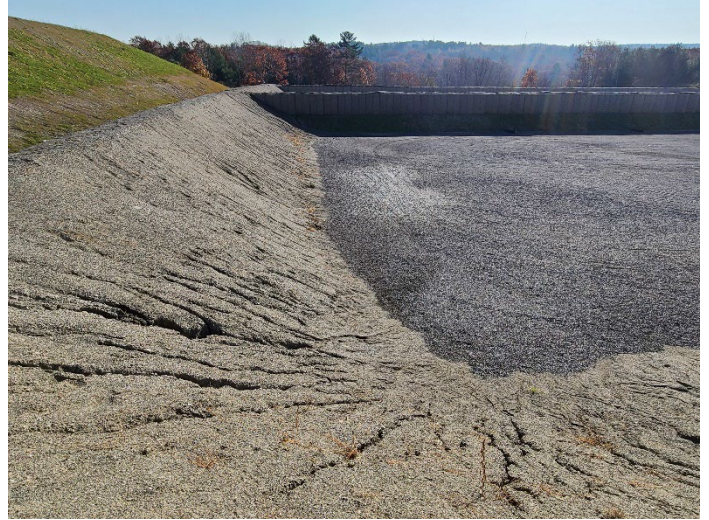
November 9, 2021: Post-Construction. View is to the east, along to the top of the firing range impact wall (sand) in the northeastern portion of the Site. Note (unavoidable) stormwater rills on the northern firing range impact wall. The City has indicated they will install silt collectors or hay bales on culverts between the firing range bays to prevent stormwater from transporting sand towards the river to the east.
