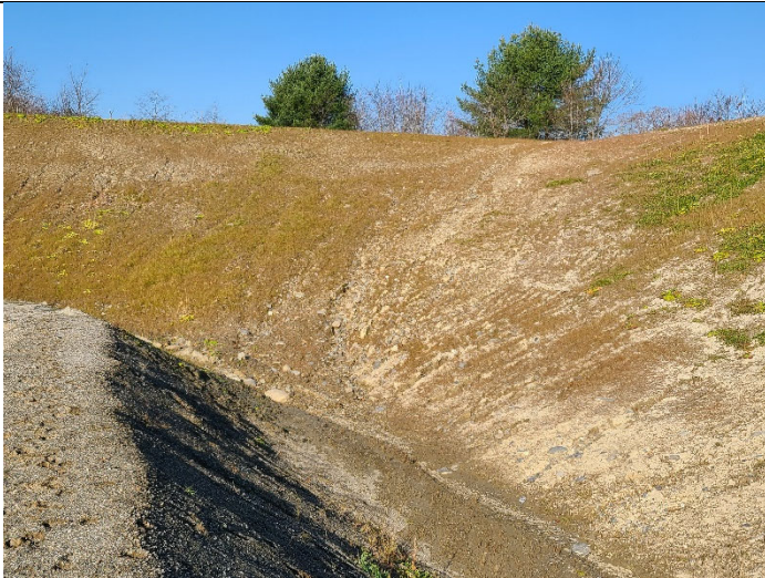
November 9, 2021: Post-Construction. View is to the northeast from the top of the firing range impact wall (sand) with northern soil berm to the right. Note stormwater rills on the interior northeast corner of the northern soil berm. The City indicated they will install riprap in this area.
