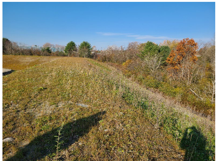
November 9, 2021: Post-Construction. View of the top and the northern/back side of the northern soil berm. Note good grass capture and minimal stormwater impacts.
