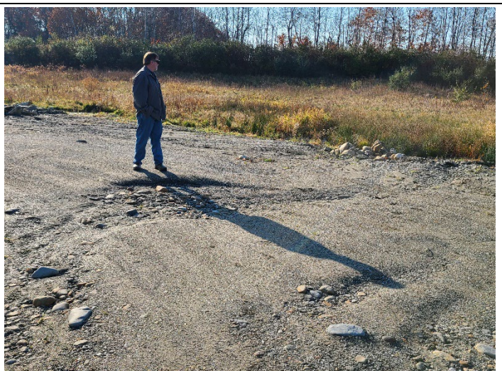
November 9, 2021: Post-Construction. Stormwater impacts at the end of the central berm. The City has indicated that a culvert and riprap apron will be installed in this area.
