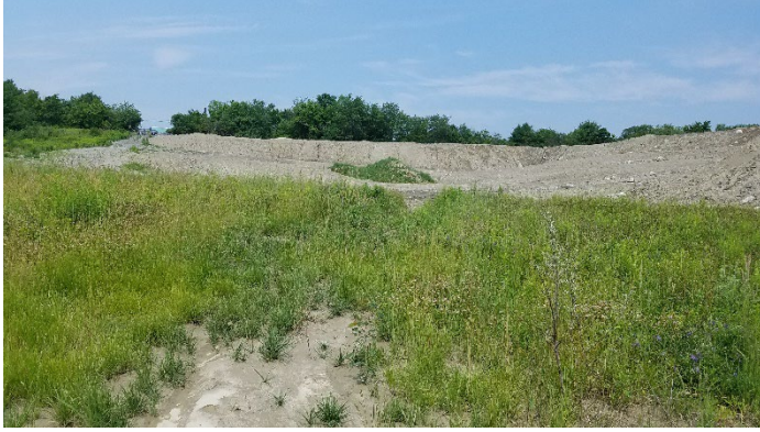
July 3, 2018: After placement of soil. View is to the west from the eastern edge of the property (the Site entrance can be seen in the left portion of the horizon). Note sediment runoff from the Site in the foreground leading towards the adjacent River.
