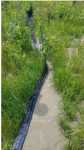
July 3, 2018: After placement of soil. View of silt fence installed along eastern edge of property. Note that silt fence is overwhelmed by sediment and failing.
