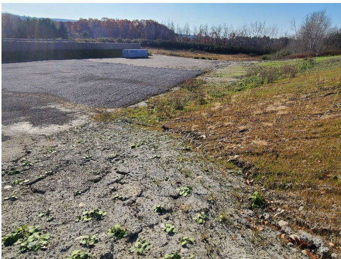
November 9, 2021: Post-Construction. View is to the southeast from the top of the firing range impact wall towards the western firing range bay. Note stormwater impacts from the northeastern portion of the Site onto the surface of the firing range. The City has indicated that additional work will be performed in this area.
