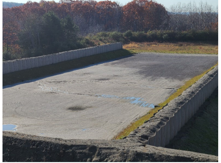
November 9, 2021: Post-Construction. View is to the southeast from the top of the northern soil berm. This overview of the eastern firing range shows stormwater passing through culverts and running across the gravel surface of the firing range, towards the river to the east. The City will install silt collectors on the culverts.
