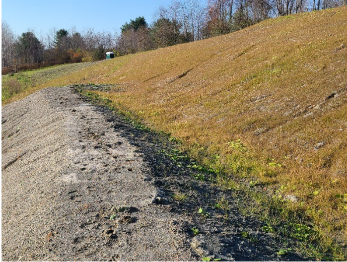
November 9, 2021: Post-Construction. View is to the south, along to the top of the firing range impact wall (sand) with the western soil berm to the right. Note stormwater rills on the western soil berm.
