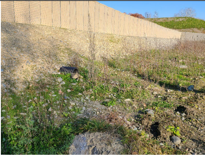
November 9, 2021: Post-Construction. View is of the eastern side of the eastern berm. Note culvert outfalls beneath the berm, typical and minor stormwater rills.
