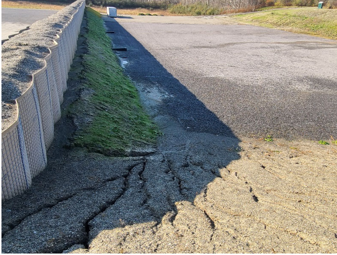
November 9, 2021: Post-Construction. View is to the south showing (unavoidable) stormwater impacts to the firing range impact wall (sand). Stormwater flows along the inside of the berm before passing through a culvert. The City has indicated they will install silt collectors or hay bales on these culverts to prevent stormwater from transporting sand towards the river to the east.
