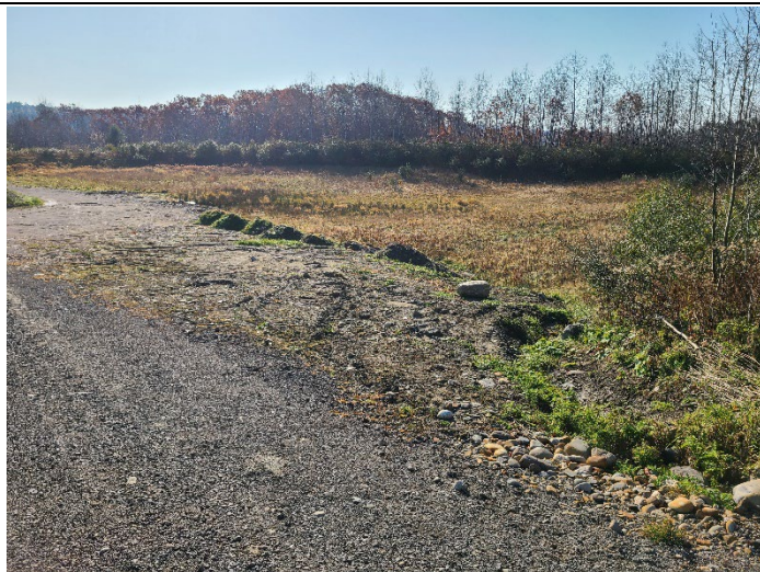
November 9, 2021: Post-Construction. Minor stormwater runoff issues along the southern side of the site access road (the City indicated ditches and a culvert will be installed).
