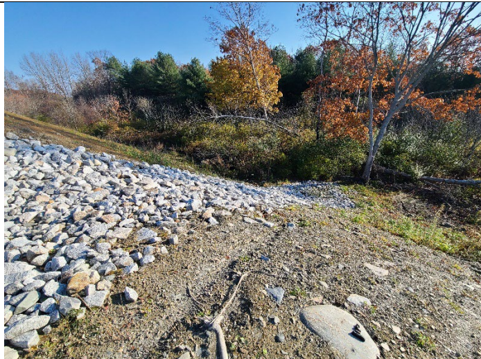
November 9, 2021: Post-Construction. Riprap outfall from the stormwater plunge pool. Discharge is to the east towards the river.
