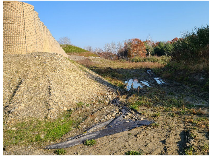
November 9, 2021: Post-Construction. View is to the north, from the end of the eastern berm separating the eastern firing range bay from undeveloped area to the east. Note construction impacts of the ground surface and exposed geotextile fabric. The City has indicated that earthwork repair will occur in this area.
