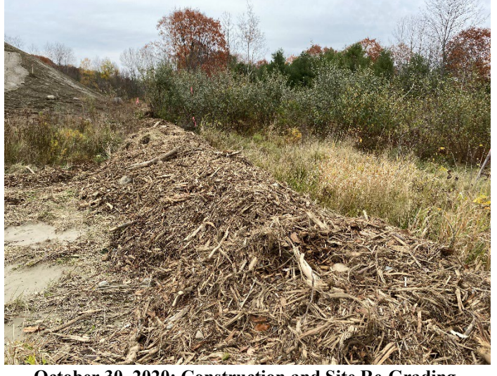
October 30, 2020: Construction and Site Re-Grading. Erosion control mulch berm at eastern edge of property, typical.
