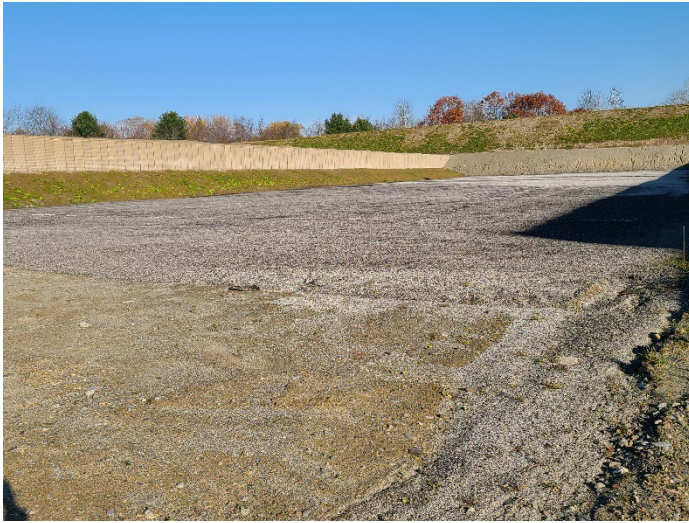
November 9, 2021: Post-Construction. View is to the northwest, from the end of the eastern firing range bay. Note stormwater rills in the picture foreground. The City has indicated that earthwork repair will occur in this area (and the area to the east of the eastern firing range bay).
