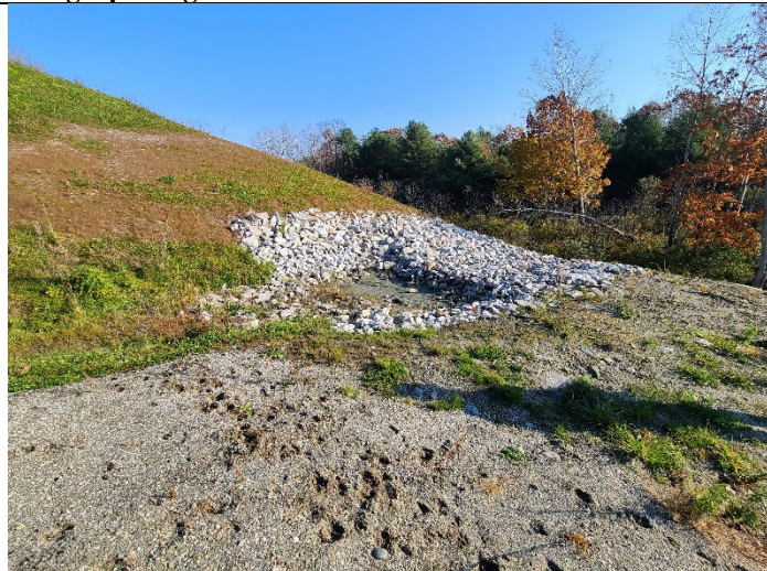
November 9, 2021: Post-Construction. View of stormwater plunge pool installed along the top of the northern soil berm.
