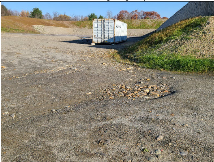
November 9, 2021: Post-Construction. View is to the north, from the end of the central berm. Note evidence of stormwater runoff. The City has indicated that a culvert and riprap apron will be installed in this area.
