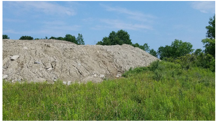
July 3, 2018: After placement of soil. View is to the west, from the eastern edge of the Site of a soil stockpile in the northern portion of the Site. Note stormwater rills along the back of the stockpile.
