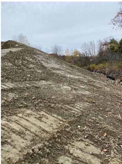
October 30, 2020: Construction and Site Re-Grading. Northern edge of the soil stockpile in the northern portion of the Site. Note silt fence at the bottom of the slope.
