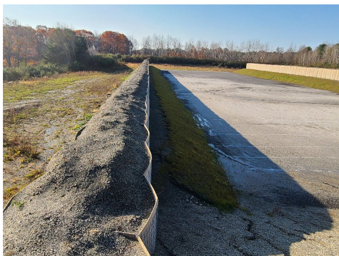
November 9, 2021: Post-Construction. View is to the south showing the top of the eastern sand-filled berm separating the eastern firing range from the eastern undeveloped area.
