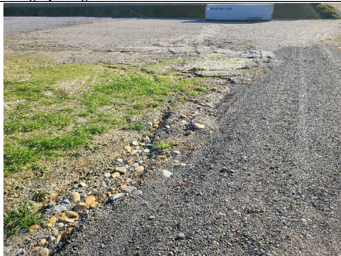
November 9, 2021: Post-Construction. Minor stormwater runoff issues along the northern side of the site access road (the City indicated ditches and a culvert will be installed).
