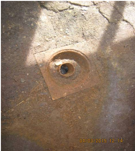
Additional floor drain in boiler room.
