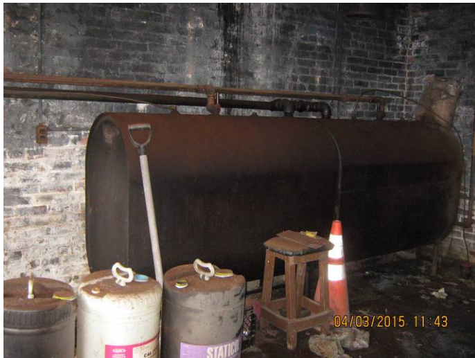
Two 275-gallon heating oil ASTs and three empty, plastic drums in boiler room.
