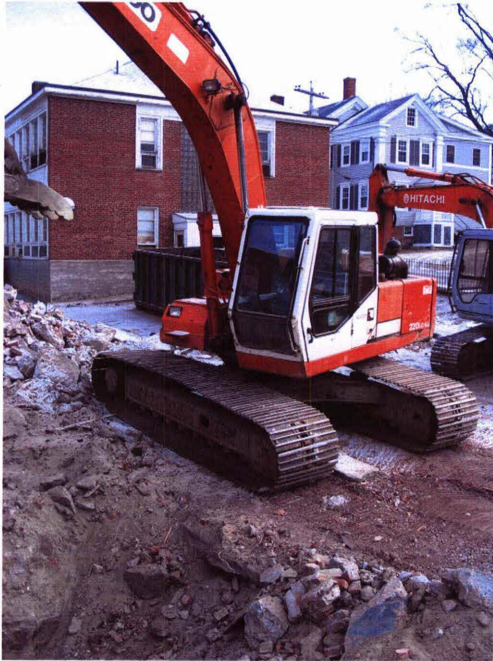
WINTHROP COMMERCIAL CENTER BOILER ROOM DEMOLITION 3-1-2006 P. BLANCHARD A-157-2005
