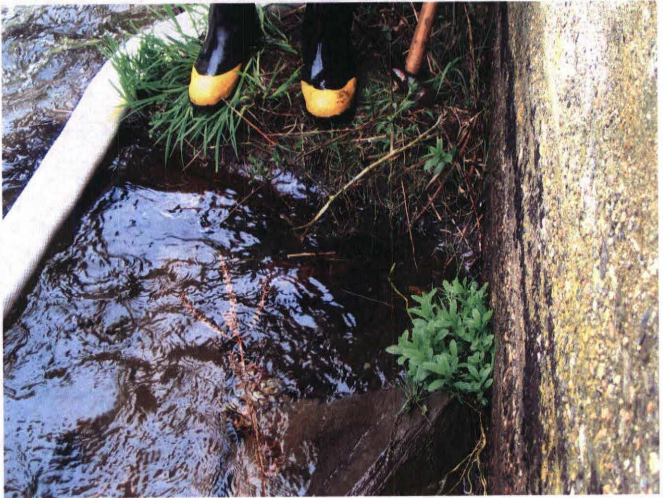
SNEEN ON MILL STREAM BOILER ROOM FOUNDATION 5-27-2005 A-157-2005 P. BLANCHARD
