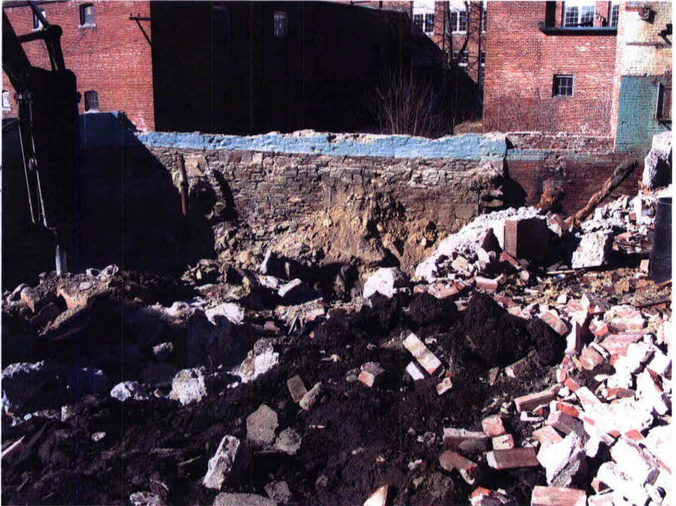
WINTHROP COMMERCE CENTER DEMOLITION BOILER ROOM 3-7-2006 P. BLANCHARD A-157-2005
