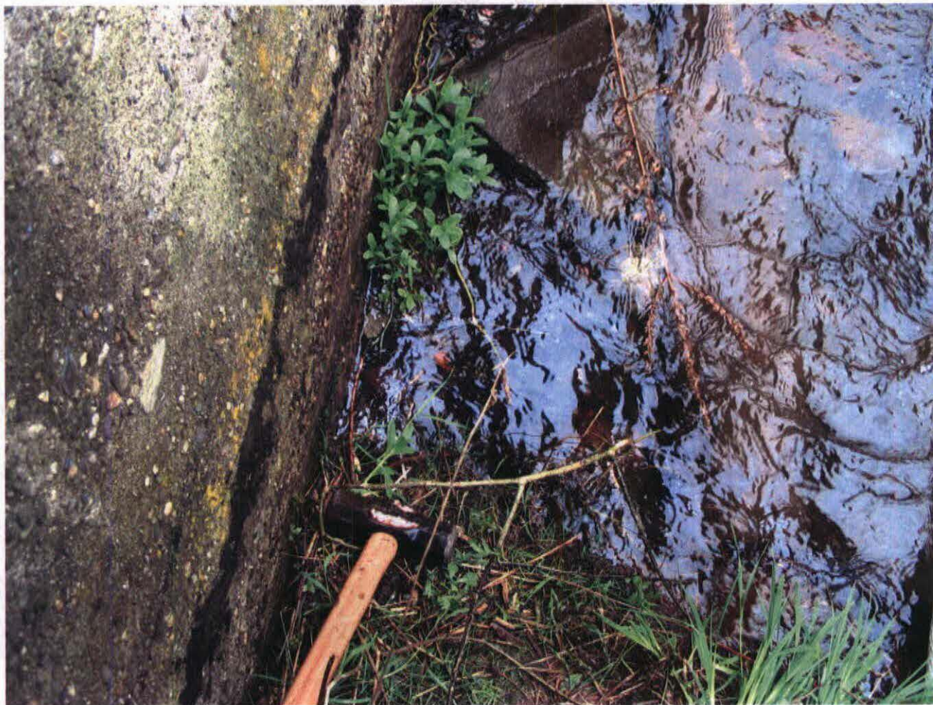
SNEEV ON MILL STREAM BOILER ROOM FOUNDATION 5-27-2005 A-157-2005 P. BLANCHARD
