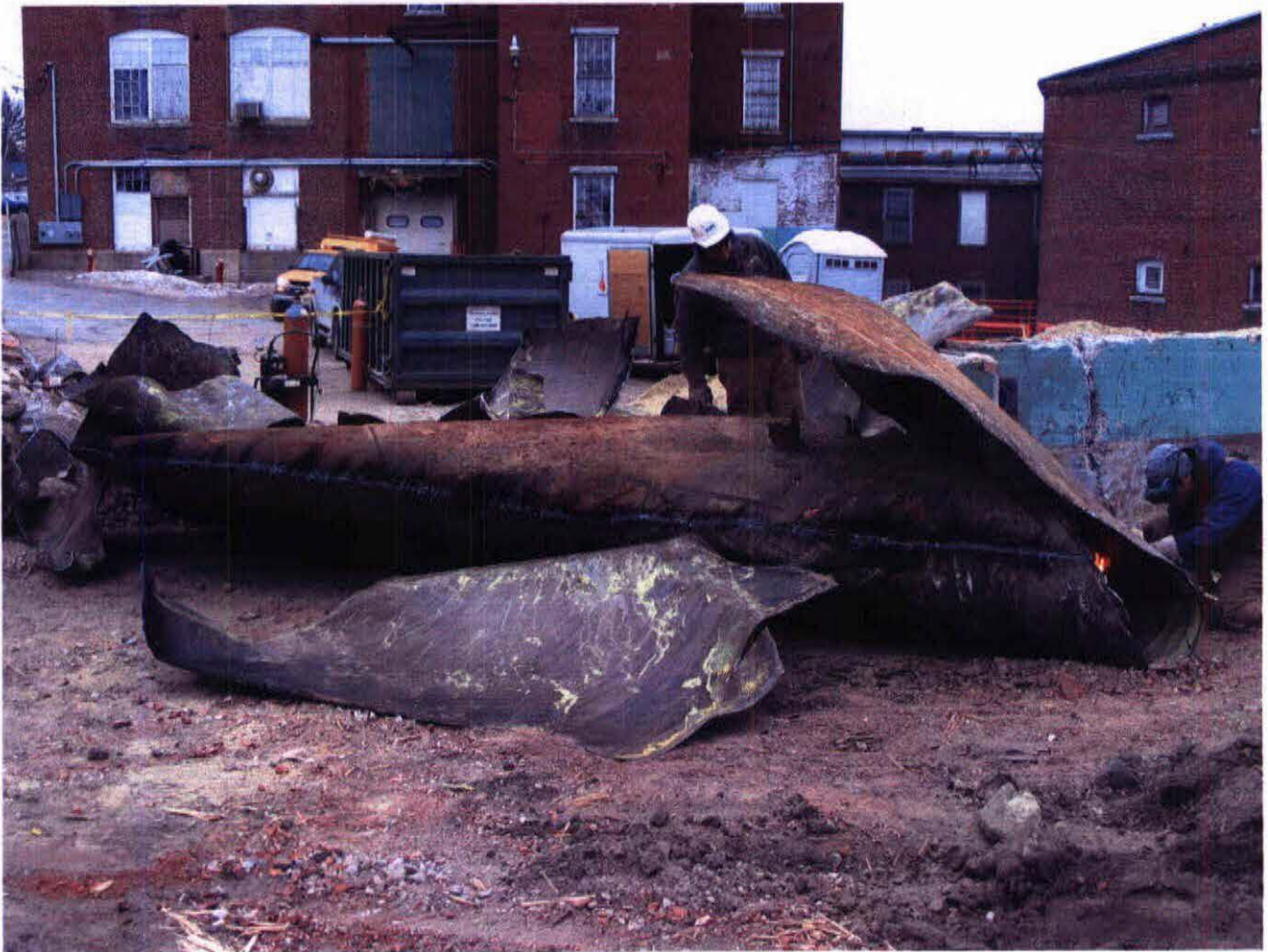
WINTROP COMMERCE CENTER REMOVED U.S.I. CUTTING UP FOR SCRAP 3-2-2006 P. BLANCHARD A-157-2006
