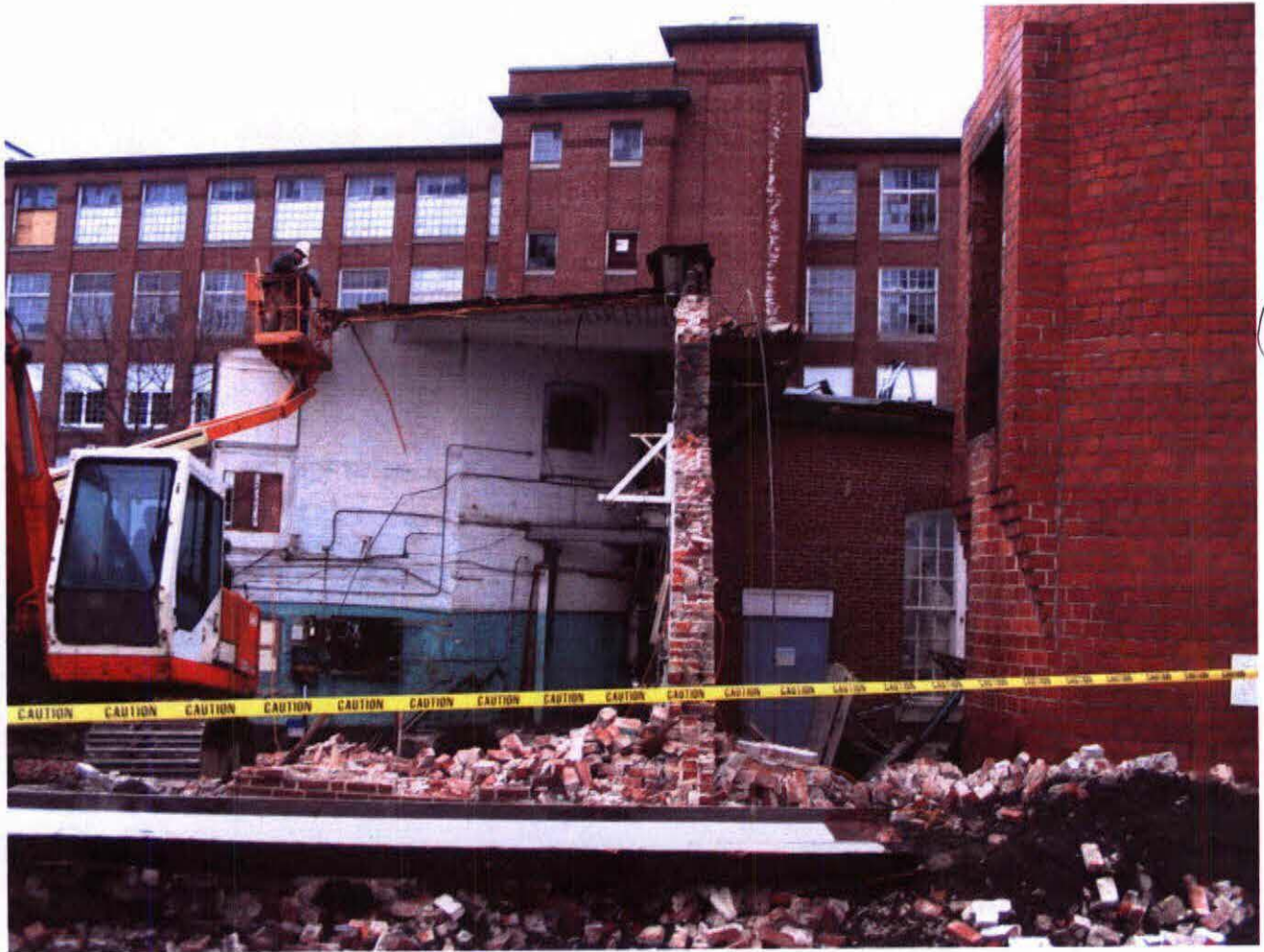
WINTHROP COMMERCE CENTER BOILER ROOM DEMOLITION 2-17-2006 P. BLANCHARD A-157-2005
