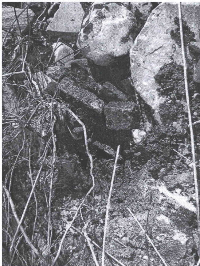
Photograph No. 1, Oil Seep Below Boiler Room
