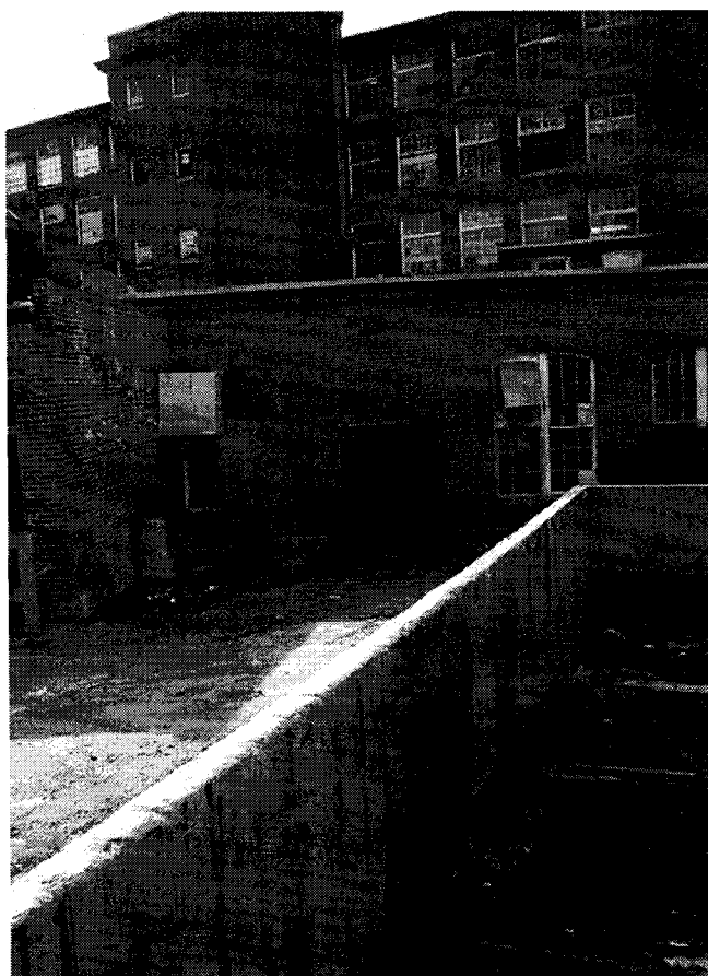
Photograph No. 7 Storm Drain Location
