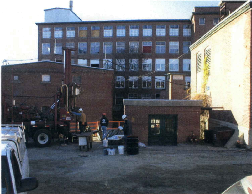
Installation of soil boring SB-2 near the pump house
