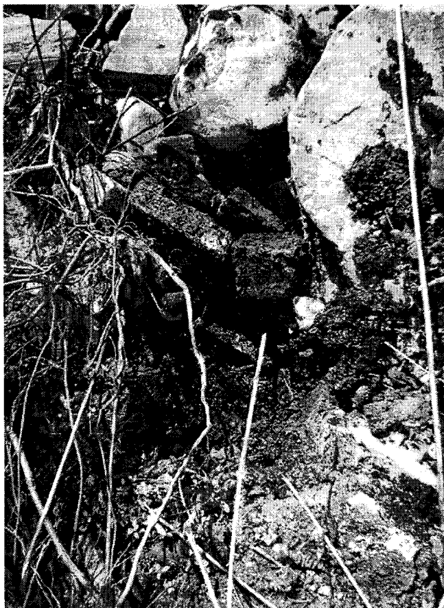
Photograph No. 1, Oil Seep Below Boiler Room
