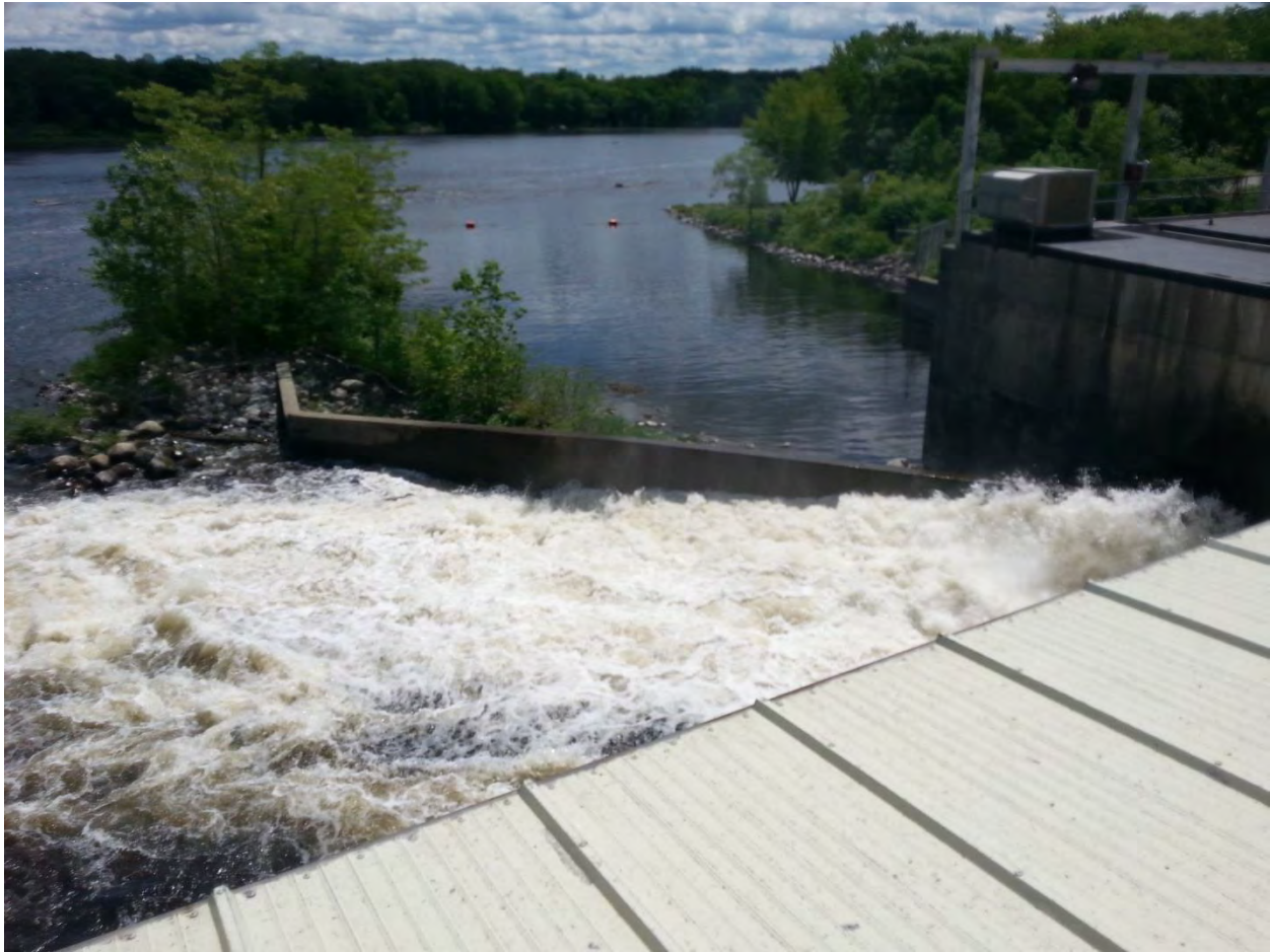
FIGURE 11: VIEW FROM THE PLATFORM ON THE DOWNSTREAM END OF THE FOREBAY BETWEEN THE TWO POWERHOUSES LOOKING DOWNSTREAM.
