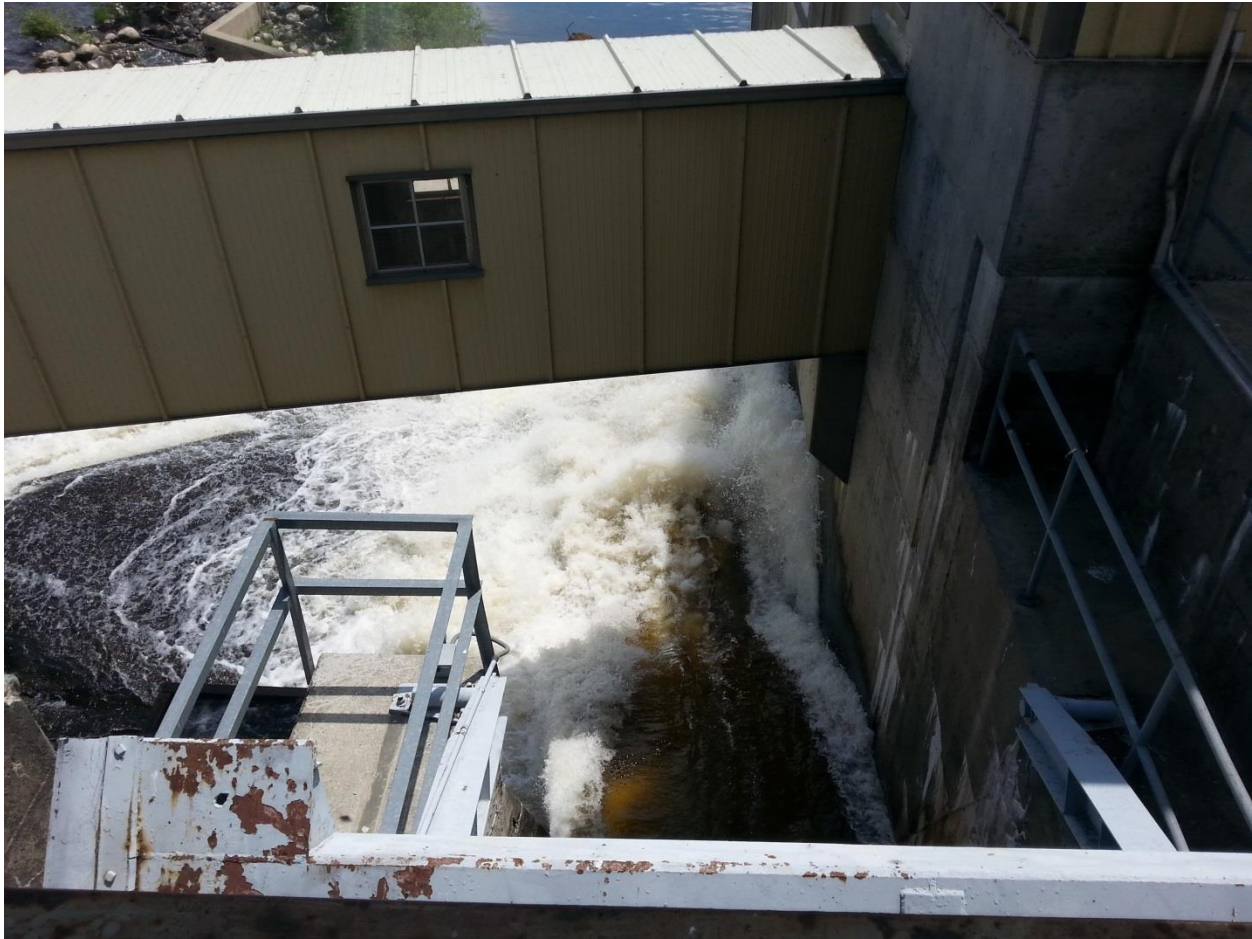
FIGURE 10: VIEW FROM ABOVE THE TAITNER GATE LOOKING DOWNSTREAM.
