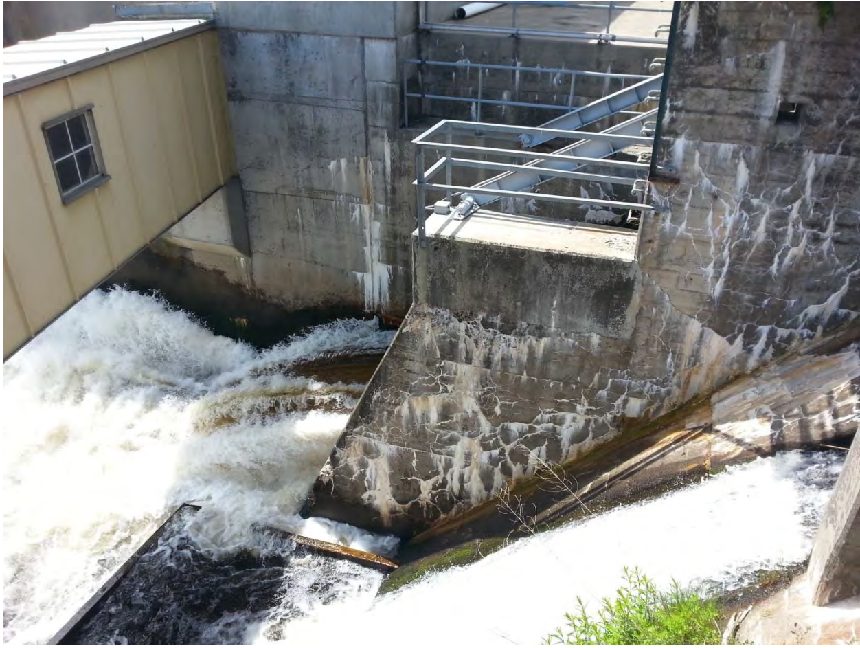
FIGURE 9: VIEW FROM AN ACCESS PLATFORM BEHIND THE UNITS 1 THROUGH 6 POWERHOUSE LOOKING AT THE DISCHARGE FROM THE TANTER GATE SHOWN IN FIGURE 8.
