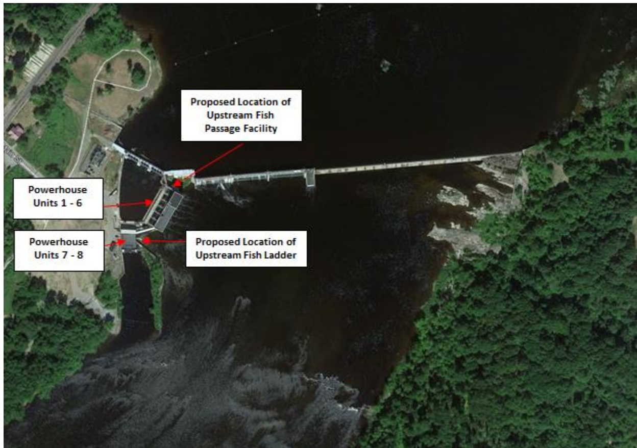
FIGURE 2. SHAWMUT DAM, POWERHOUSES, TAILRACES, PROPOSED LOCATION OF UPSTREAM FISH PASSAGE FACILITY (PHOTO YEAR: 2018)
