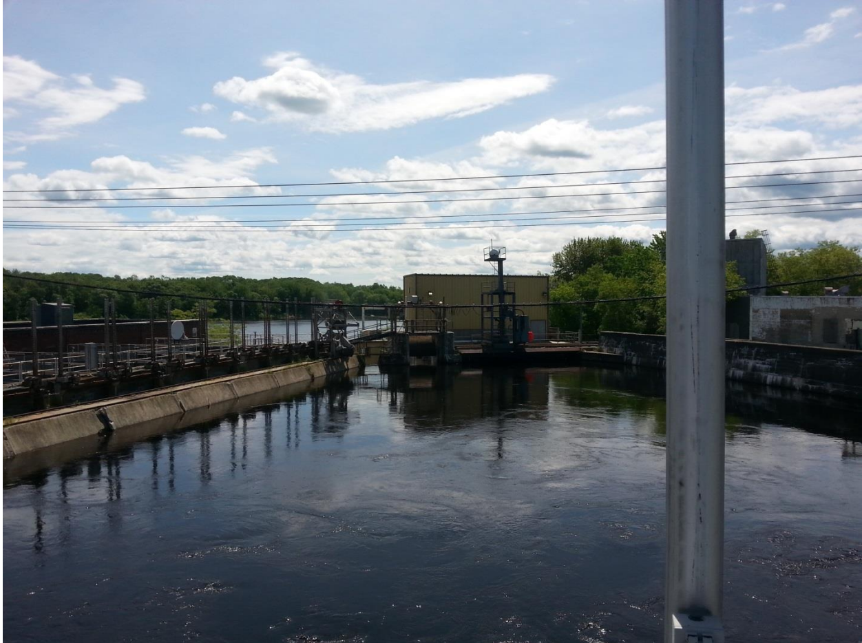
FIGURE 7: VIEW FROM ABOVE THE HEAD GATE STRUCTURE LOOKING DOWNSTREAM INTO THE FOREBAY.
