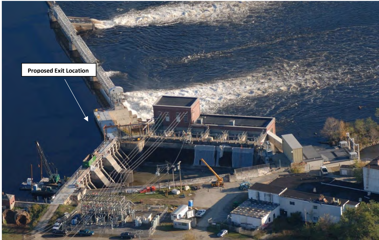
FIGURE 4. PROPOSED EXIT LOCATION FROM UPSTREAM FISH PASSAGE FACILITY (PHOTO DATE: 10/12/09)
