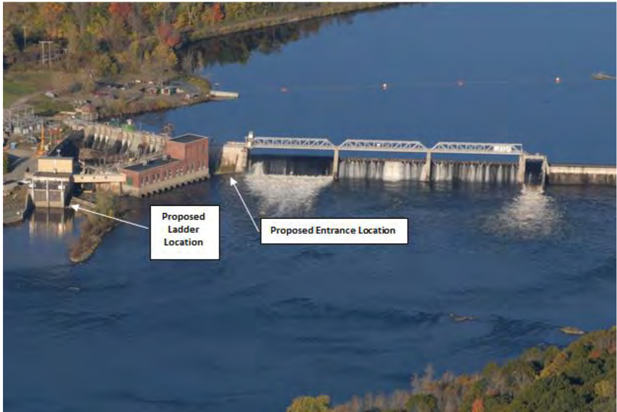
FIGURE 3. PROPOSED ENTRANCE LOCATION TO UPSTREAM FISH PASSAGE FACILITY AND FISH LADDER (PHOTO DATE: 10/12/09)
