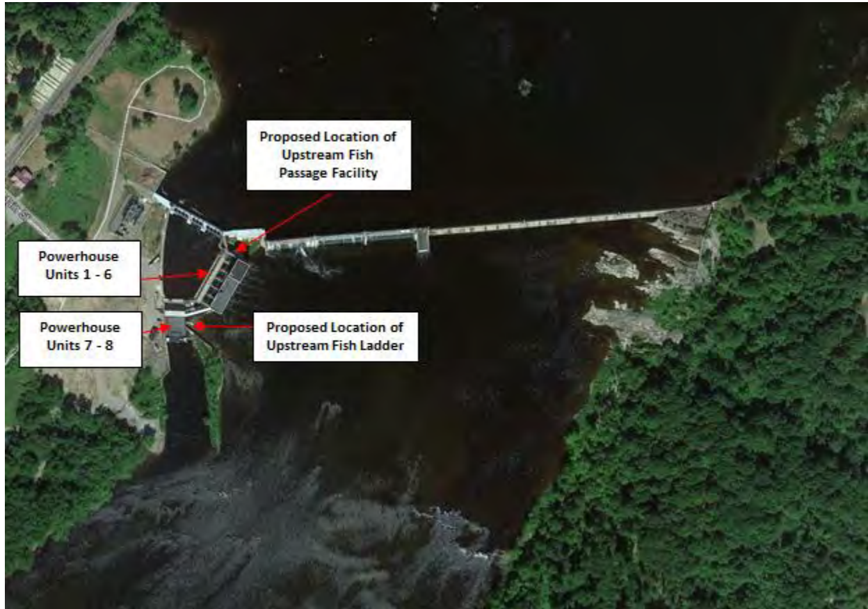
FIGURE 2. SHAWMUT DAM, POWERHOUSES, TAILRACES, PROPOSED LOCATION OF UPSTREAM FISH PASSAGE FACILITY (PHOTO YEAR: 2018)
