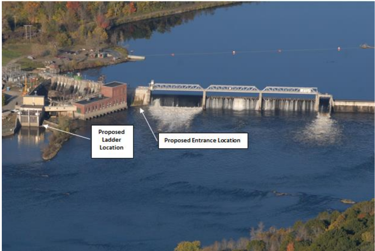
FIGURE 3. PROPOSED ENTRANCE LOCATION TO UPSTREAM FISH PASSAGE FACILITY AND FISH LADDER (PHOTO DATE: 10/12/09)
