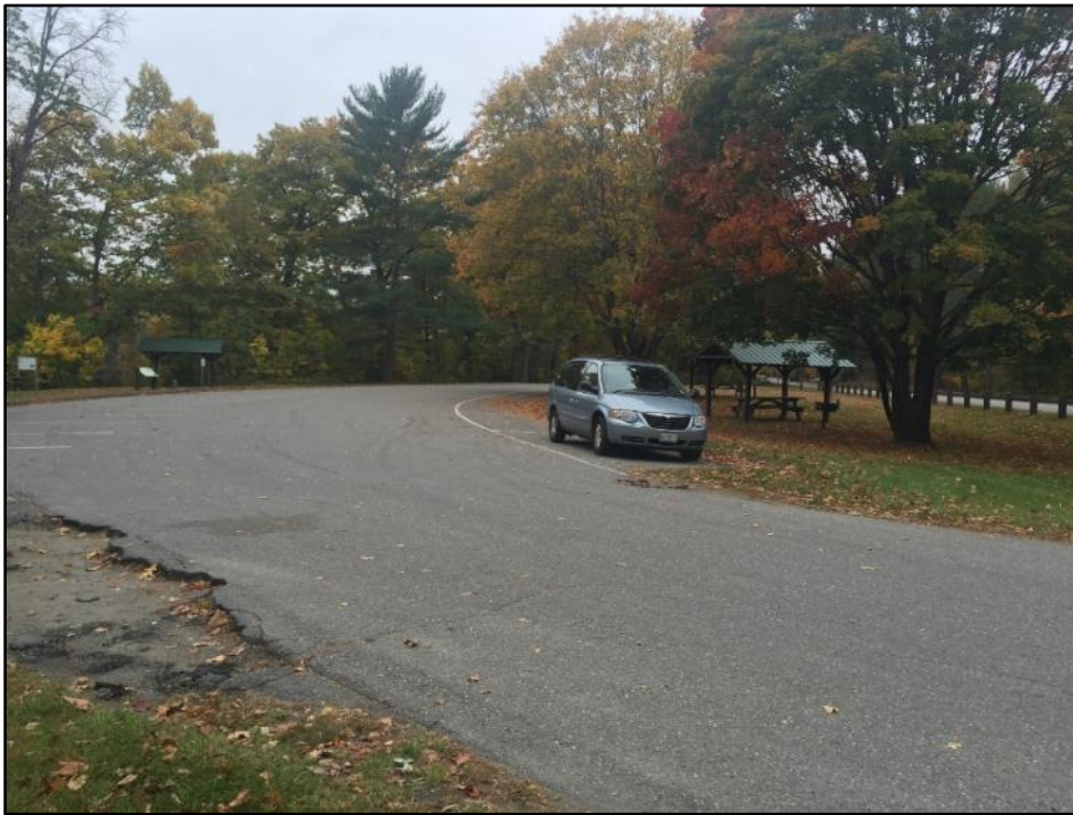
Photo 4-22 Skowhegan Route 2 Wayside Picnic Parking Area
