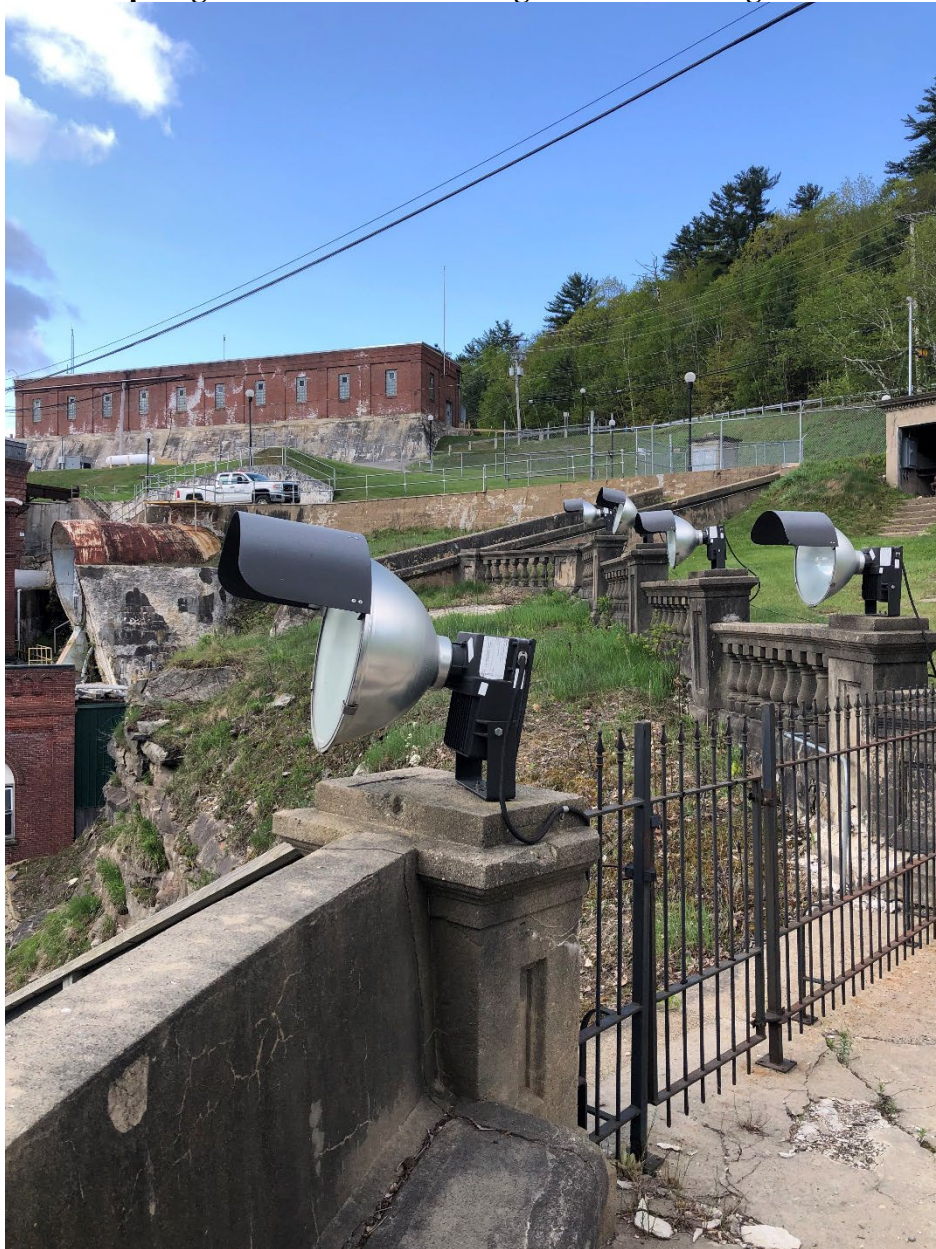
Photo 8 Spotlights and Ornate Fencing at West Viewing Area
