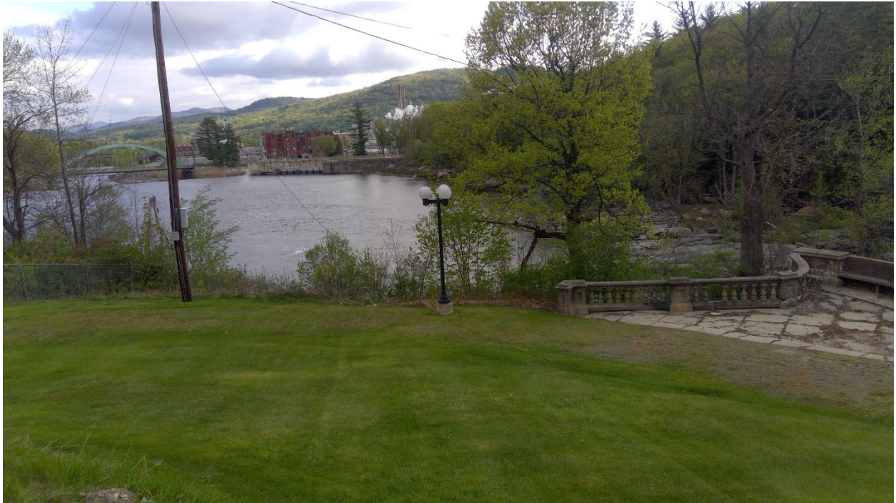
Photo 7 Exposed embankment to the north of the West Viewing Area and proposed location of ornate fencing
