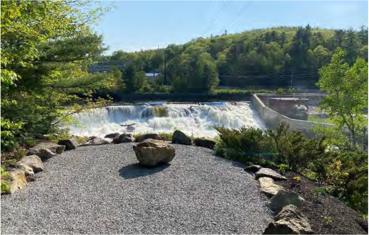
Figure 58: View of Upper Dam bypass reach from overlook (part of alternate trail).
