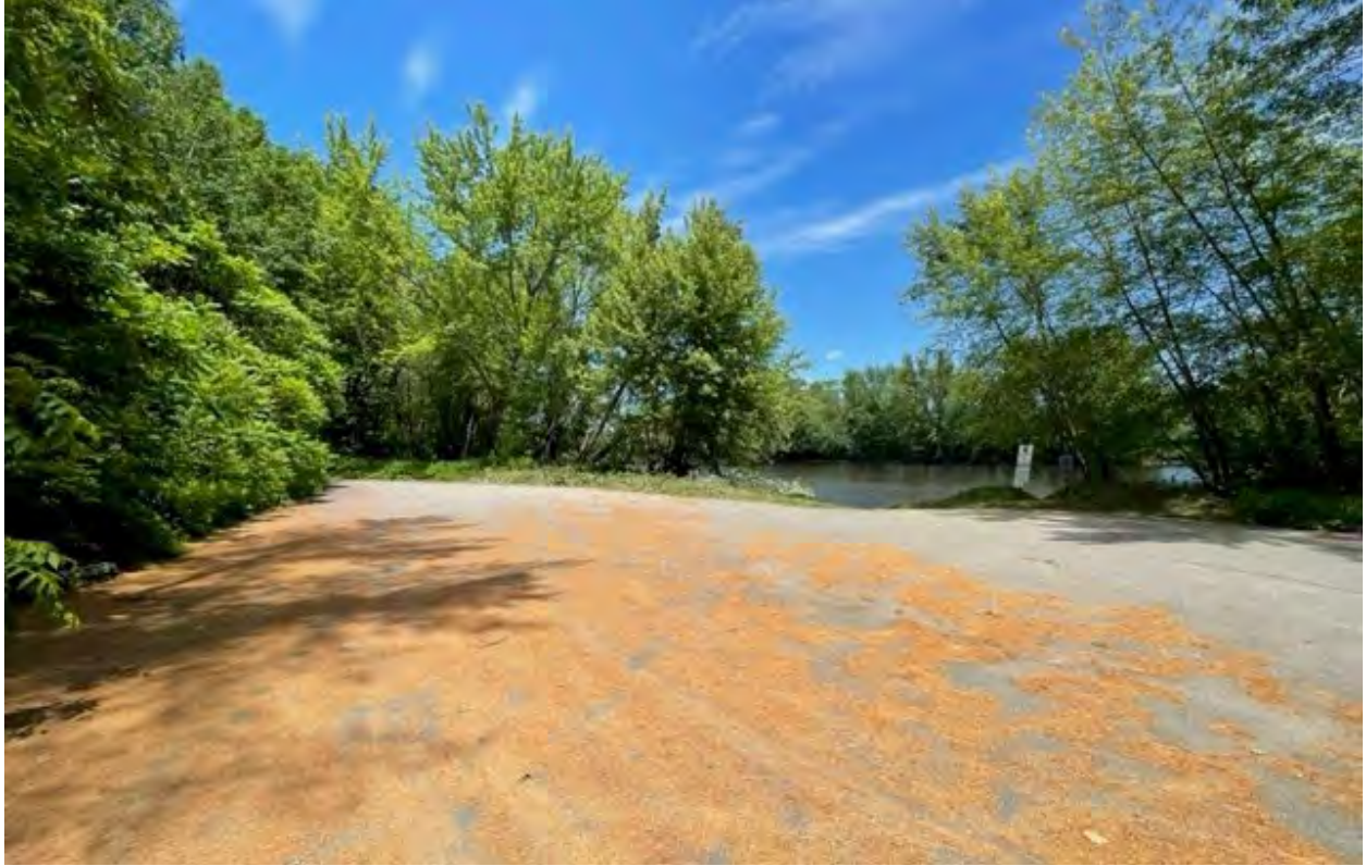
Figure 38: Paved parking area and concrete boat ramp.
