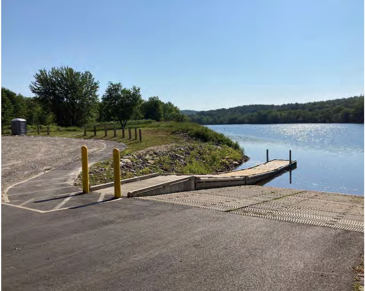
Figure 51: Concrete boat ramp (larger of the two boat ramps) with wooden dock.
