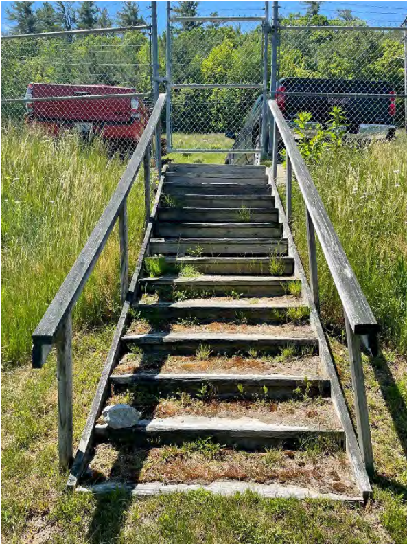
Figure 72: Stairway from West Viewing Area to existing parking area.
