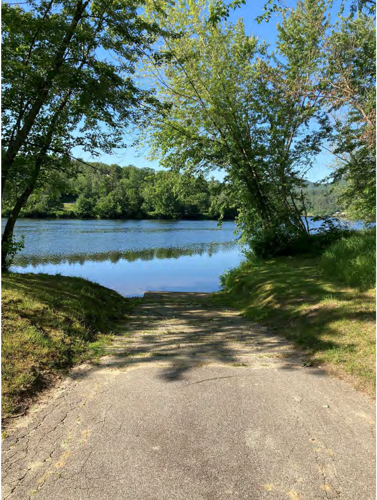
Figure 50: Concrete boat ramp (smaller of the two boat ramps).
