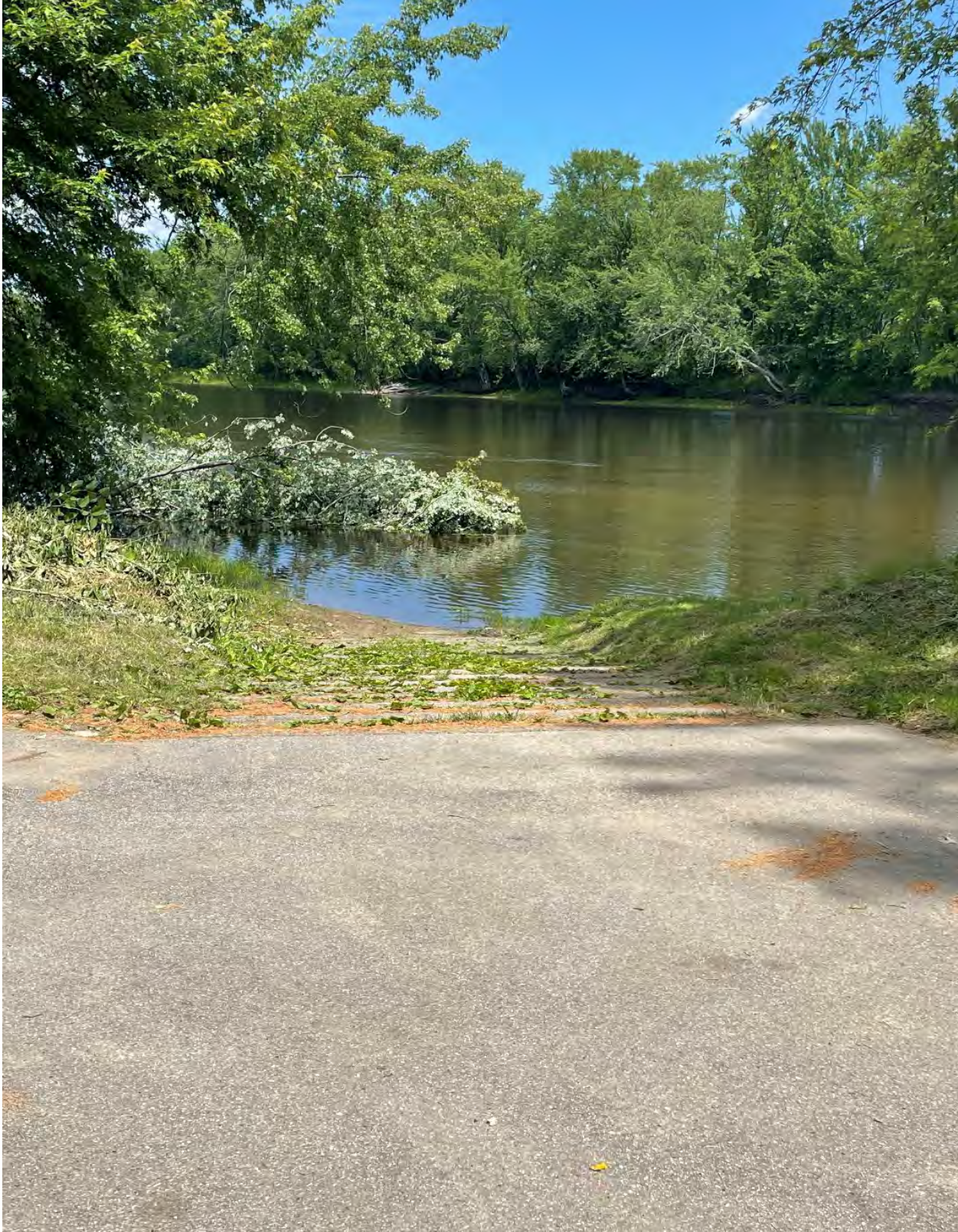
Figure 37: Paved parking area and concrete boat ramp.
