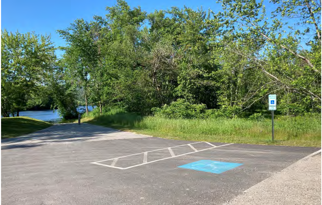
Figure 46: Paved ADA accessible parking space.
