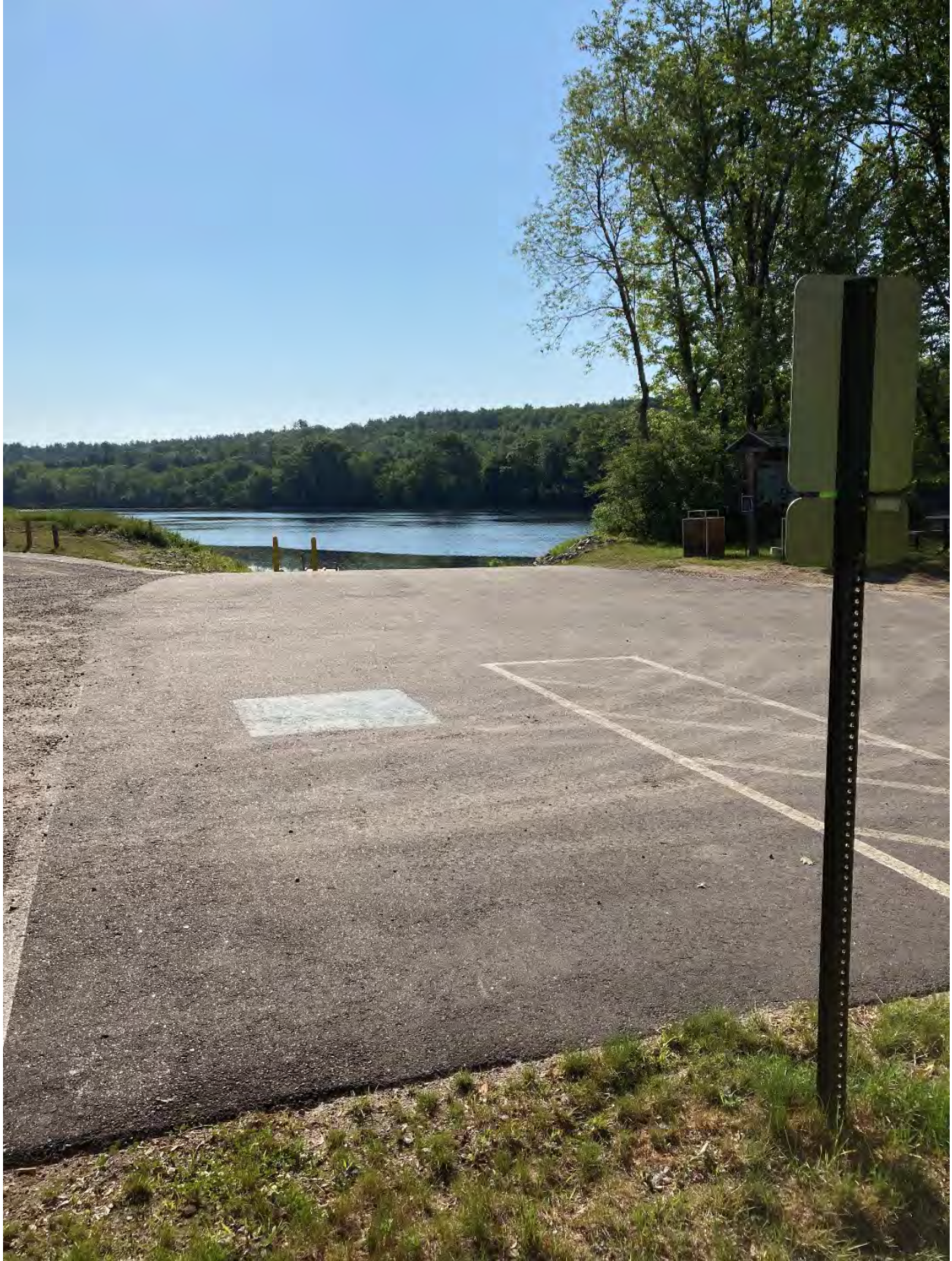
Figure 47: Paved ADA accessible parking space.
