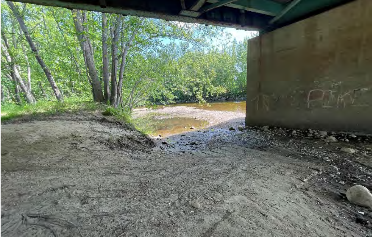
Figure 10: Concrete boat ramp under bridge.
