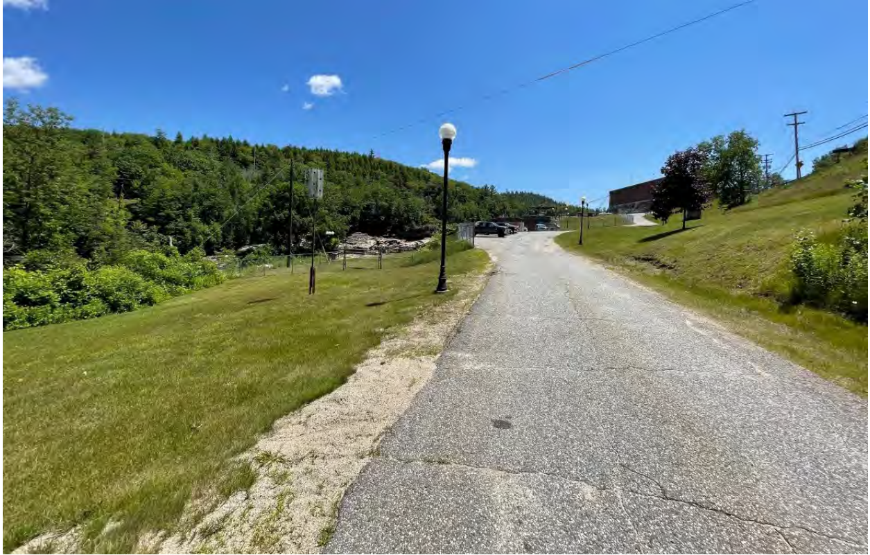
Figure 75: Paved road and walkway near West Viewing Area.
