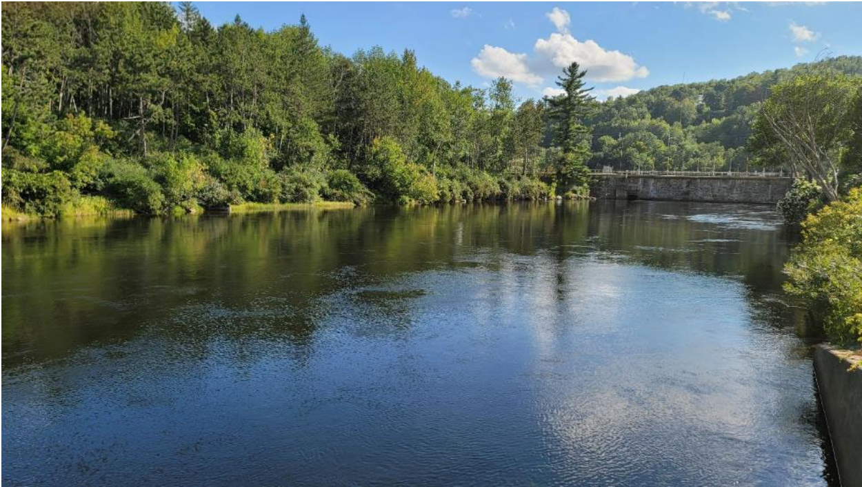
Bridge Street (canal) (Located in Middle Dam bypass reach):
