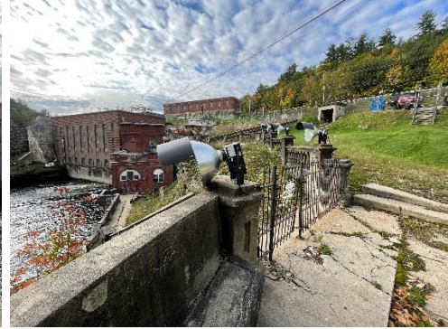
Photo at KOP facing south (upstream).
