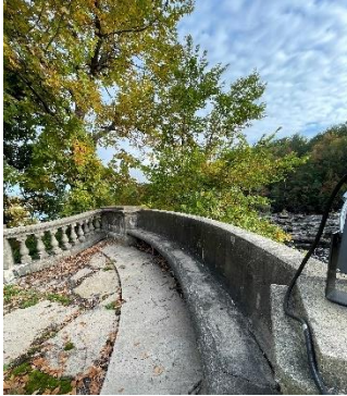
Photo at KOP facing north (downstream).
