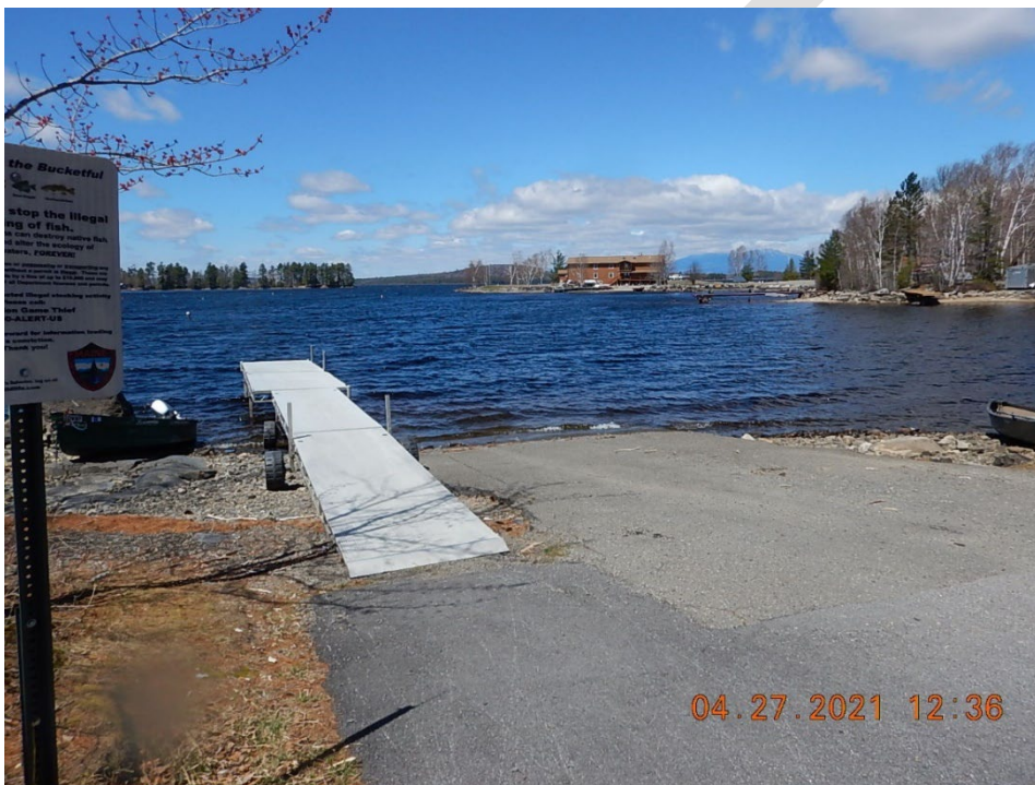
Photo 8. South Twin Lake Boat Launch and Dock.
