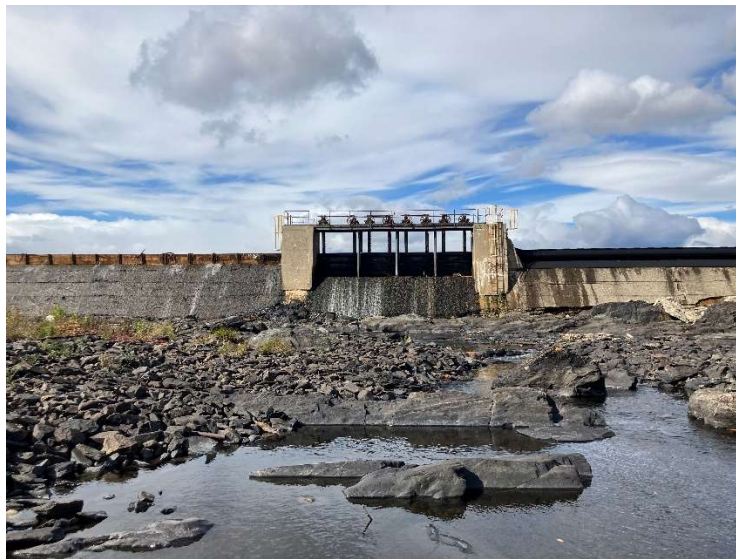
Figure 4. View upstream towards Stone Dam. Note minimum flows provided by way of leakage and spillover from wind action.
