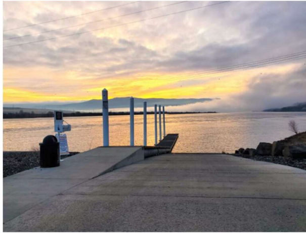
Figure 3. Washington reservoir water access facility.
