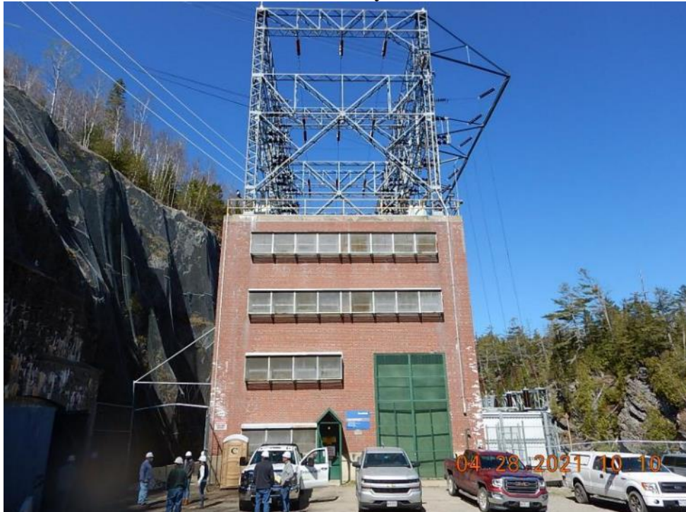
Photo 5.9-2 View of McKay Station
