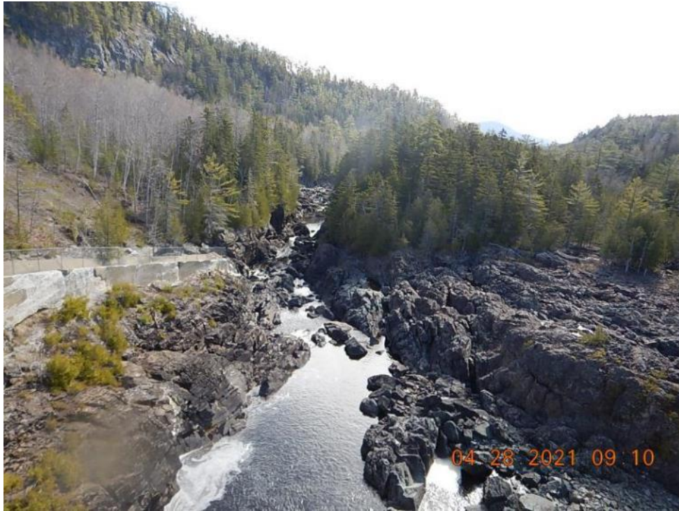
Photo 5.9-1 View of the Upper Gorge from Ripogenus Dam
