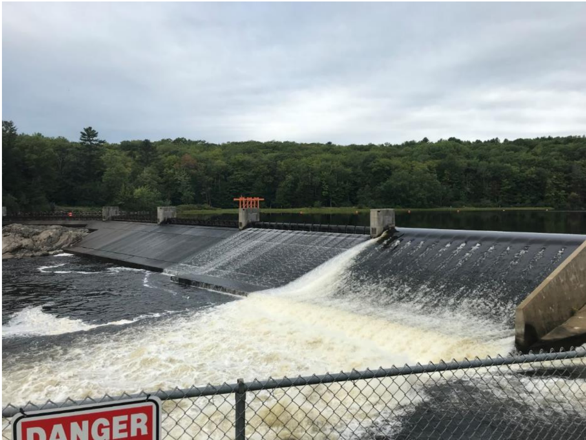
Figure 3.0-1: Flow Conditions before Stranding Evaluation Survey
