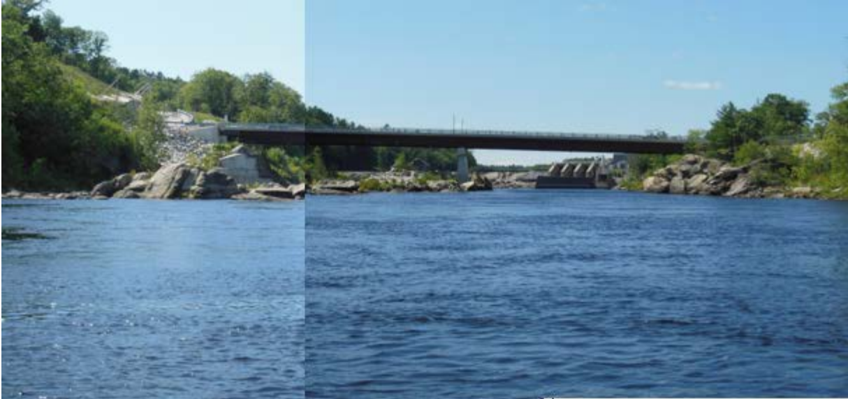
Canal St bridge at northern end of the impoundment
