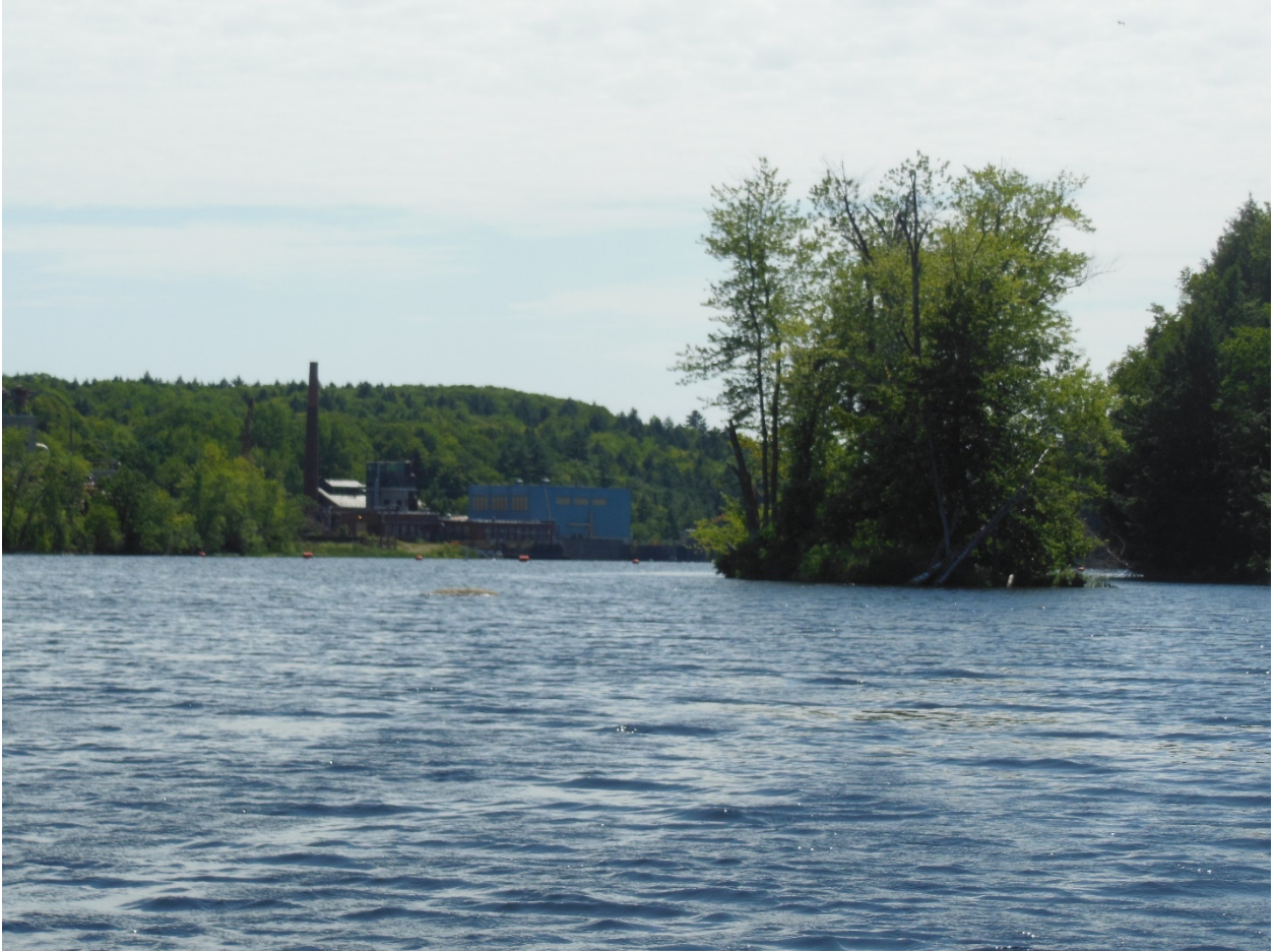
Dam related facilities southern end of Pejepscot Project, looking downstream
