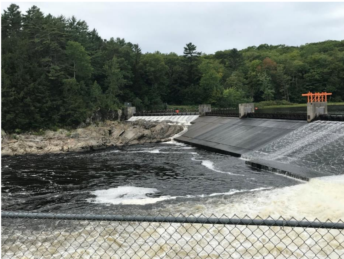
Figure 5.0-1: Initiation of Bascule Gate Operation (9:19 am)
