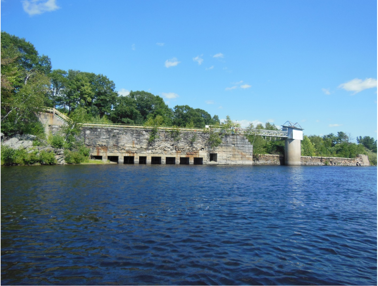
Hardened shoreline/developed areas on north-eastern end of the impoundment
