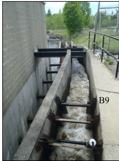
Figure 4 – Turbulent Resting Pool Downstream of Baffle “B9”
