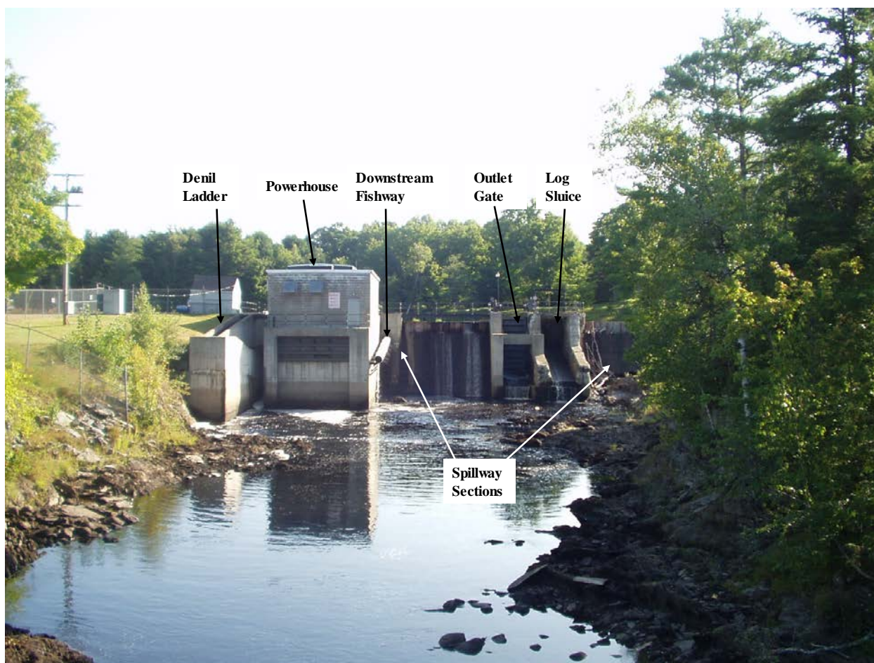
Photo 4.6 View of powerhouse, dam, fishways, and spillway.
