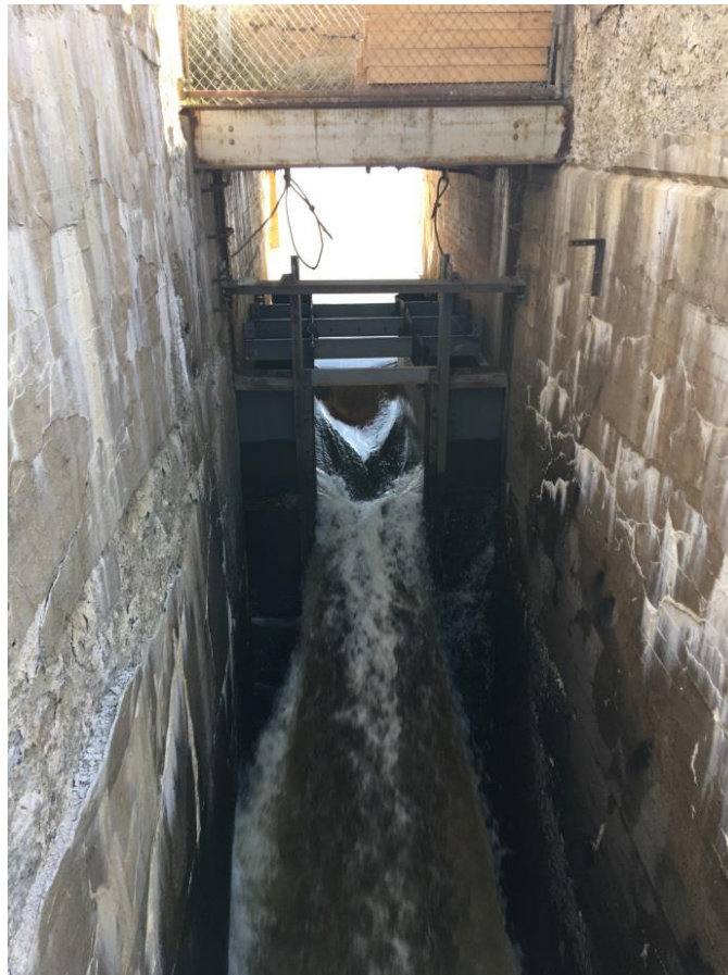
FIGURE 6 GRAHAM LAKE DAM FISH PASSAGE WEIR
