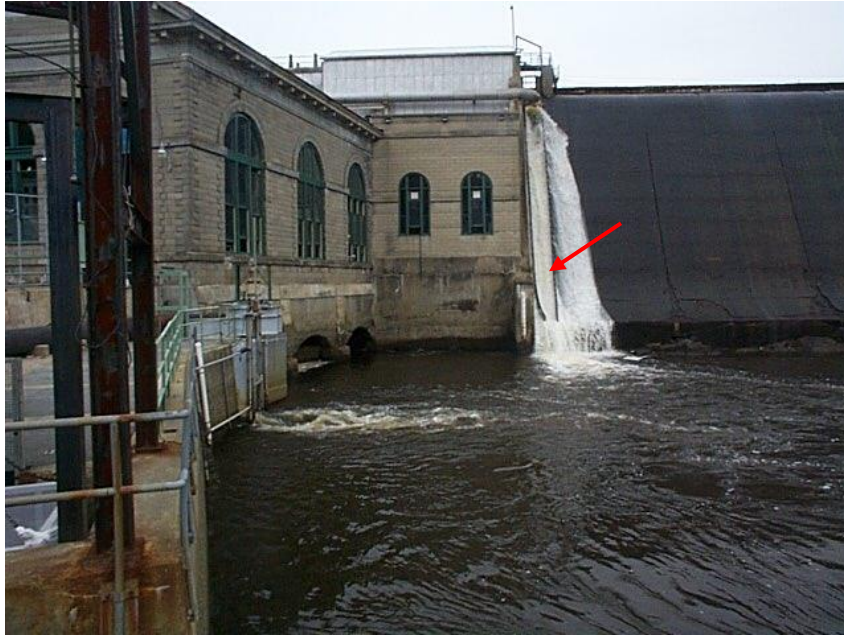
FIGURE 5 VIEW OF DISCHARGE FROM DOWNSTREAM FISH PASSAGE PIPE AND SURFACE WEIR AT THE ELLSWORTH DAM
