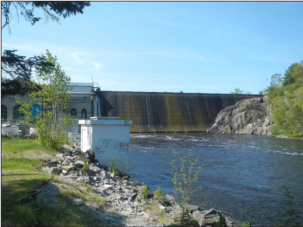
Photo A-1: Ellsworth Dam Spillway and Powerhouse
