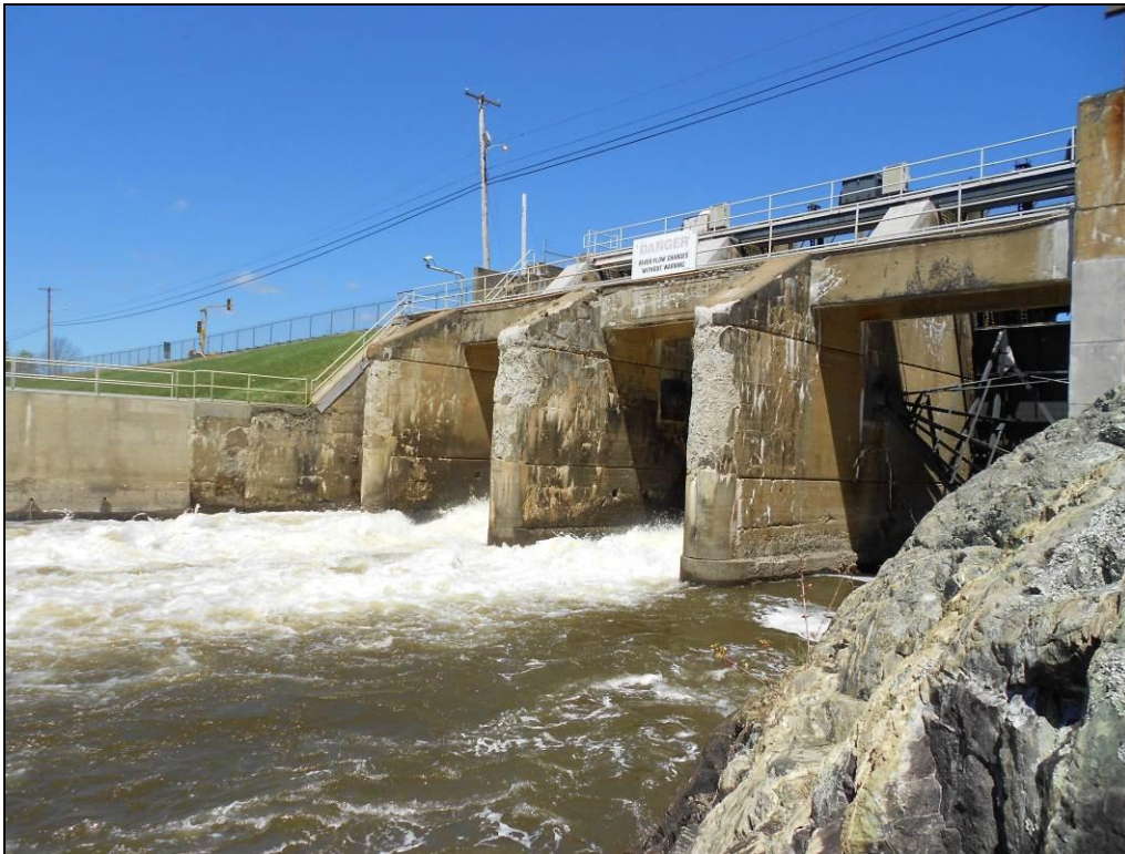
Photo A-4: Graham Lake Dam Gate Structure
