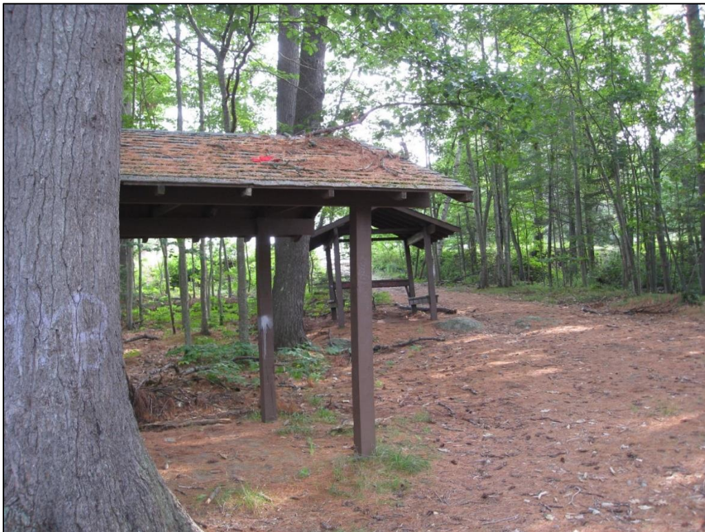
Photo 4-13: Day-use area shelters and path
