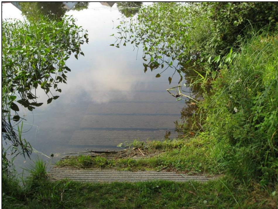
Photo 4-3: Lake Leonard carry-in boat launch ramp
