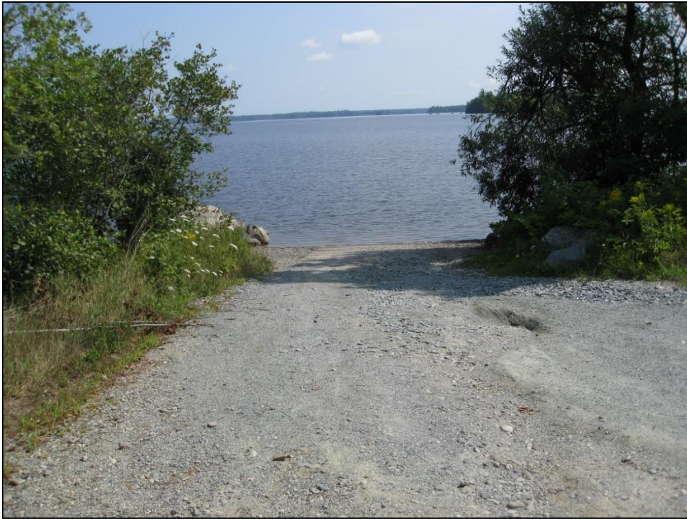
Photo 4-6: Graham Lake boat launch ramp
