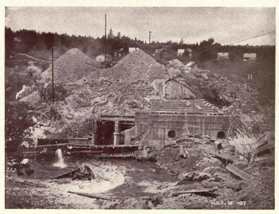
HE finished work is now to the 42.5 level but all of the concrete is not in the dam itself. The power house foundation piers are progressing and two of them are shown completed and on the third the forms are ready to be filled.
