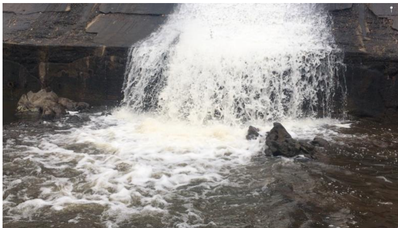
^Toe of the Ellsworth dam, showing exposed rocks and ledge
