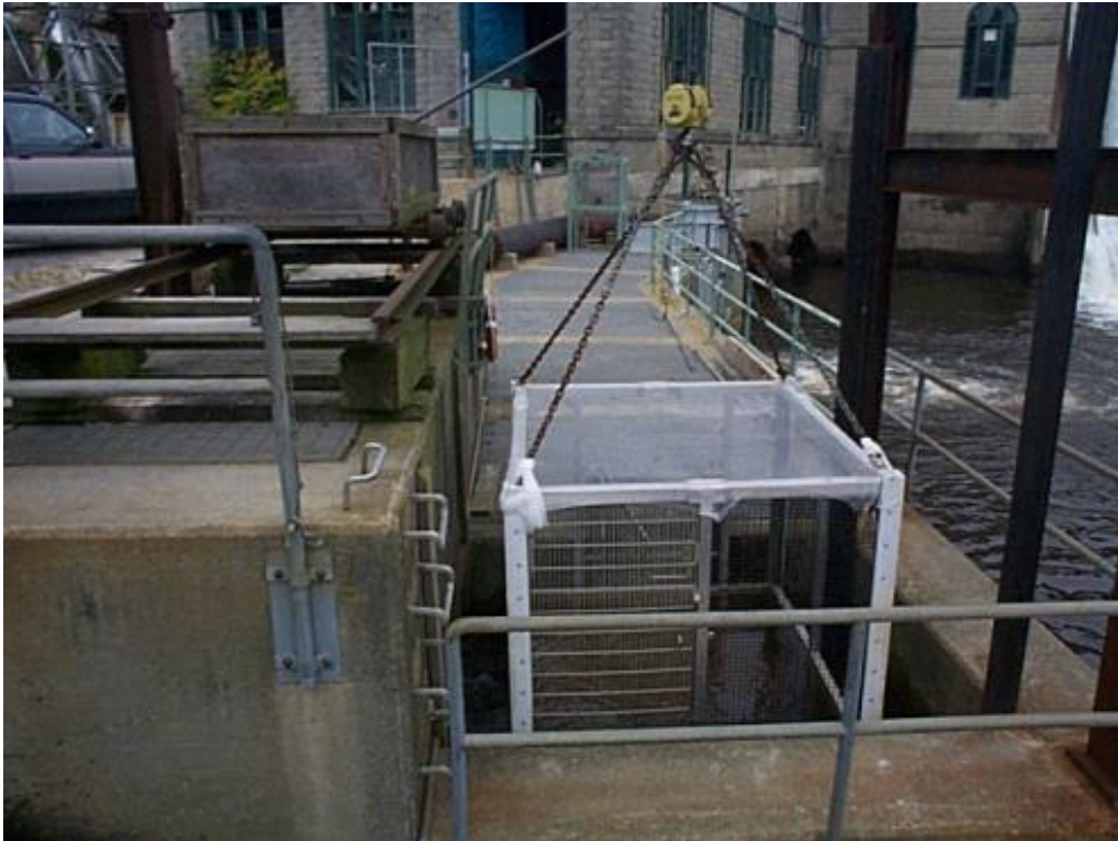
FIGURE 6 VIEW OF FISHWAY HOPPER IN OPERATION USED FOR TRANSFERRING FISH TO THE HOLDING TANK AT THE ELLSWORTH DAM
