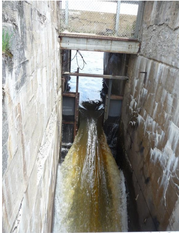
FIGURE 6 GRAHAM LAKE DAM FISH PASSAGE WEIR
