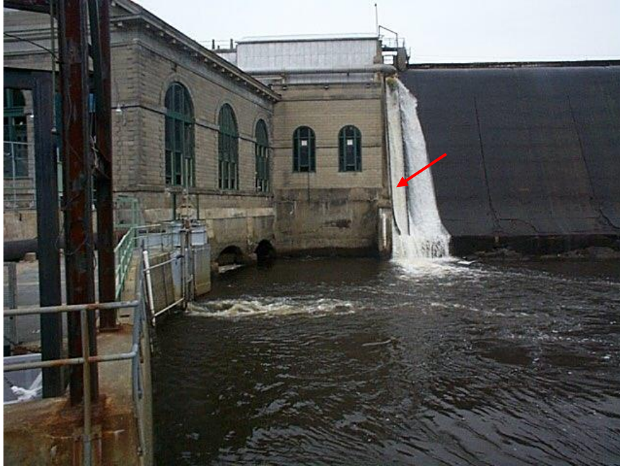
FIGURE 5 VIEW OF DISCHARGE FROM DOWNSTREAM FISH PASSAGE PIPE AND SURFACE WEIR AT THE ELLSWORTH DAM
