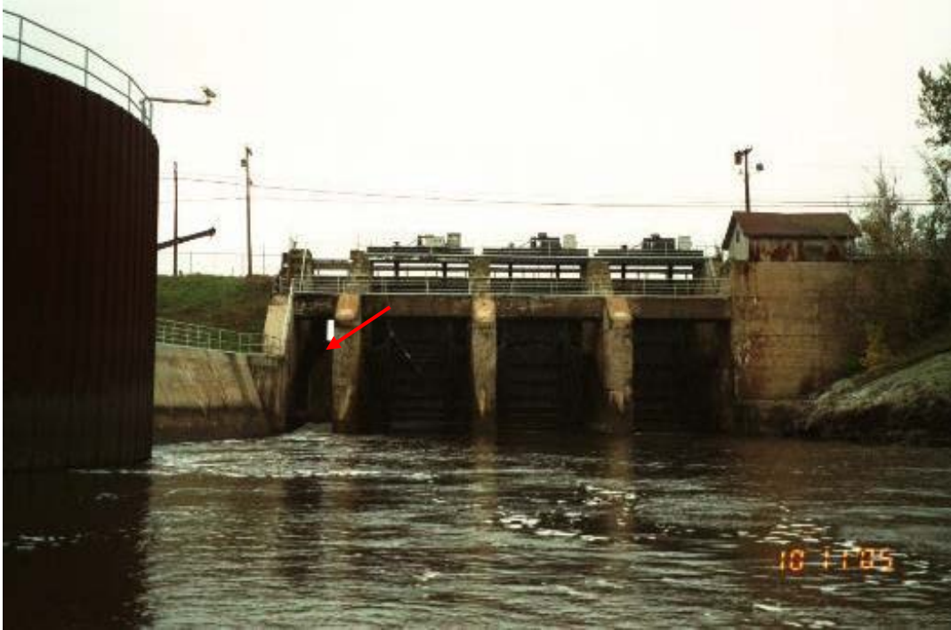
FIGURE 5 VIEW OF DOWNSTREAM SIDE OF THE GRAHAM LAKE DAM, WHERE THE DOWNSTREAM BYPASS IS INTEGRAL WITH THE RELEASE GATES (ARROW)
