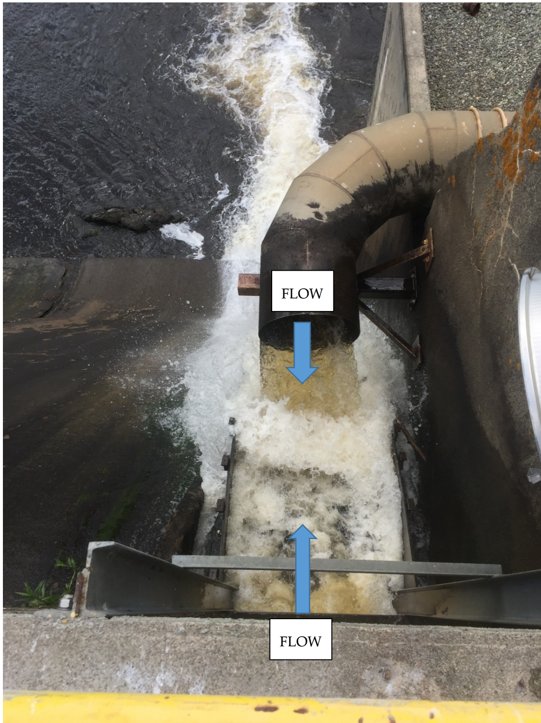
Figure 5.6. Zone of shear along the downstream bypass system at Ellsworth Dam. The flow from the third weir flows is nearly perpendicular to the direction of the flow from the first two weirs.
