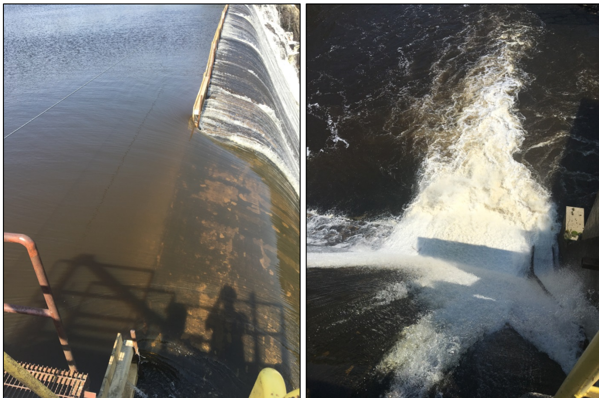
Figure 1-2. Approximately 20 feet of opened flashboards (three sections) at the Ellsworth Dam to provide additional passage opportunity for tagged Atlantic salmon smolts, spring 2017.
