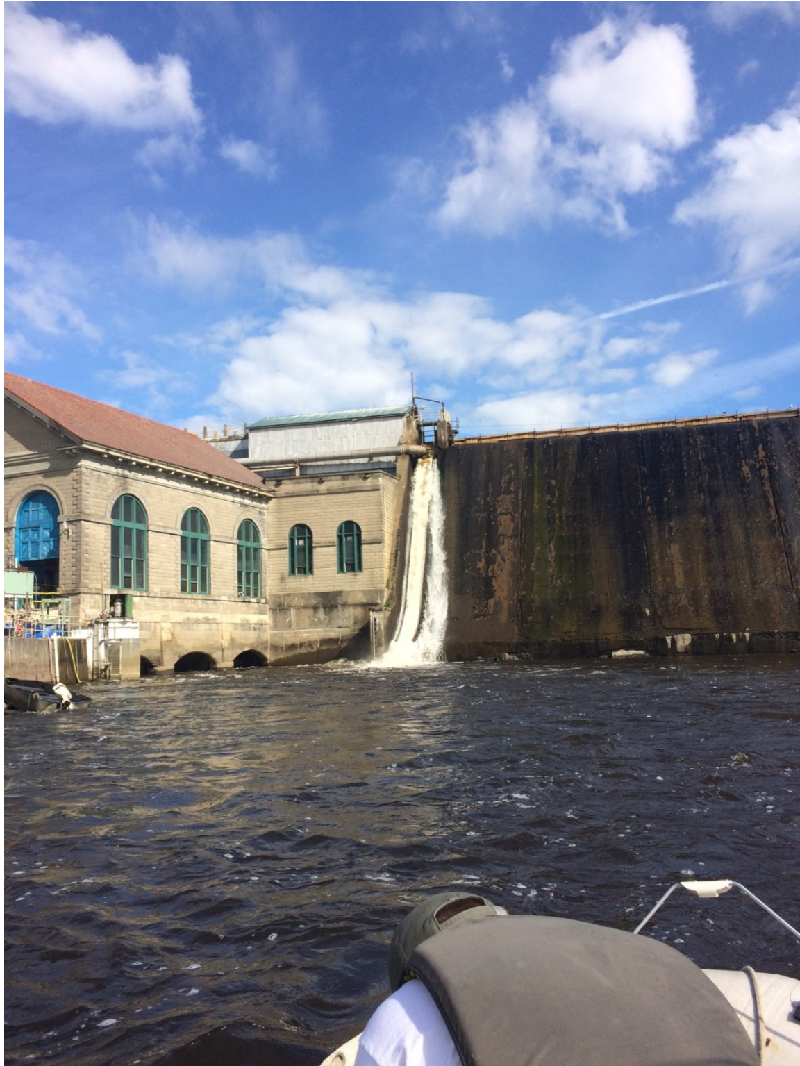
Figure 1.1. Ellsworth Dam with the powerhouse shown at left. Turbine Unit 1 discharges perpendicular to the face of the dam and turbine Units 2-4 discharge parallel to the dam face. The downstream bypass sluice can be seen directly to the right of the powerhouse.
