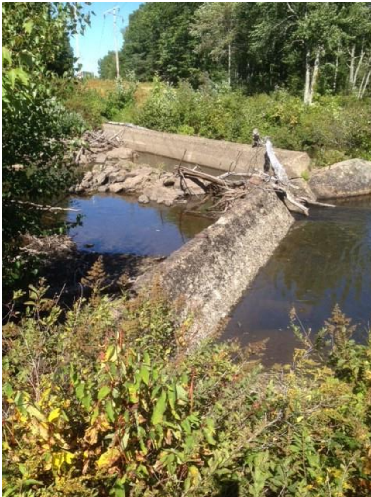
Photo 3 – Branch Lake Stream dam
