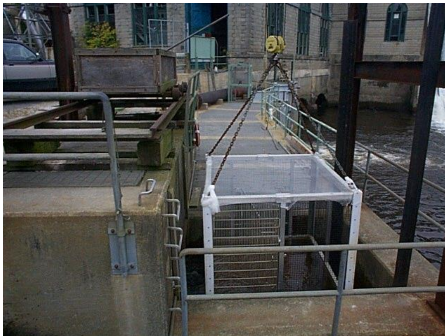
FIGURE 3 VIEW OF FISHWAY LIFT IN OPERATION USED FOR TRANSFERRING FISH TO THE HOLDING TANK AT THE ELLSWORTH DAM
