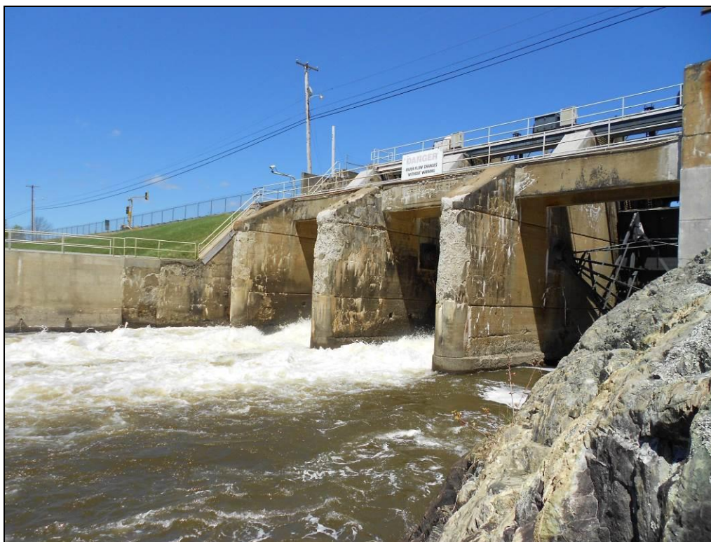
Photo A-4: Graham Lake Dam Gate Structure
