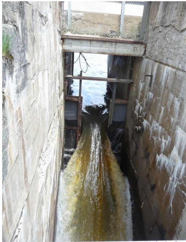
FIGURE 6 GRAHAM LAKE DAM FISH PASSAGE WEIR
