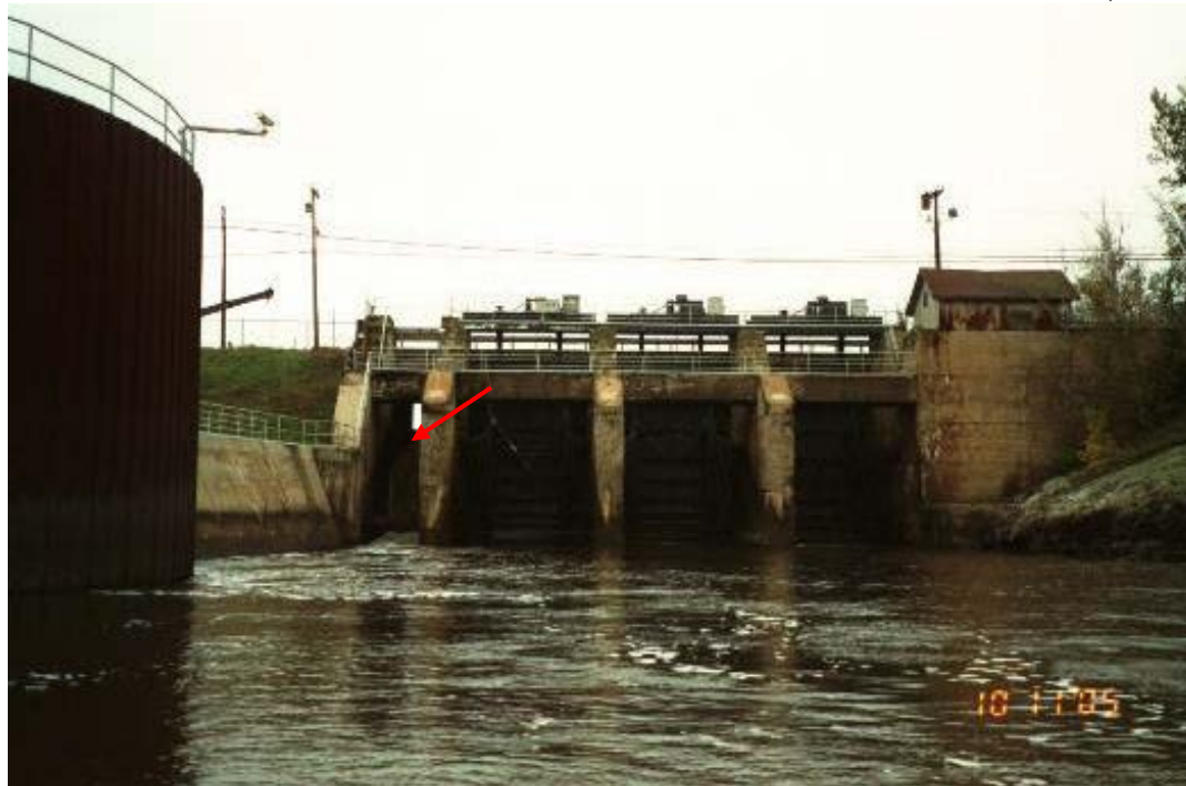
FIGURE 5 VIEW OF DOWNSTREAM SIDE OF THE GRAHAM LAKE DAM, WHERE THE DOWNSTREAM BYPASS IS INTEGRAL WITH THE RELEASE GATES (ARROW)
