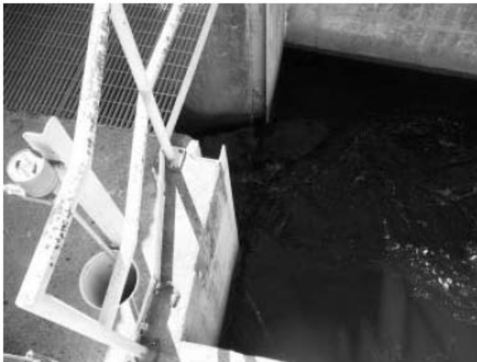
FIGURE 4 VIEW OF DISCHARGE FROM DOWNSTREAM FISH PASSAGE PIPE (ARROW) AT THE ELLSWORTH DAM
