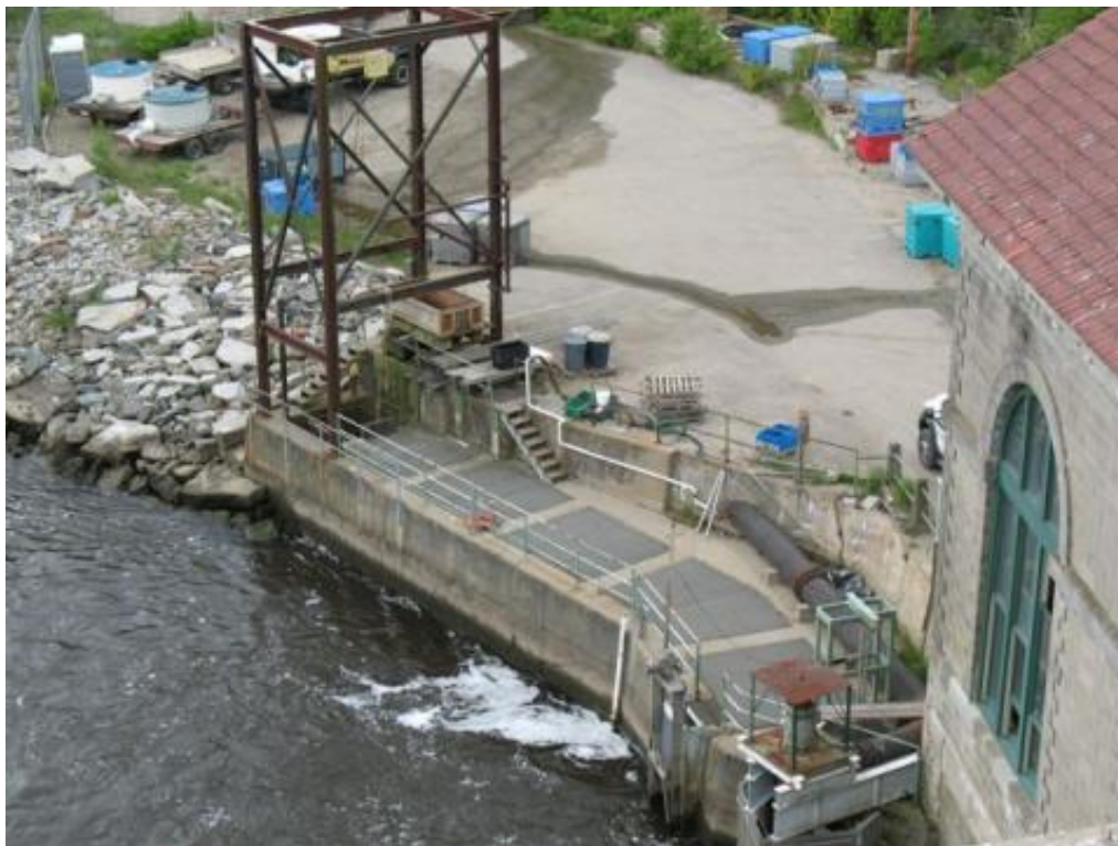
FIGURE 7 OVERVIEW OF FISHWAY TRAP AND TRANSFER FACILITY AT THE ELLSWORTH POWERHOUSE TAILRACE
