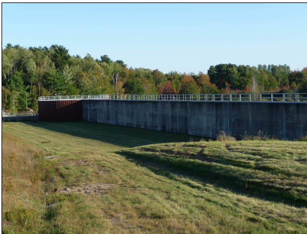
Photo A-5: Graham Lake Dam Flood Control Structure
