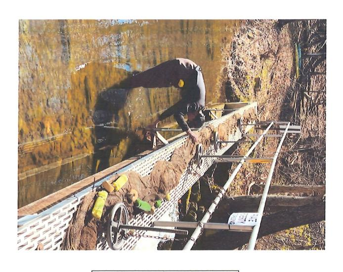
This gentleman is standing in the water prior to the Coffin Dam. You can see that the water level is not even up to his knees. The Coffin Dam only controls 12 inches of water from 263 to 264 feet. The 4 hand wheels used to change the gate height are all visible. The seine net is lowered while the 7 Lakes Alliance Dive Team is pulling Curly-leaf Pondweed so that plant fragments are not carried over the dam thus spreading this noxious, highly invasive, aquatic plant.
