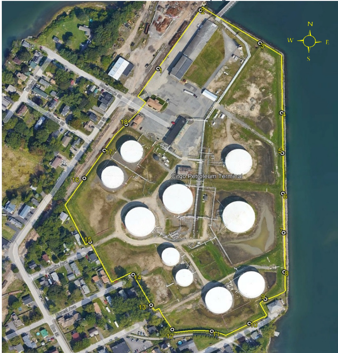
Aerial View of the CITGO South Portland Terminal Fenceline Sampling Locations
