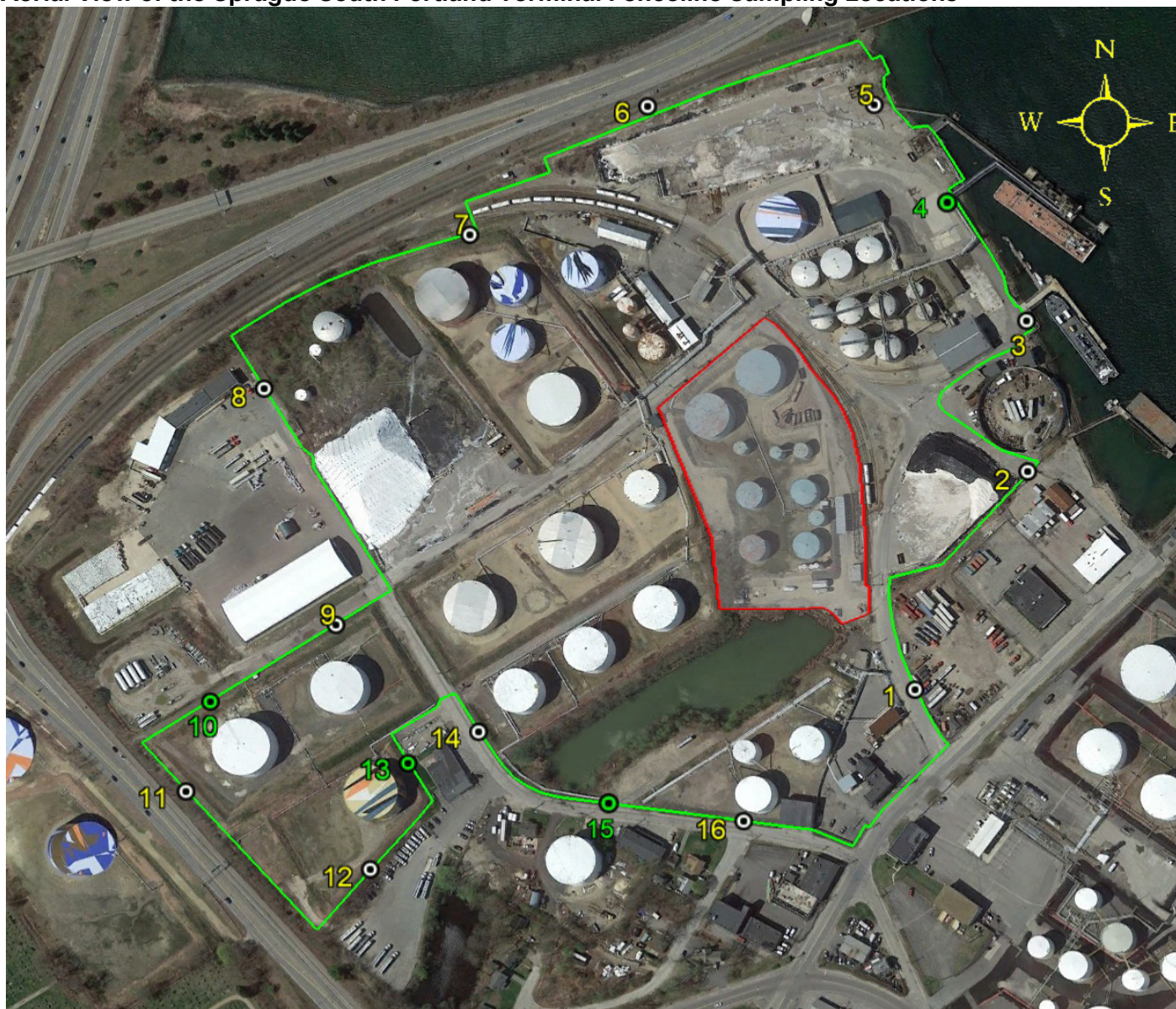
Aerial View of the Sprague South Portland Terminal Fenceline Sampling Locations
