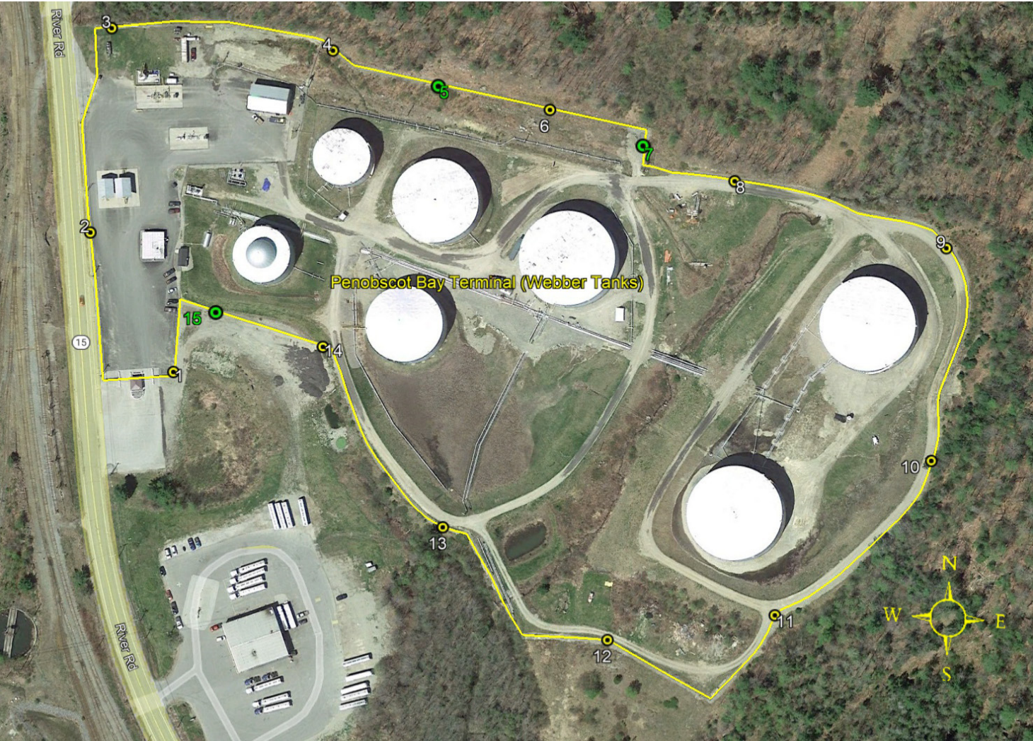
Aerial View of the Fenceline Monitor Locations for the Penobscot Bay Terminal
