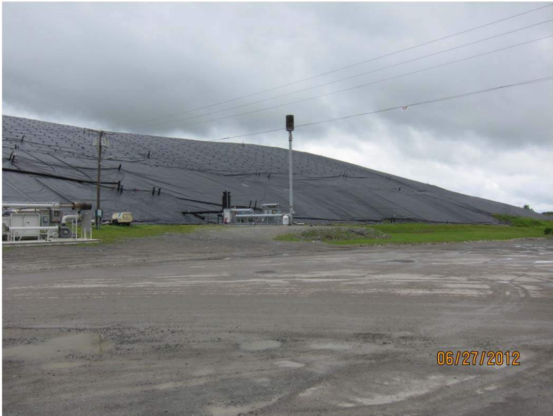
north side, looking south at northern slopes of Cell 3 (left) and Cell 1&2 (right)
