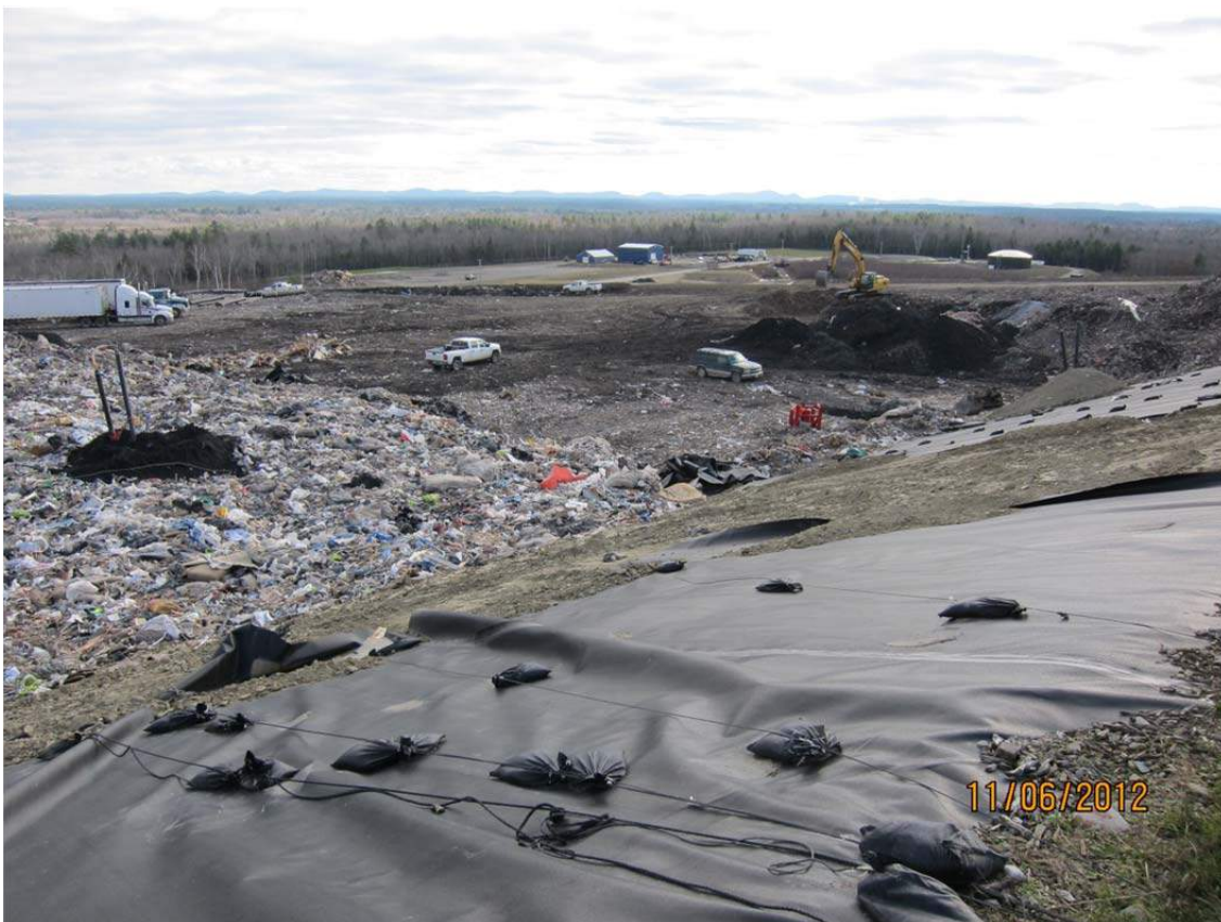
Cell 3 - eastern interim slope (with active cell to left) looking south
