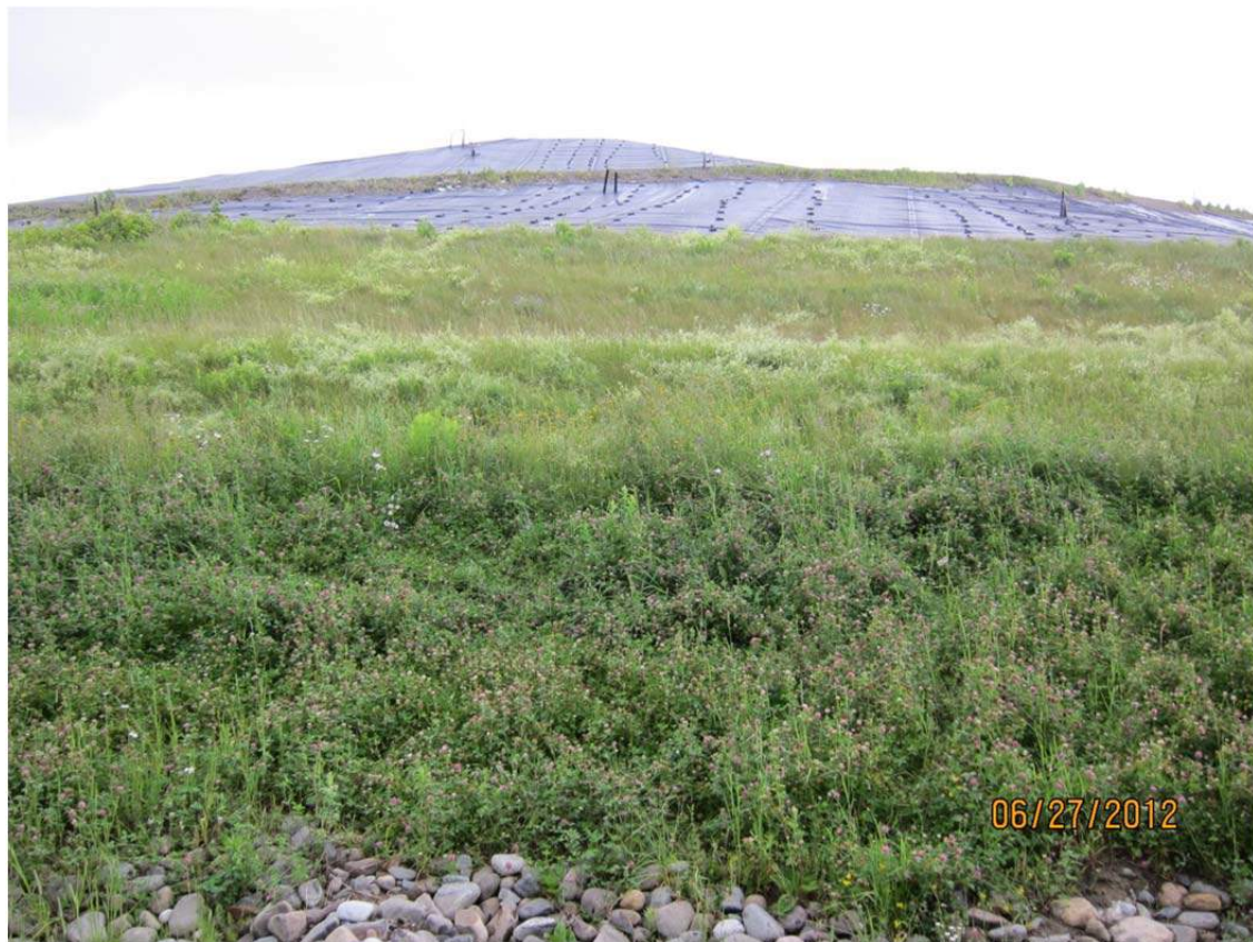
western side, looking northeast at western slope of Cell 1&2
