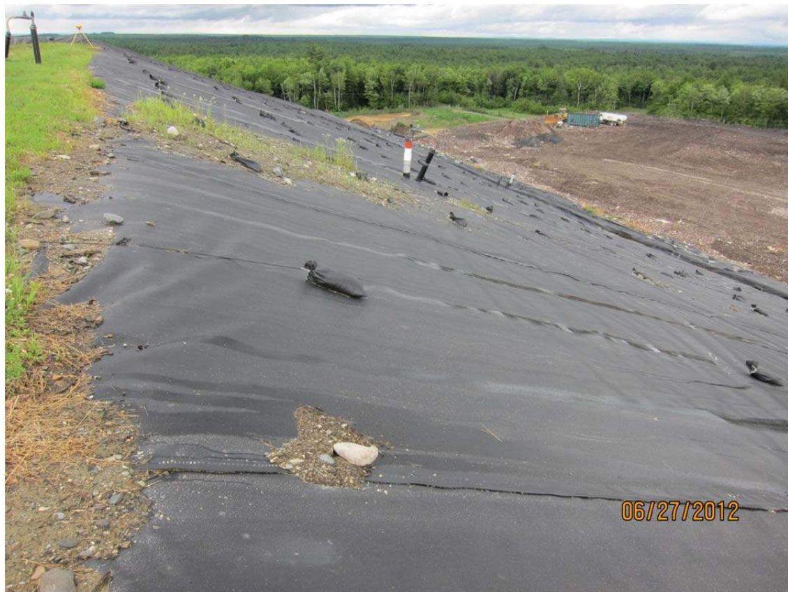
Cell 3 - eastern interim slope looking north
