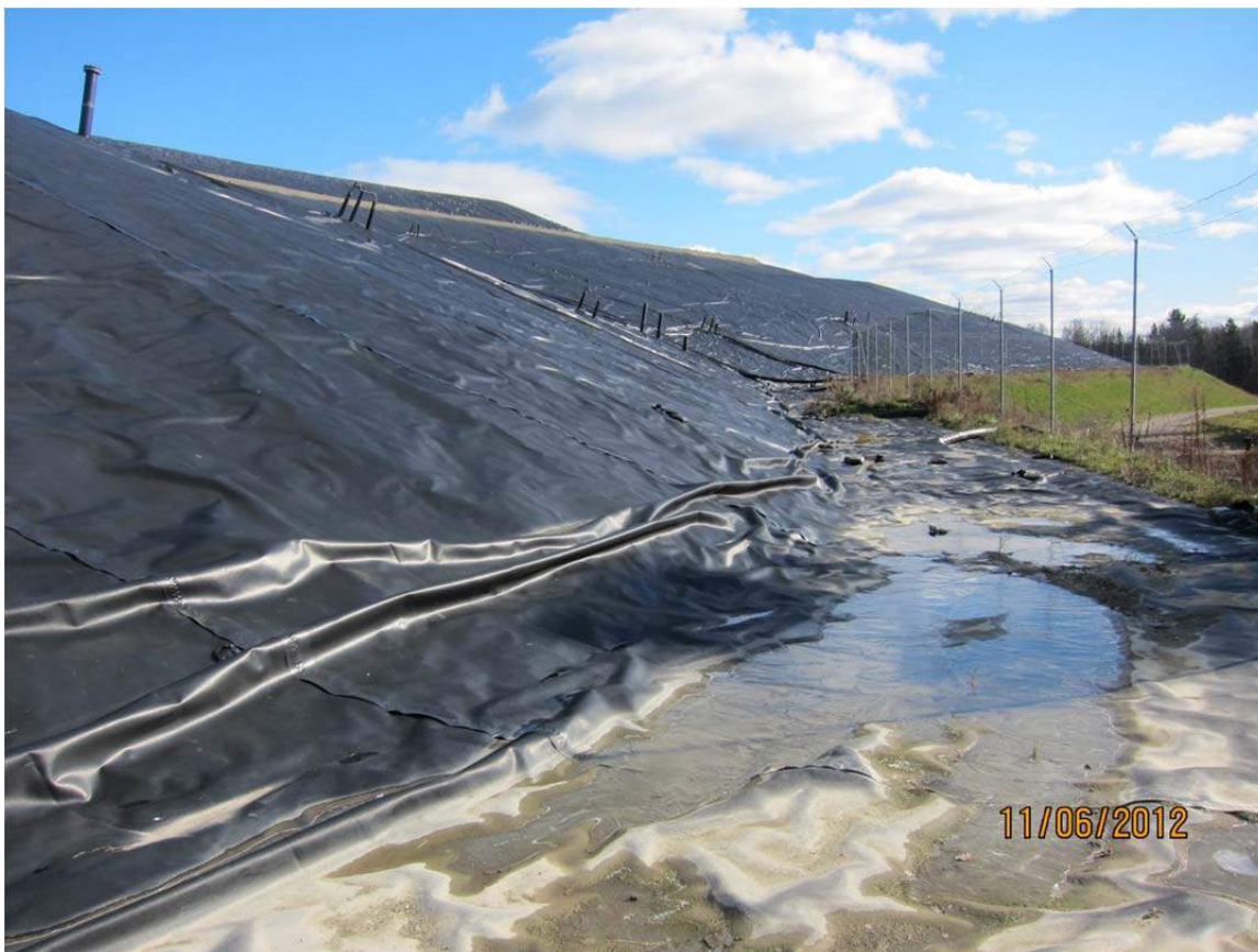
western side, looking southeast along western slope of Cell 4
