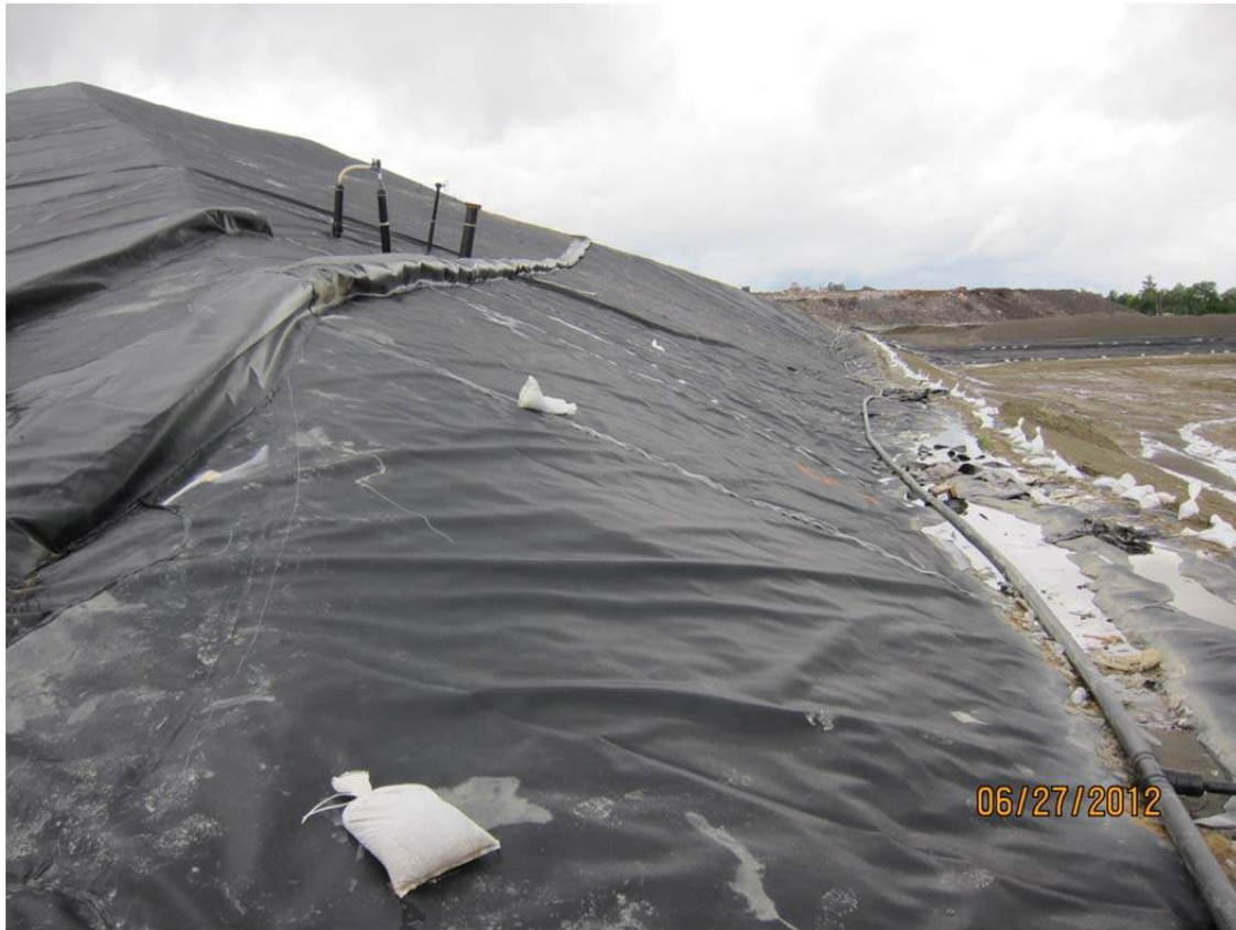
SE corner looking north along eastern slope of Cell 4
