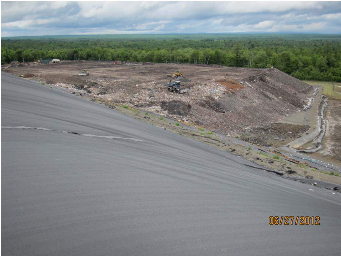
eastern interim slope, Cell 3, looking northeast towards active cell
