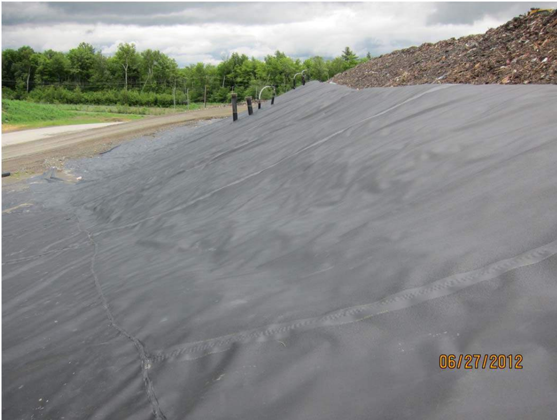
NE corner looking east at northern slope of Cell 3B
