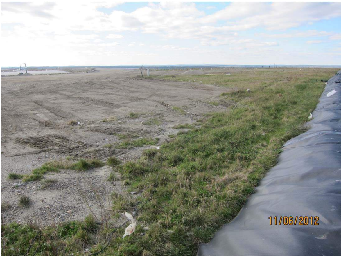
northeast corner: top of Cell 3 looking southwest
