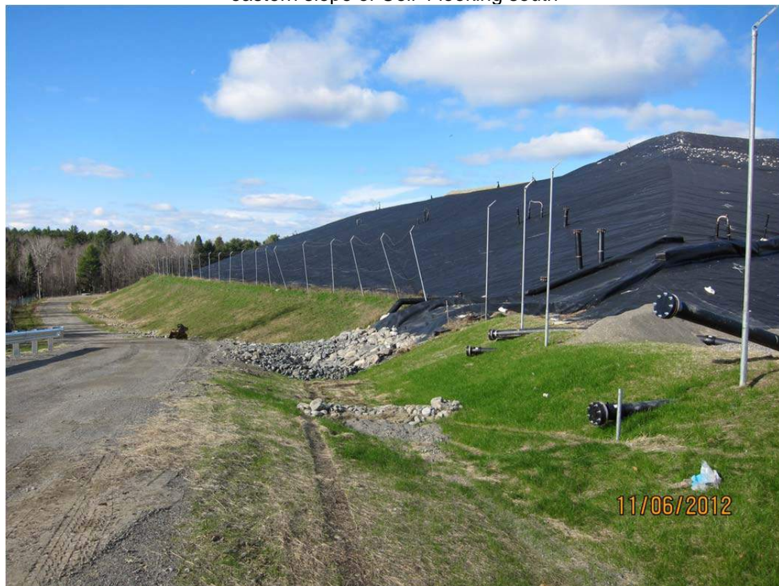
SE corner of Cell 4 looking west along southern slope of Cell 4
