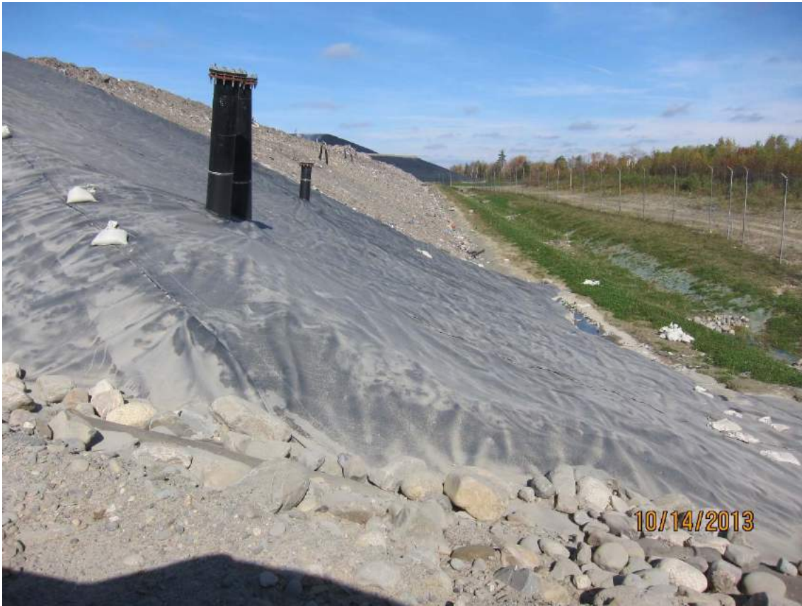
SE corner of Cell 8 looking northerly along active Cell 8
