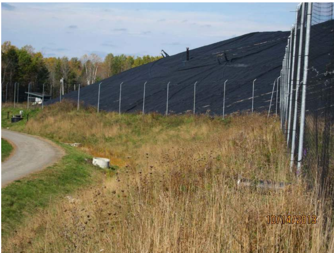
SW corner of Cell 4/6 looking southeasterly towards lower slope of Cell 4/5
