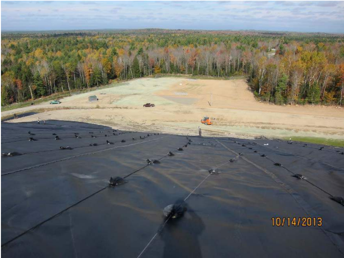
crest of northwest corner of Cell 1/2 looking down onto northwestern sed pond
