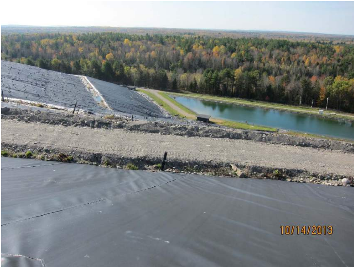
bottom portion of western slope of Cell 4/5
