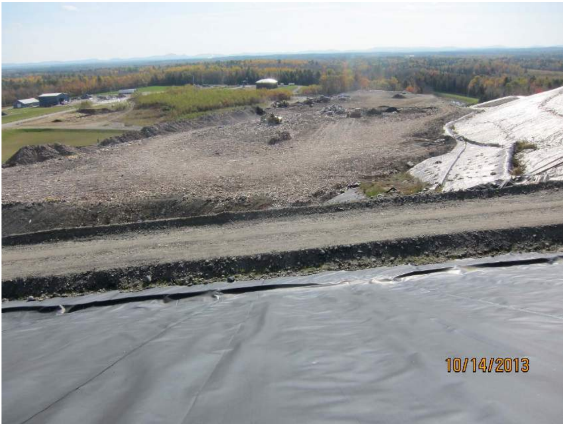
on the top of southern slope of Cell 7, looking south
