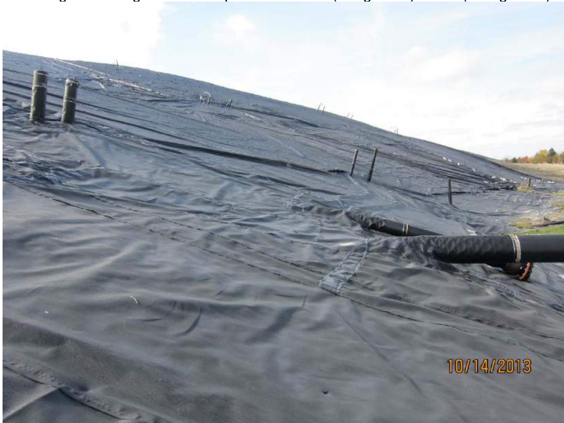
northern slope looking west along transition slope between Cell 3 and Cell 1 & 2
