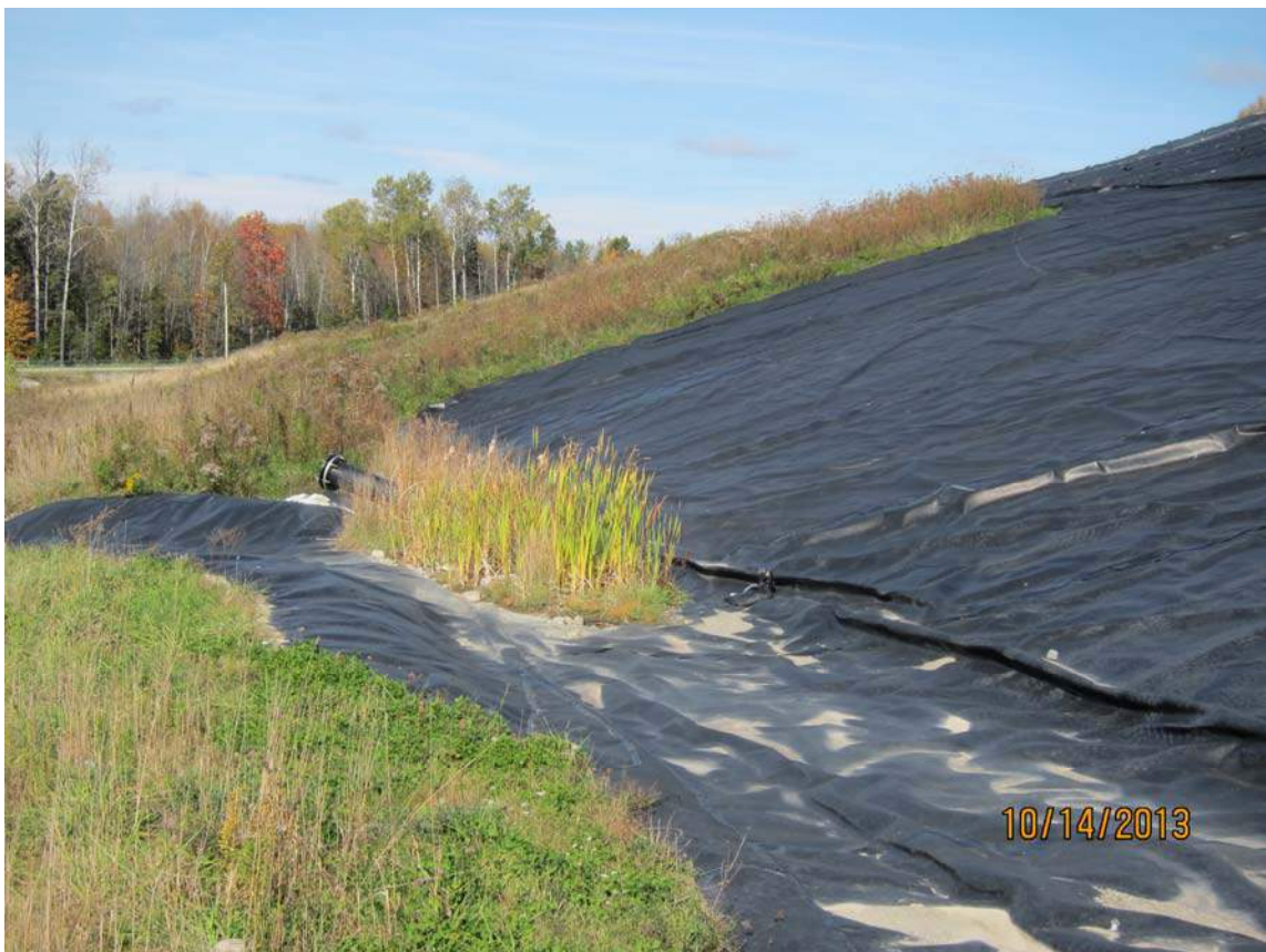
SW corner of Cell 4 looking northwesterly along lower SW slope of Cell 1/2
