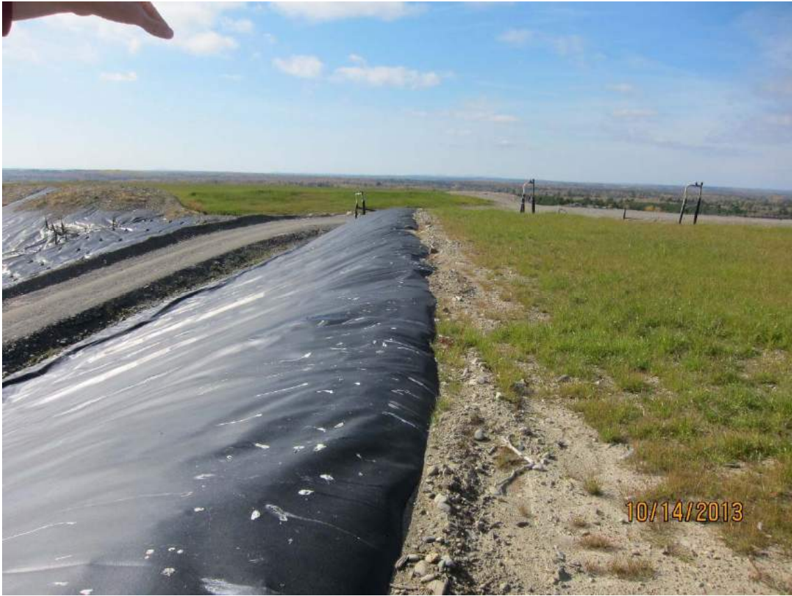
top of Cell 7 southern slope, looking southwest on landfill top of Cell 3/4 (fore) & Cell 4/5 (aft)
