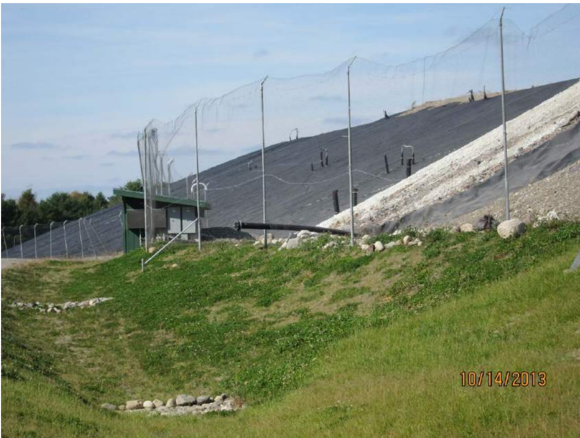
SW corner of Cell 8 looking southwesterly along lower slope of Cell 4/6
