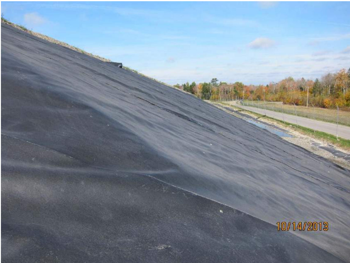
SE corner of Cell 7 looking northwesterly along the bottom of NE slope of Cell 7
