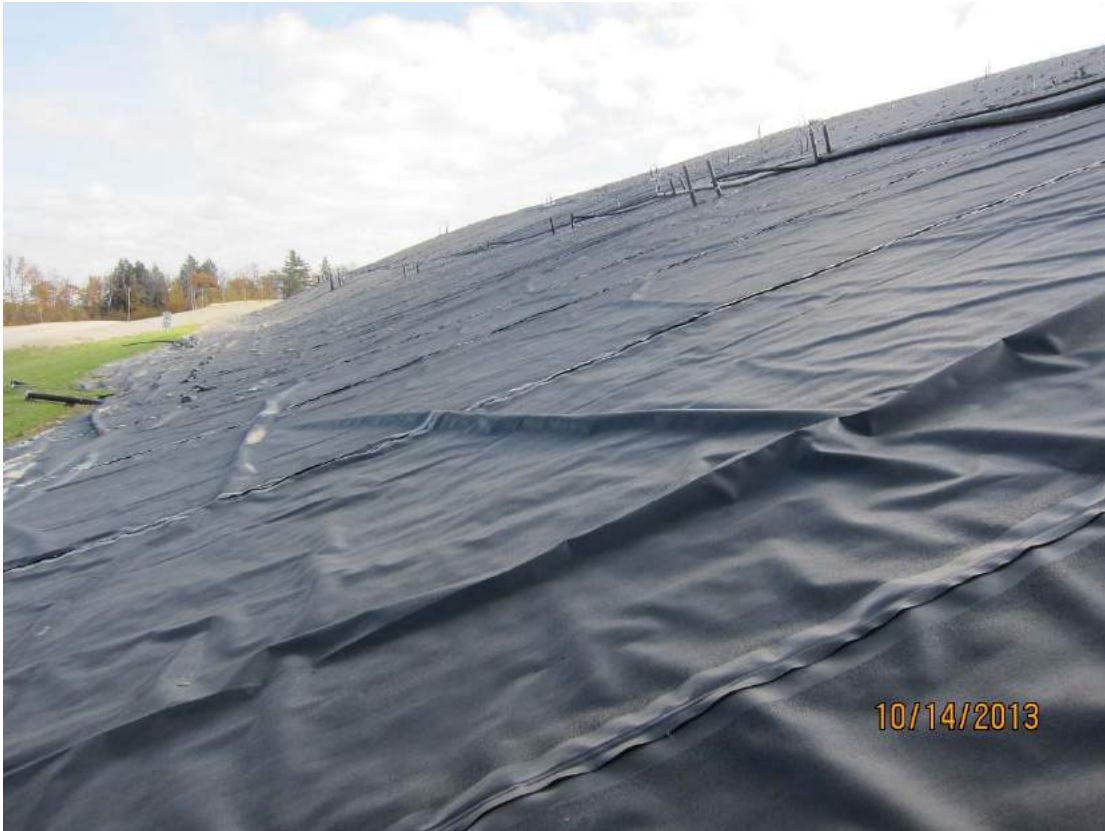
looking east along northern slope of Cell 1 & 2 (foreground) Cell 3 (background)
