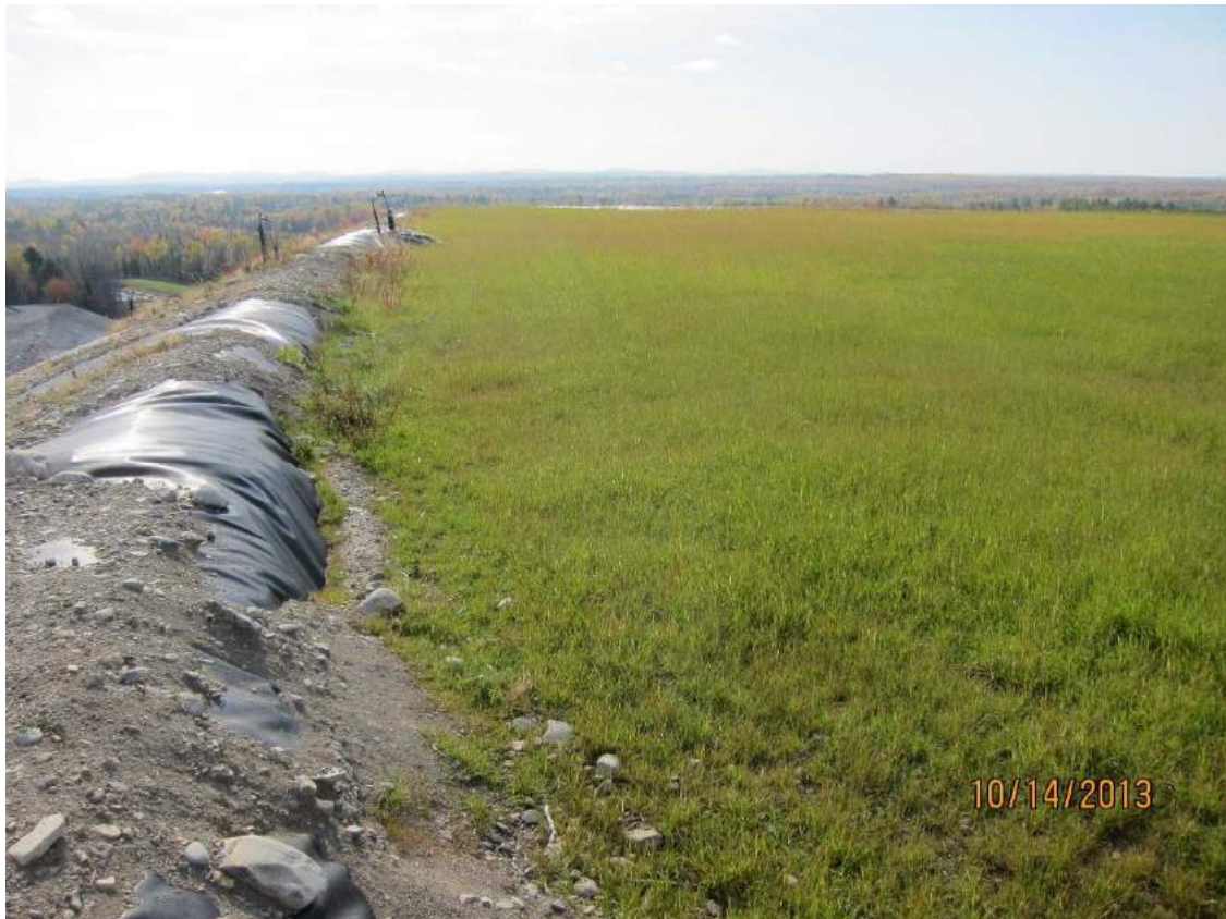
at the crest of eastern interior slope of Cell 5 looking south along the eastern top of Cell 5
