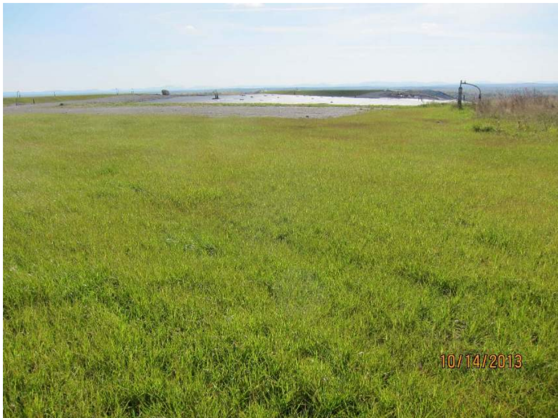
crest of northwestern corner of Cell 1/2 looking over the top of Cell 2
