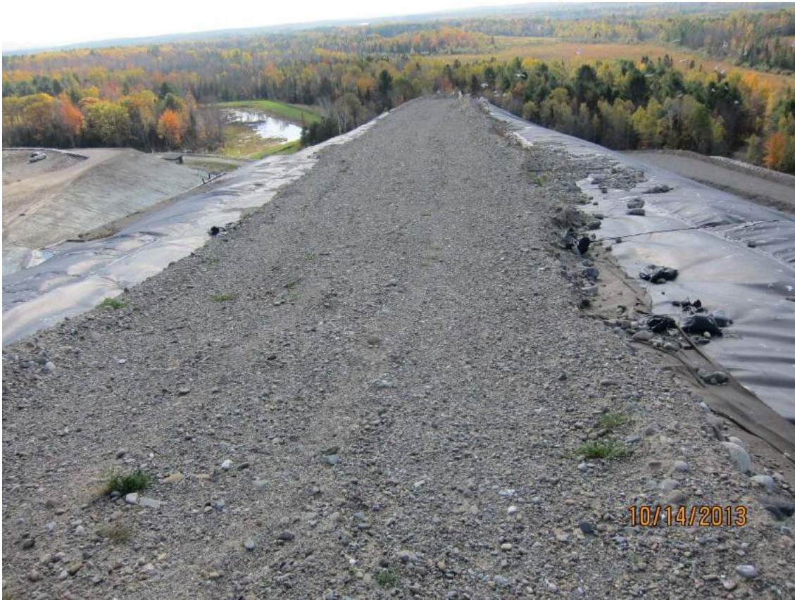
at the crest of eastern interior slope of Cell 5, looking south over the top of Cell 6
