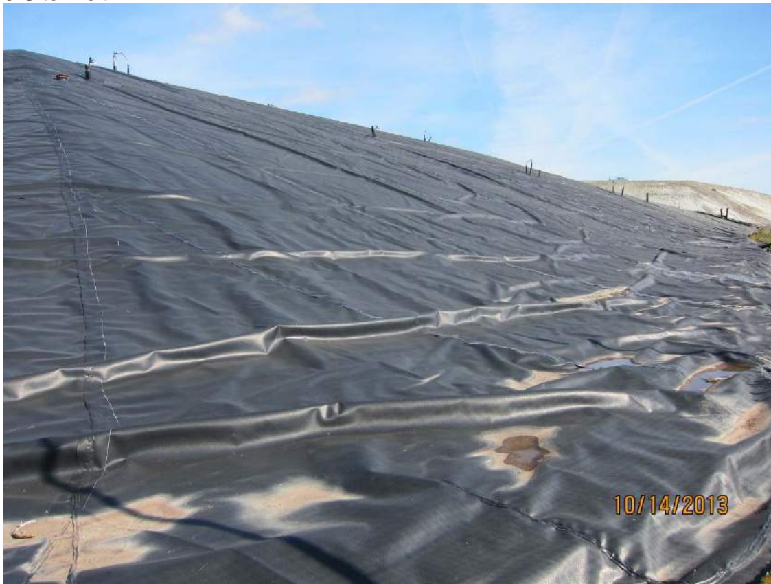
SW corner of Cell 4/6 looking southeasterly along lower slope of Cell 4/6
